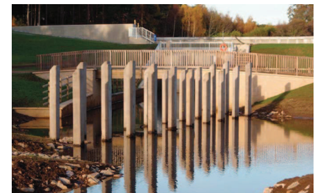
Upstream coarse trash screen
