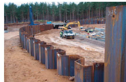
Chapelton Dam sheet pile seepage cut-off
