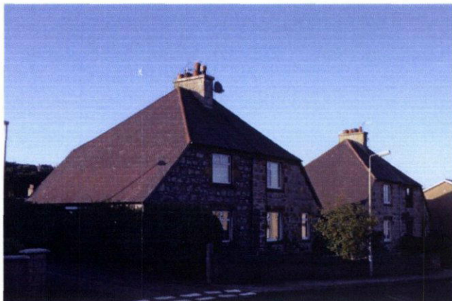
Image 13. House type on Church Street, Seatown, Lossiemouth, bringing roof materials well below the wall lines
