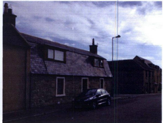
Image 14. House on junction of Commerce Street & High Street, Lossiemouth, introducing roof materials to walls
