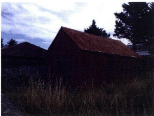
Image 19. Corrugated metal historic fisherman's / salting shed in James Street (West)
