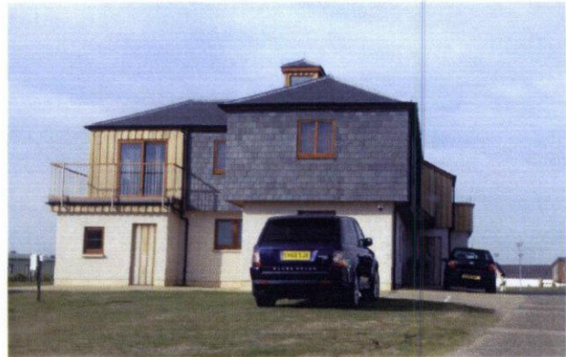
Image 16. Only on close approach to building is it apparent that lower walls are finished in alternative material.
