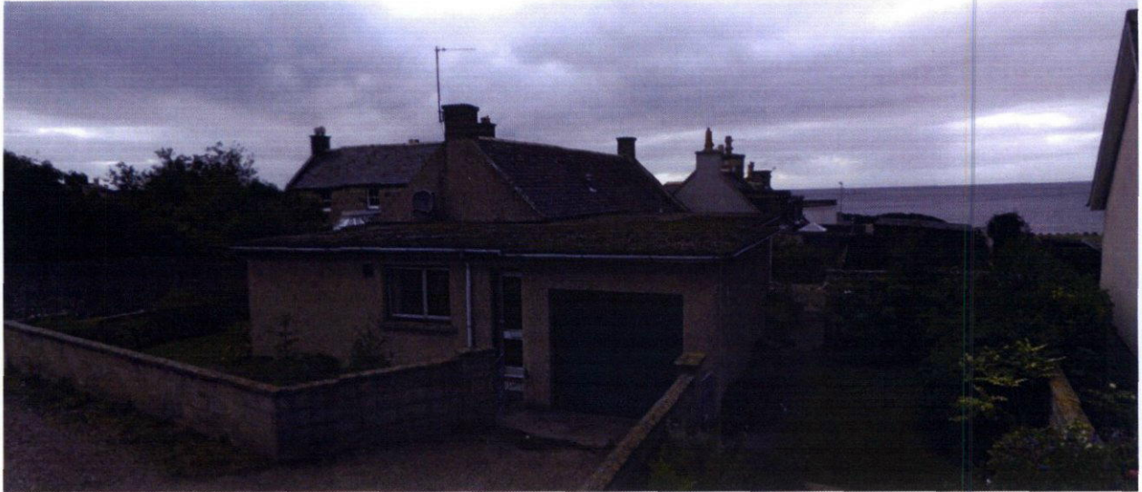
Image 2. The damaged and unsightly flat roof extension wrapping around the South and East of the property
