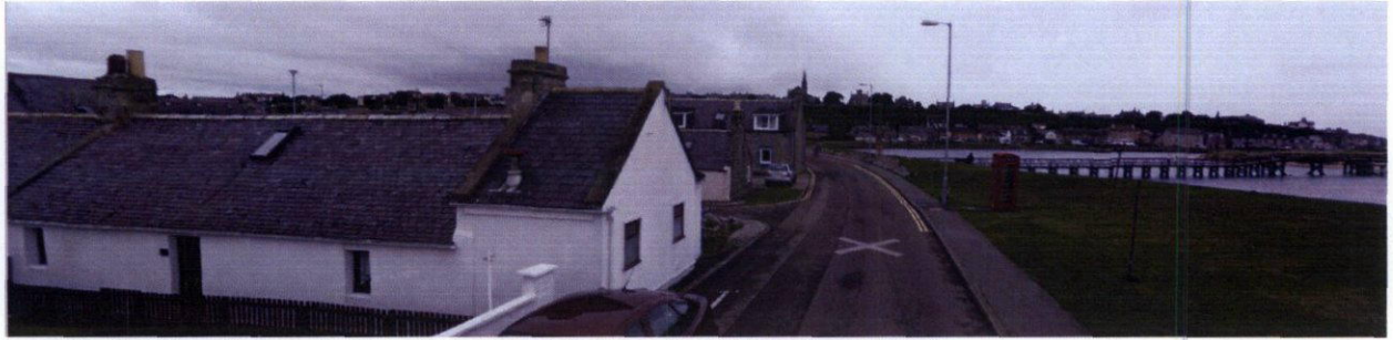
Image 10. Traditional fisherman's cottages in Seatown of Lossiemouth with facing the East Beach
