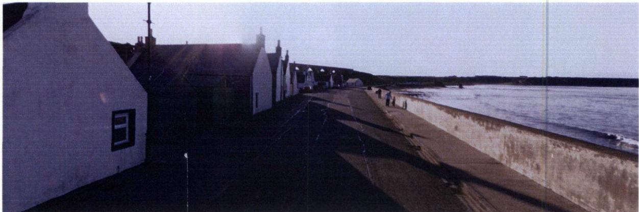
Image 7. Traditional fisherman's cottages in Cullen, turned so gable faces harsh conditions from coast
