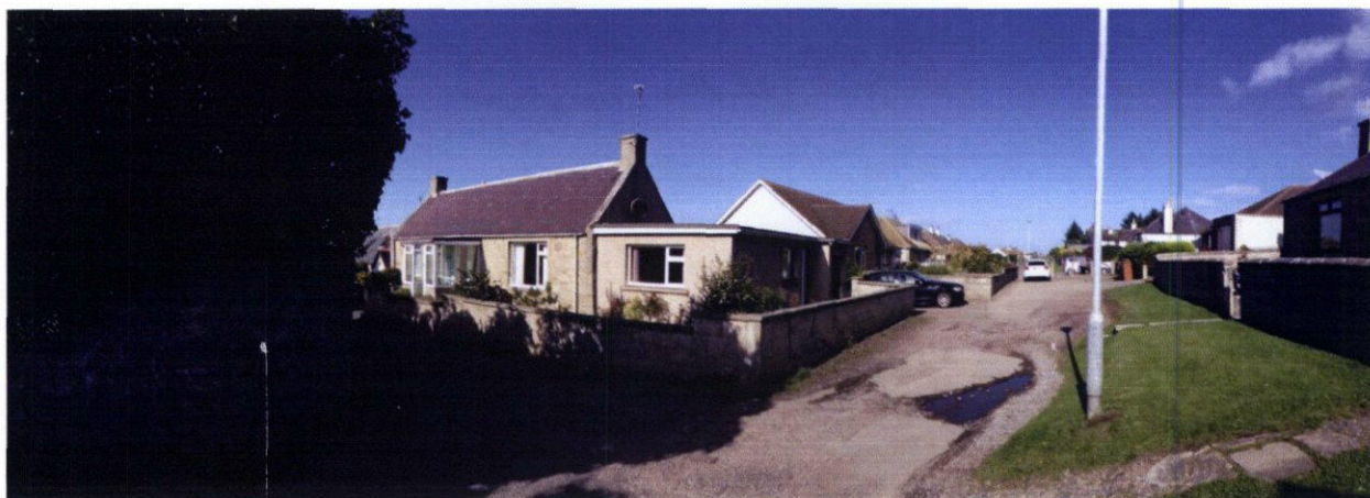
Image 1. Clanchattan, 7 Paradise Lane, Viewed from the South East on James Street, looking North West to the site
