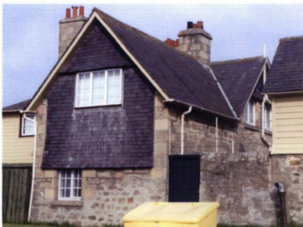
Image 17. West end of Dunbar Street - slate roofing material introduced to vertical walls
