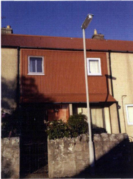
Image 21. Corrugated metal roof & wall clad house type in Church Street / Ogston Lane area
