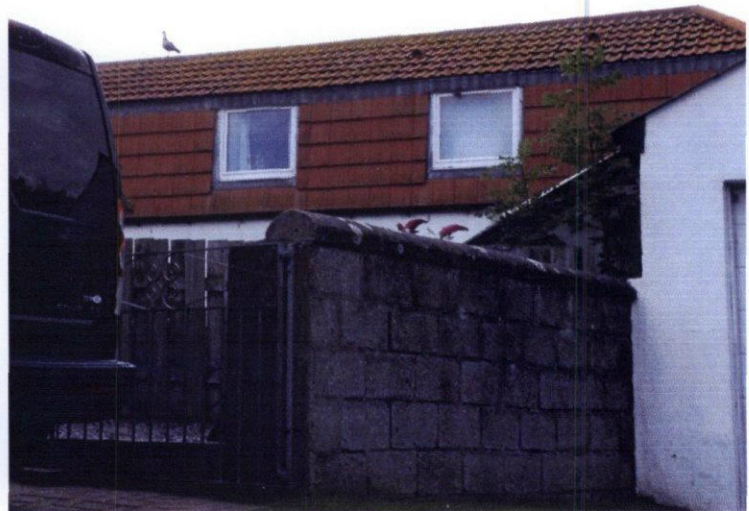
Image 22. Pan-tile roof and upper wall finish to house at far West end of James Street directly adjacent to site
