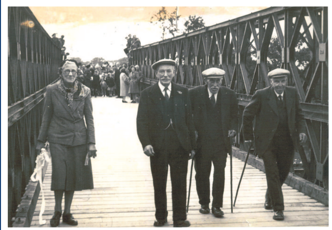
The old bridge was opened by Broom of Moy residents in 1948
