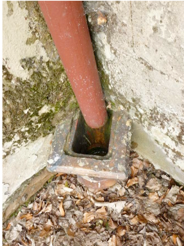
Photograph 010: The gully arrangement to the base of some pipes is unsatisfactory. It varies between pipes disappearing into the ground, to visible open gulleys, some of which are broken.
