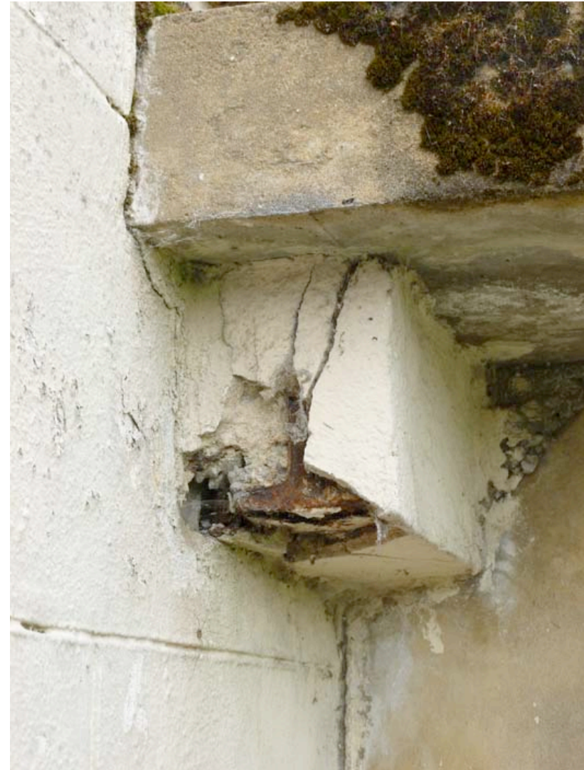
Photograph 024: The I beam supporting the external concrete landing, on the north elevation, is badly corroded.
