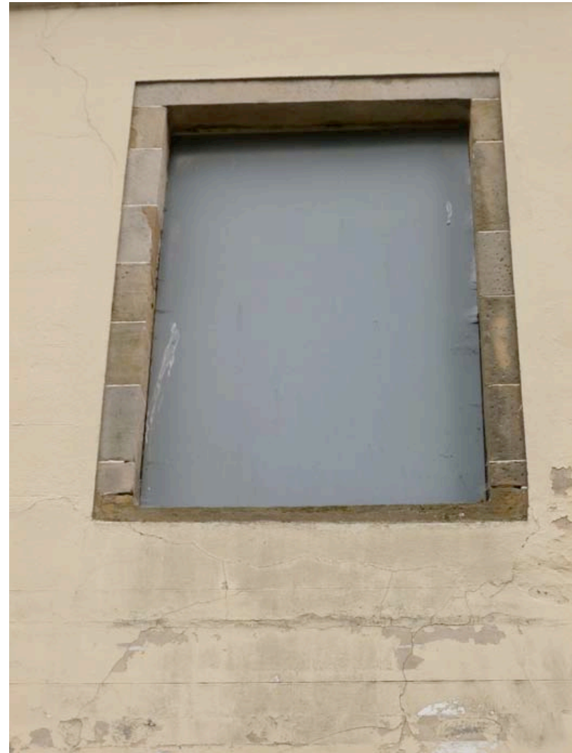
Photograph 028: There are several cracked cills around the building. This is especially apparent on the west elevation as shown in the photograph above.
