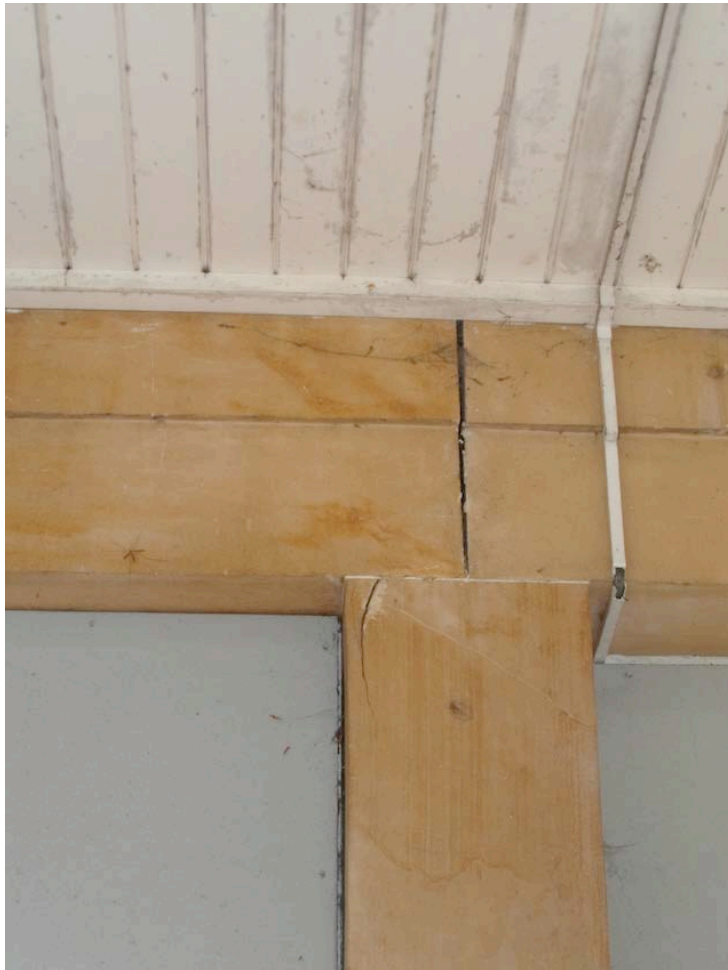
Photograph 019: The joint between the high level lintel on the porch structure has opened up which is a result of the movement in the two corner columns.
