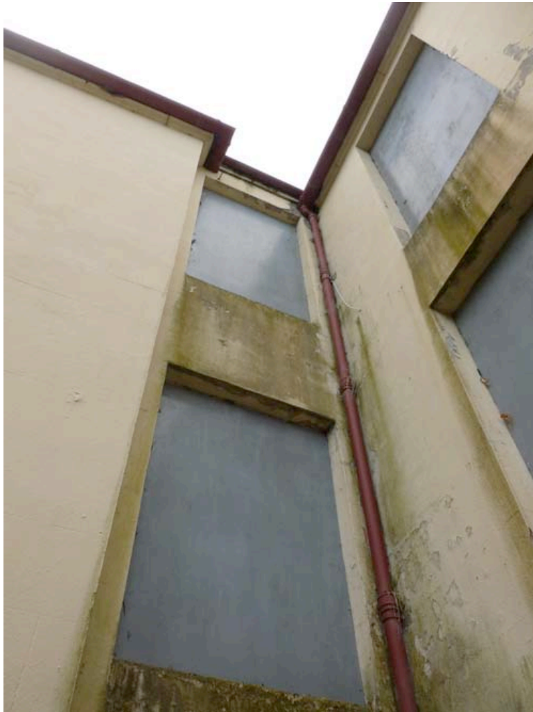
Photograph 009: The existing downpipes have been painted in red oxide. The downpipe, shown above, has been blocked by vegetation, which has in turn caused a build up of water in this location.
