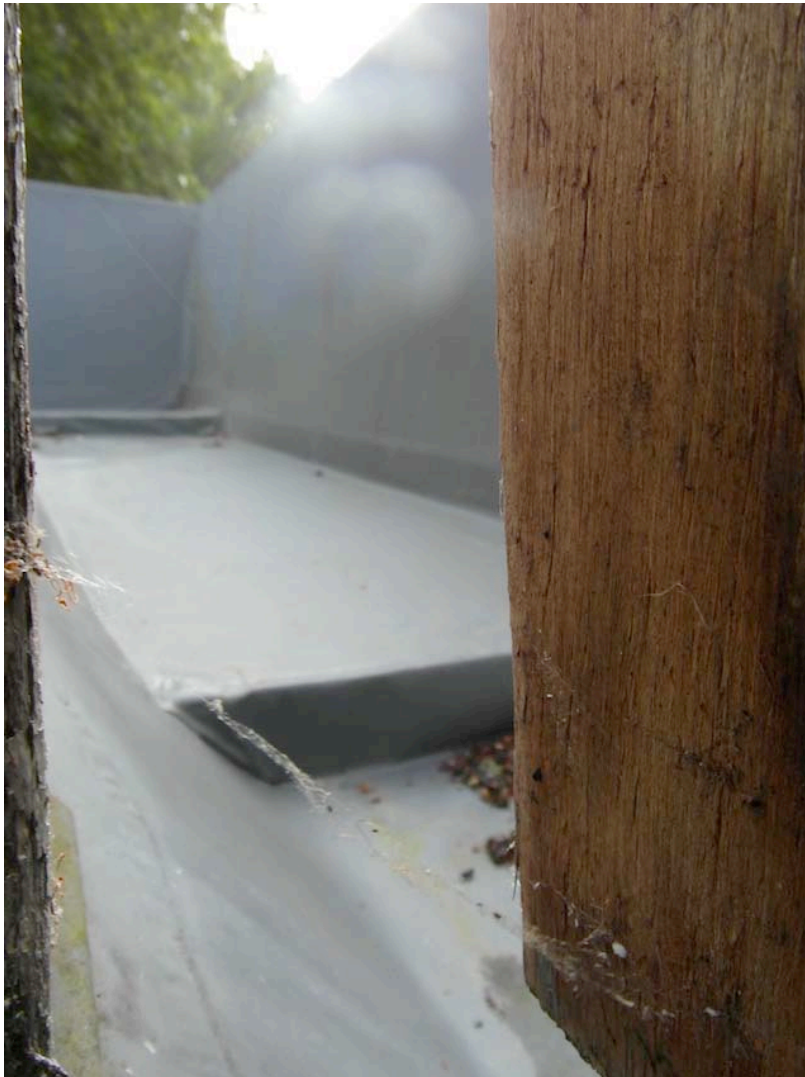
Photograph 007: The perimeter parapet gutter has been clad in sarnafil.
