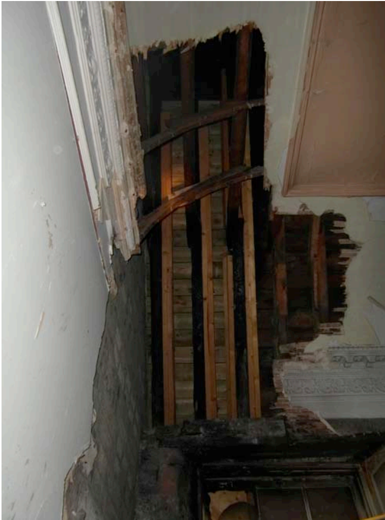
Photograph 035: The ceiling has been damaged in xF.06 on the south wall by a previous outbreak of fire.
