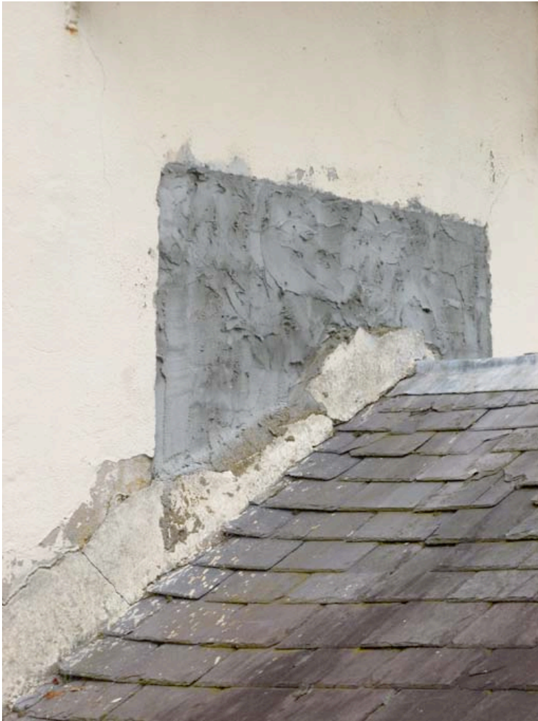
Photograph 041: Single storey ancillary building. There are a number of chipped and missing slates.
