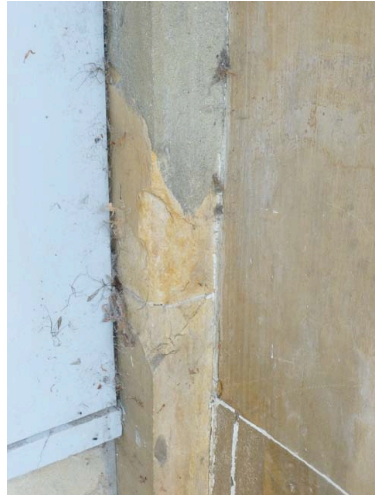
Photograph 016: The rebats for some of the windows and doors have been left exposed. Cement repairs have been made in an attempt to repair the delamination.
