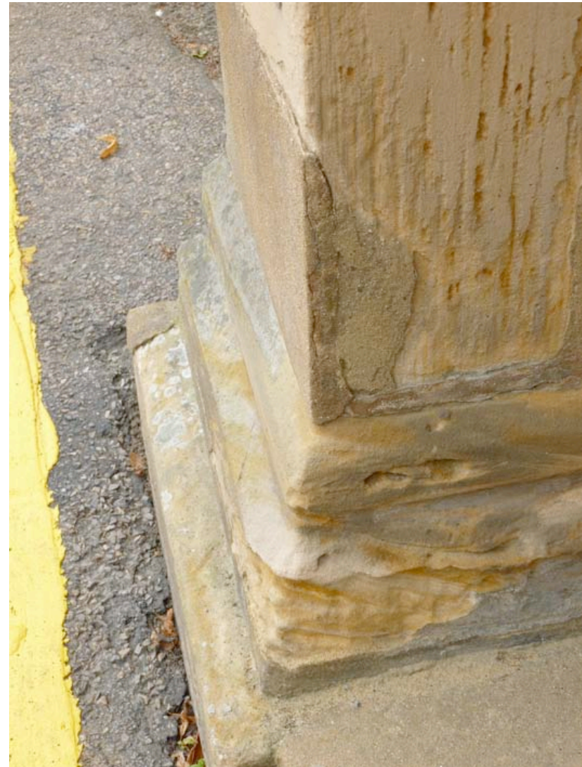
Photograph 022: Plastic repairs have been applied to the base of the column to counteract the delamination.
