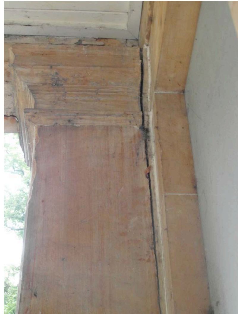
Photograph 018: Noticeable movement has occurred between the portico and the main front wall of the building.
