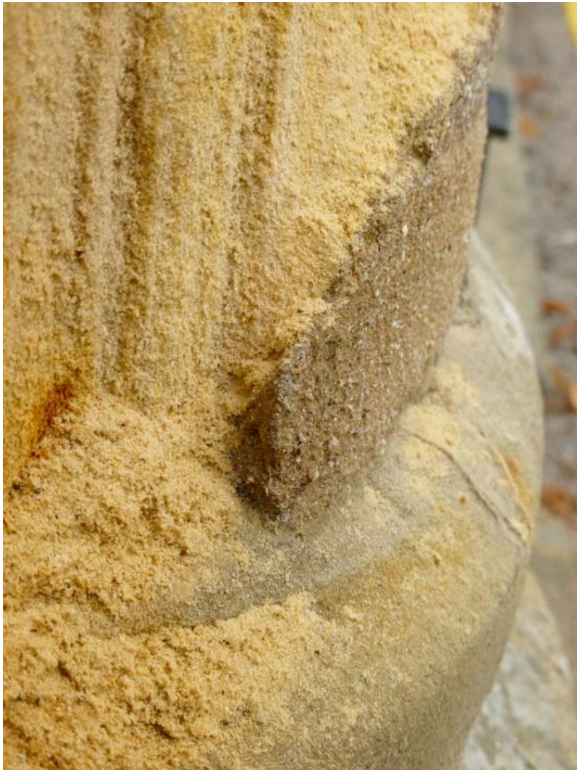
Photograph 021: The delamination of the stonework is considerable at the base of the pilasters.
