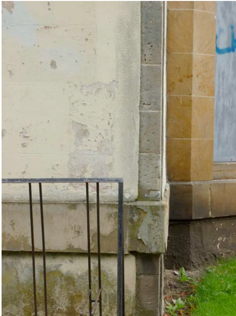
Photograph 015: The corner quoin stones have been left exposed and they have been dressed (stugged finish). The tooling may indicate an intention at some stage to carry the render over the margin stones. Some cement repairs have been made to the quoin stones.
