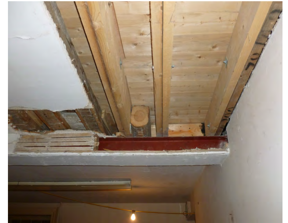
Past structural repairs to underside of ground floor
