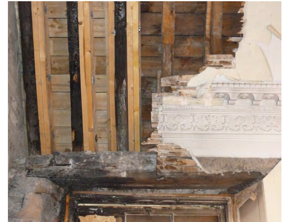
Past structural repairs to roof
