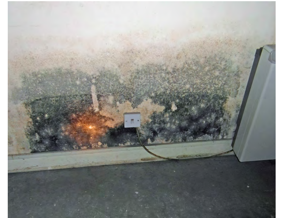
Damp penetration at lower ground level
