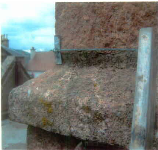
Photo 55 – String Course at First Floor Level
