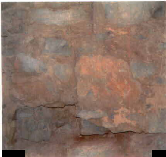
Photo 23 – North Wall, Second Floor
