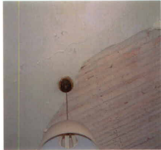
Photo 34 – First Floor Light Fitting
