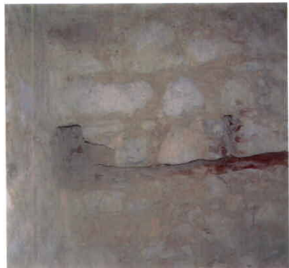
Photo 24 – Second Floor West Wall – Joist Pockets
