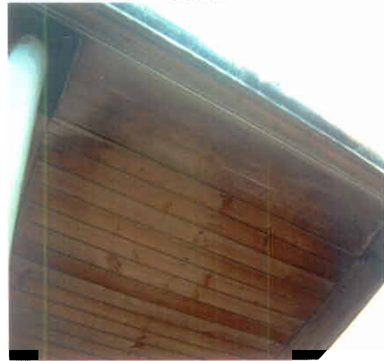
Photo 10 – Underside of Canopy above Bell
