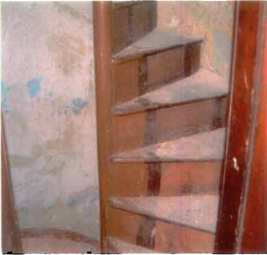
Photo 25 – Second Floor Spiral Staircase
