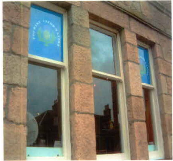
Photo 50 – North Facing Window to Ground Floor
