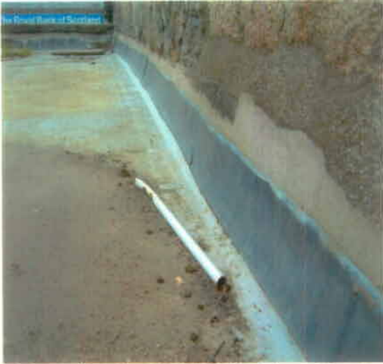
Photo 43 – Roof / Wall Flashing – North Elevation
