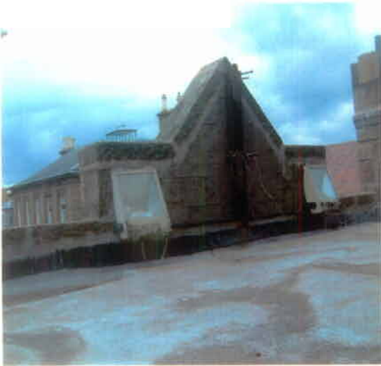
Photo 45 – North Facing Parapet Wall to Single Storey Roof
