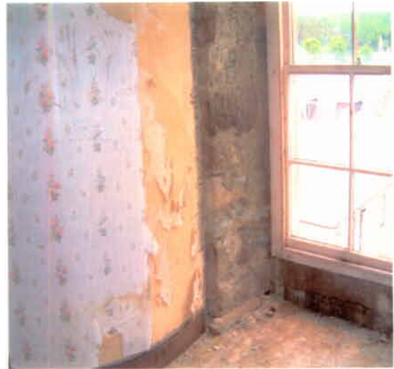
Photo 20 – Window to Third Floor
