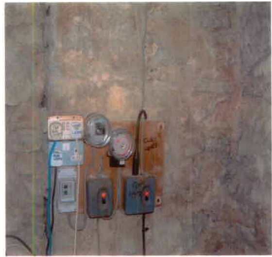
Photo 26 – Electrics to First Floor
