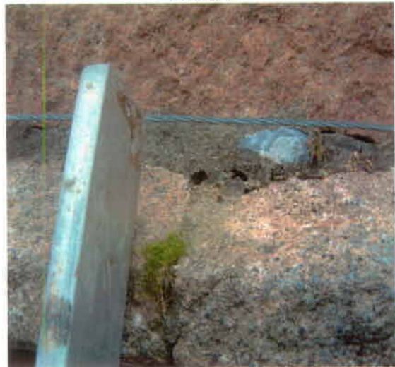
Photo 54 – Pointing at Single Storey West Wall
