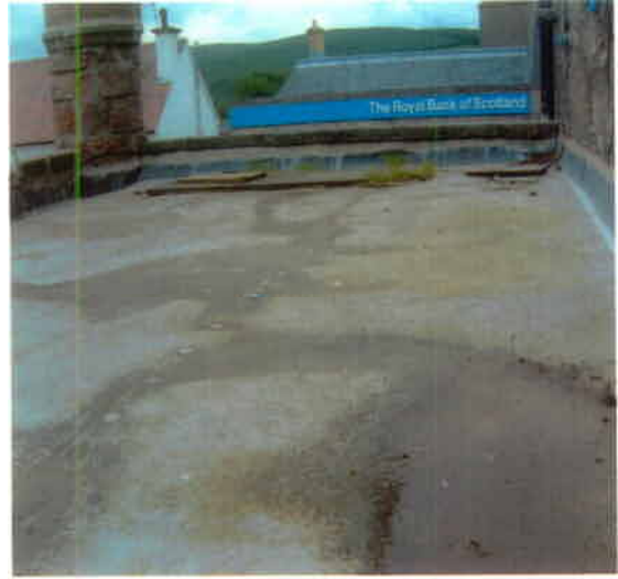
Photo 44 – Flat Roof – North Side
