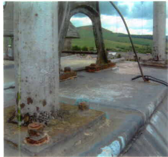
Photo 4 – Flat Lead Roof Beneath Bell
