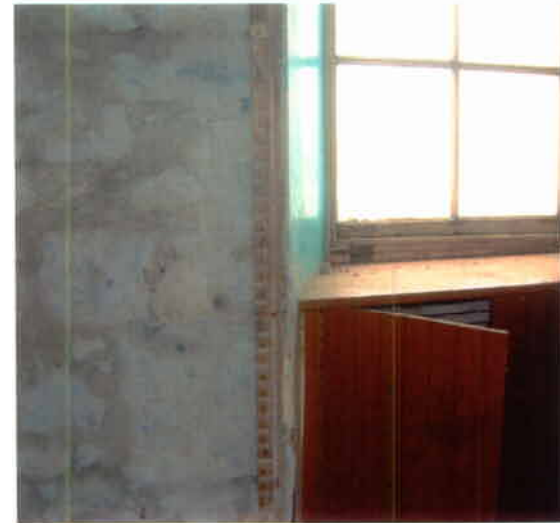
Photo 30 – First Floor – East Wall
