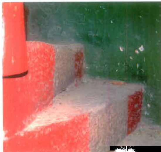
Photo 35 – Concrete Steps upto First Floor
