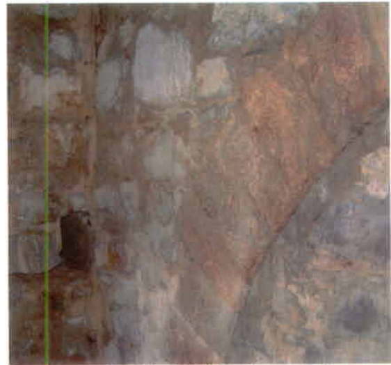
Photo 22 – North Wall, Second Floor
