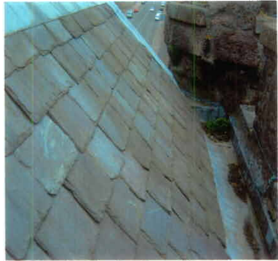
Photo 8 – East Section of Slate Roof to Tower
