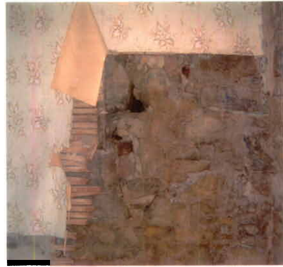
Photo 28 – First Floor South Wall
