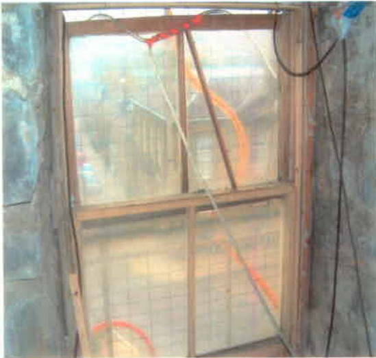
Photo 21 – Window to North Wall – 2 nd Floor
