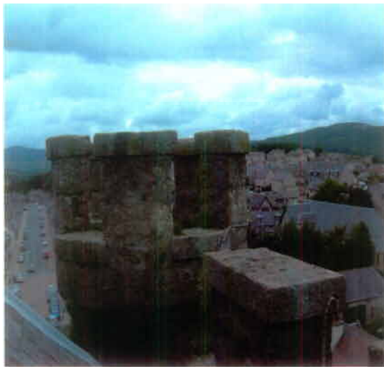
Photo 3 – North East Turret
