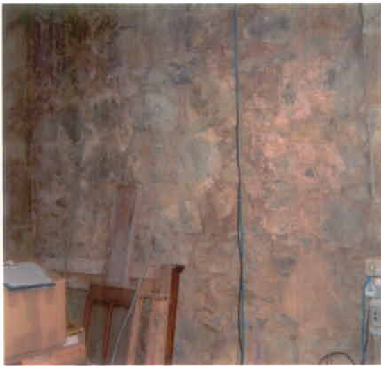
Photo 27 – First Floor – North Wall
