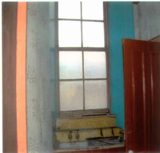
Photo 29 – First Floor – Window
