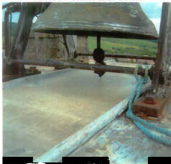
Photo 5 – Flat Lead Roof Beneath Bell
