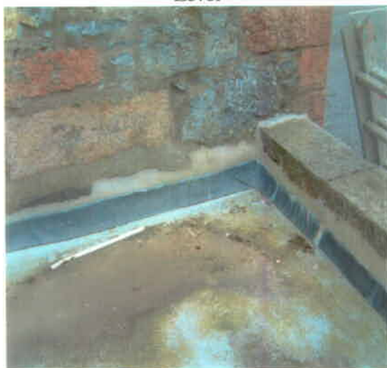
Photo 57 – Lead Flashings to Single Storey Roof
