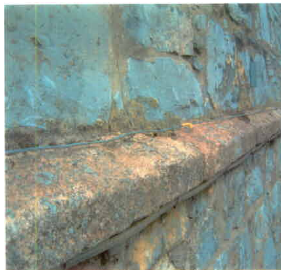
Photo 56 – String Course at First Floor Level West Elevation
