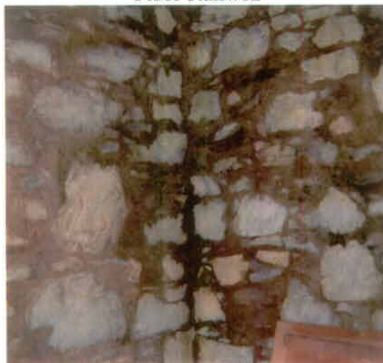
Photo 17 –SE Corner – Third Floor
