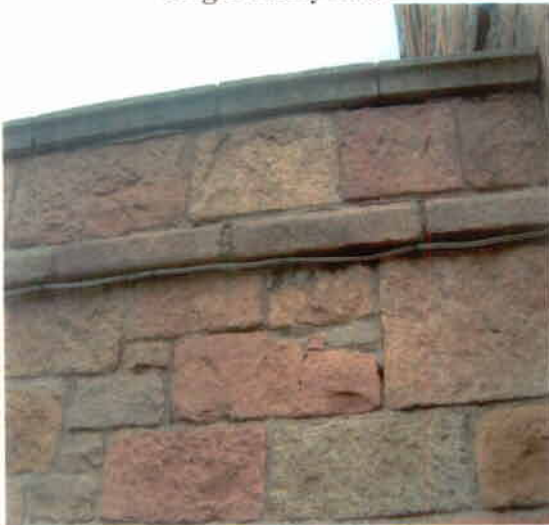
Photo 47 – West Facing Wall
