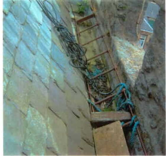
Photo 2 – East Roof Gutter
