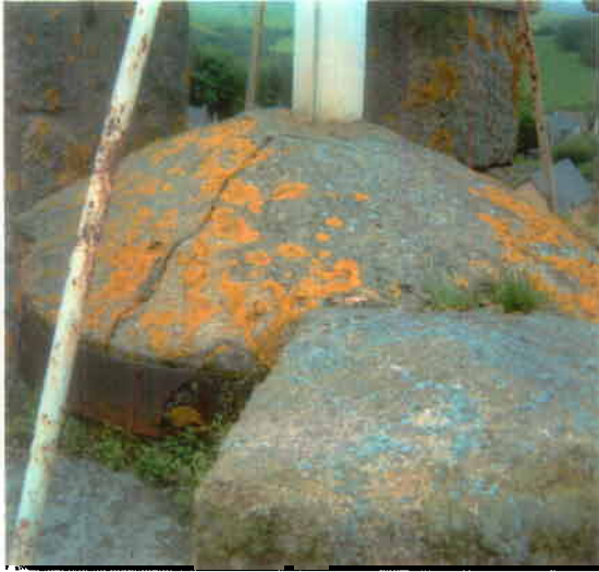
Photo 1 – SE Corner Flagpole Base
