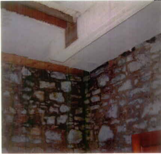
Photo 19 – Third Floor Ceiling
