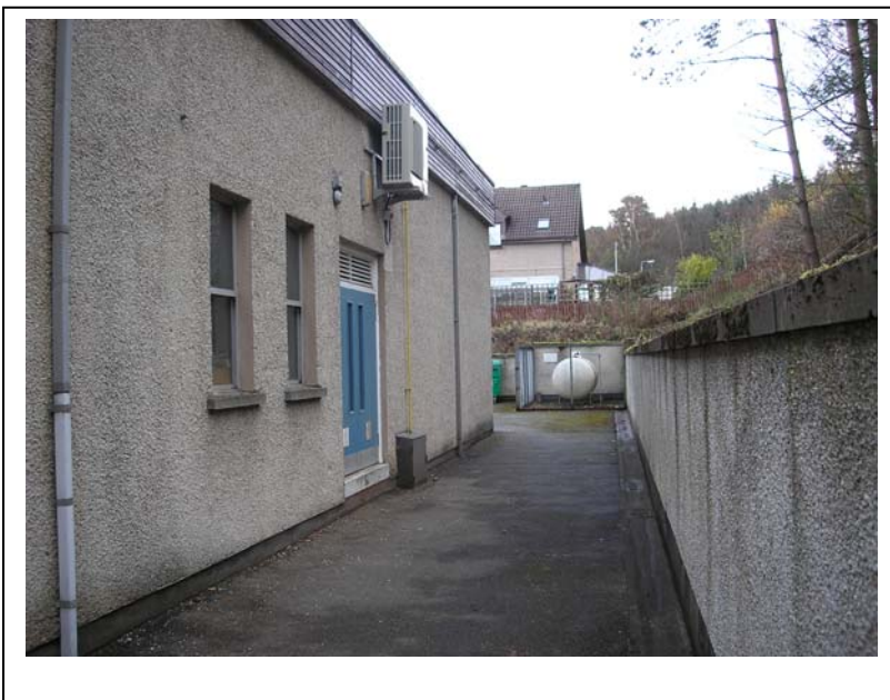
Additional photographs (Left) Rear alleyway showing door to existing boiler house and LPG tank. (Below) Side access showing two oil delivery vehicles and LPG tank
