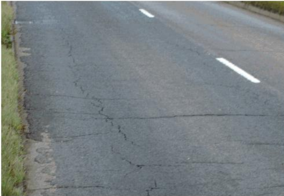
Figure 10 Road showing wheel track and transverse cracking 7
