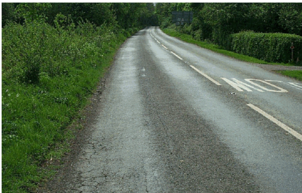
Figure 9 Unevenness of texture across the carriageway
