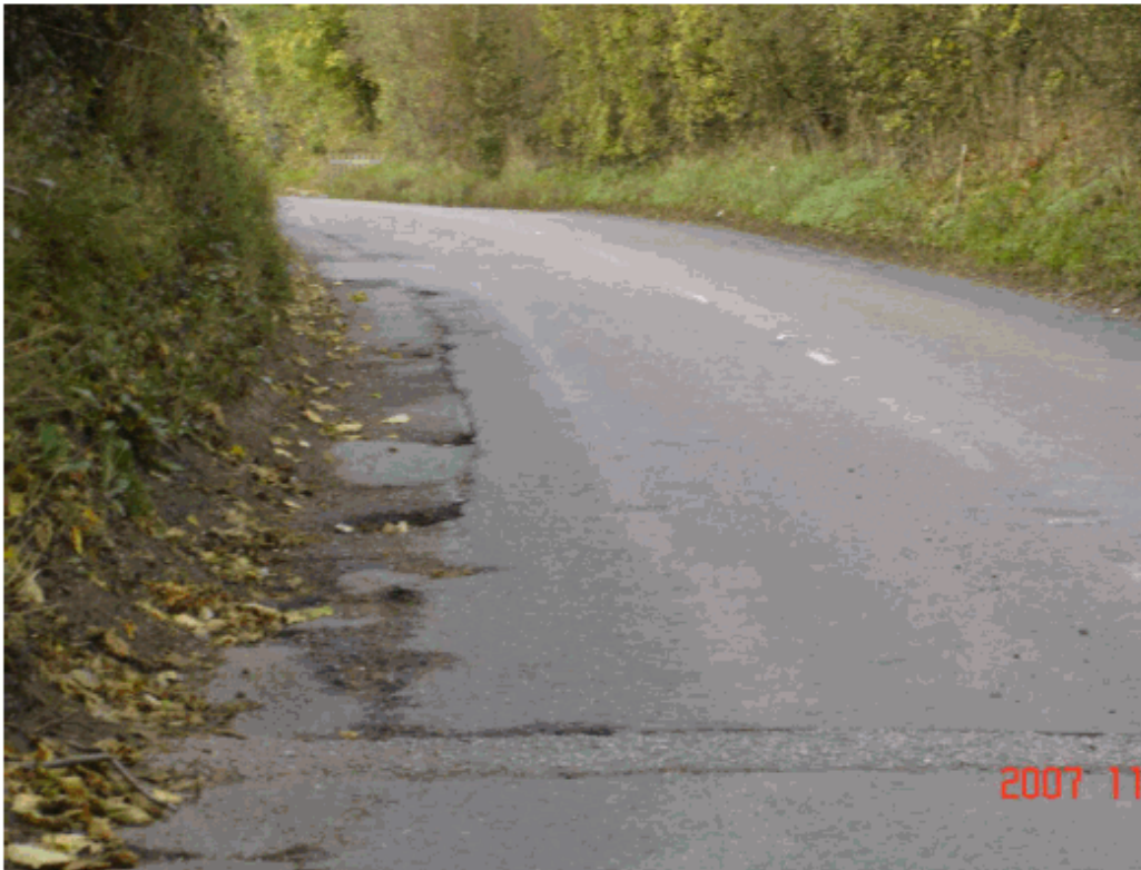
Figure 8 Road where edge of carriageway deterioration has been identified
