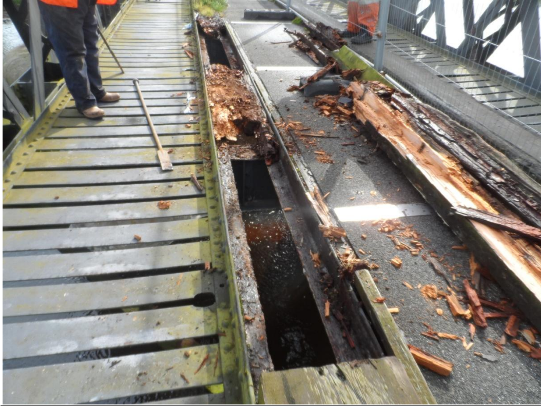
Remains of a rotten timber baulk
