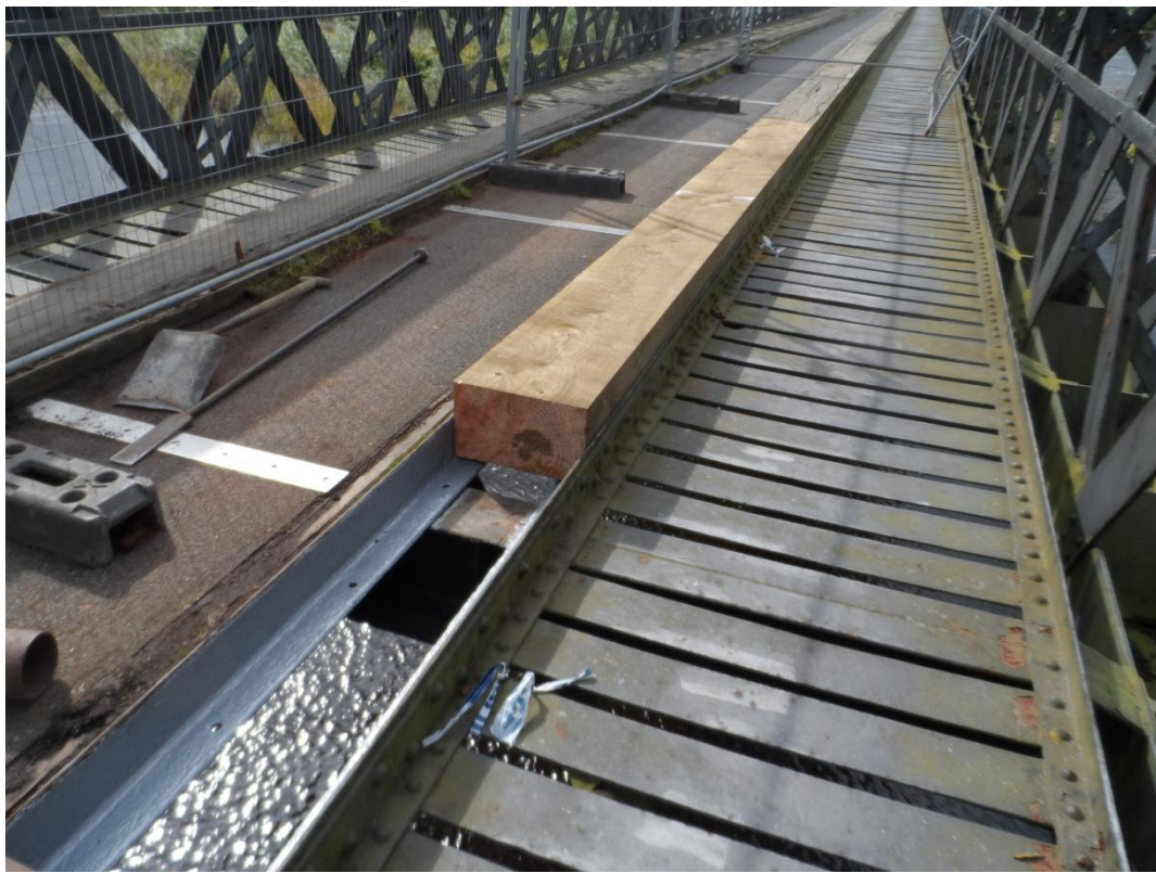
Replacement timber in place
