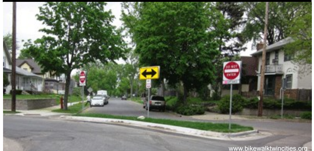
RiverLake Greenway (40th Street), Minneapolis, Minnesota. This diverter forces drivers to turn. Drivers may still access a nearby school, but the route is less direct and more circuitous. This device did not require any change to storm water structures as it left existing drainage basins intact.
