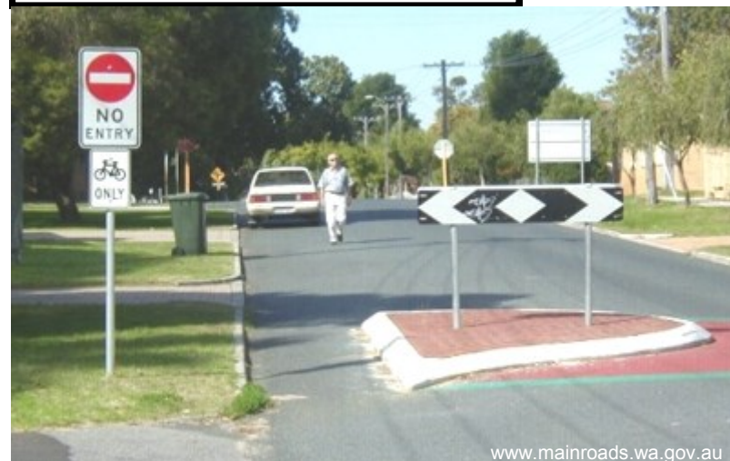
Half closure with cycle access, Western Australia. Cars may pass by this feature in one direction, but must turn in the other. It does not affect drainage structures.
