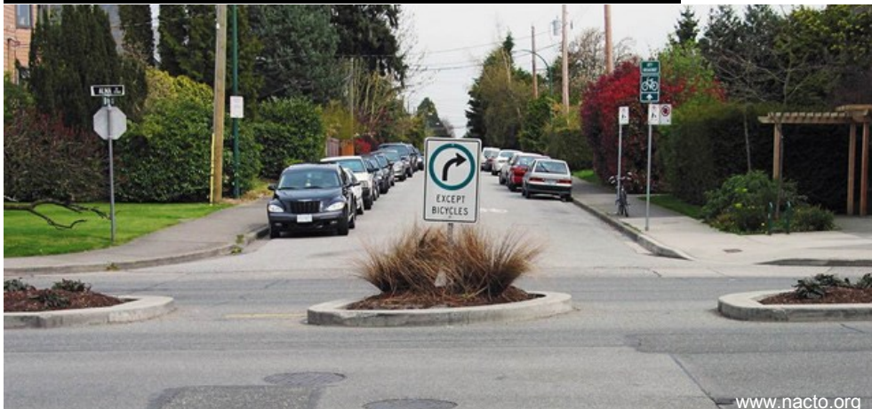
Median diverters force turns for motorised traffic, but offer permeability for cycles and pedestrians. They have the added benefit of providing a refuge space to cross busy roads.
