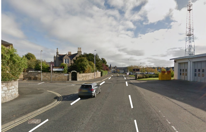
Station Road centre line removed and advisory cycle lanes added
