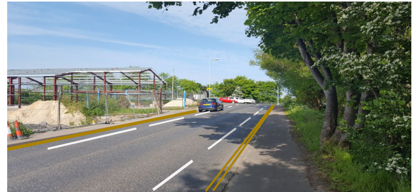
Linkwood Road, advisory cycle lanes added, parking prohibited. Very limited centre line removal required.
