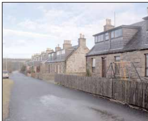
View north along Dailuaine Terrace showing the line of one-and-a-half storey, traditional stone houses with modern replacement windows and attic box dormers
