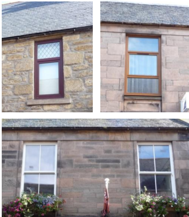
Modern replacement windows (top) and traditional timber sashes (bottom)
