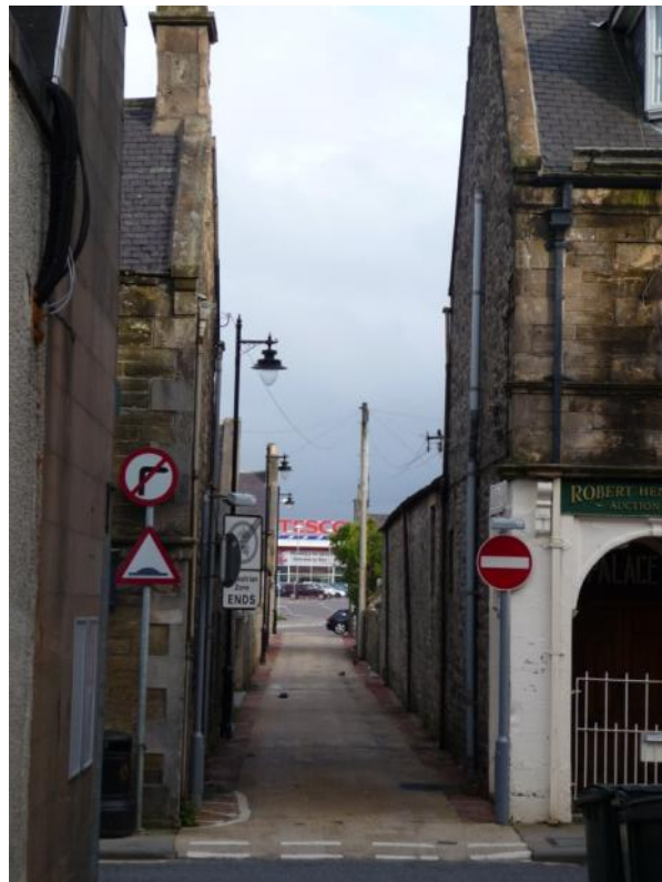
The impact of new development on views in and out of the conservation area is significant
