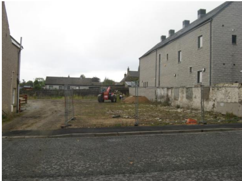
Gap sites on Mid Street (top) and Chapel Street (bottom) detract from the historic environment.
