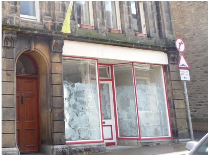
Vacant commercial premises detract from the character of Mid Street
