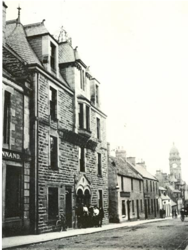
The Commercial Hotel, Mid Street, c.1900, Moray Local Heritage Centre
