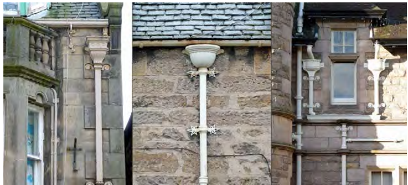
Late nineteenth century decorative cast iron rainwater goods
