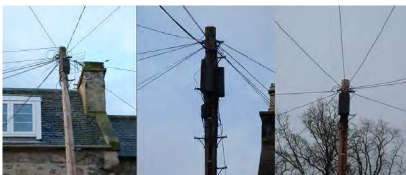
Overhead wires and poles disfigure parts of the conservation area
