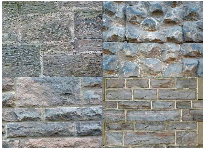
Examples of ashlar stonework of varying styles and materials found in the conservation area
