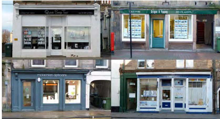
Traditional shopfronts on Forres High Street, displaying good examples of signage which is contained within the original fascia
