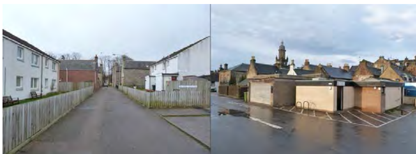
Poor boundary treatments: to social housing on Urquhart Street, and exposed in the backlands from the introduction of the car park at Leys Road
