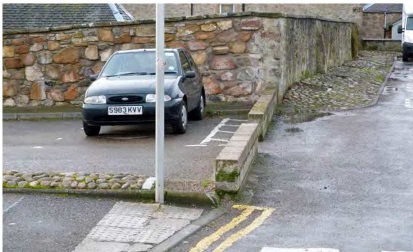
Degraded public realm at car parks
