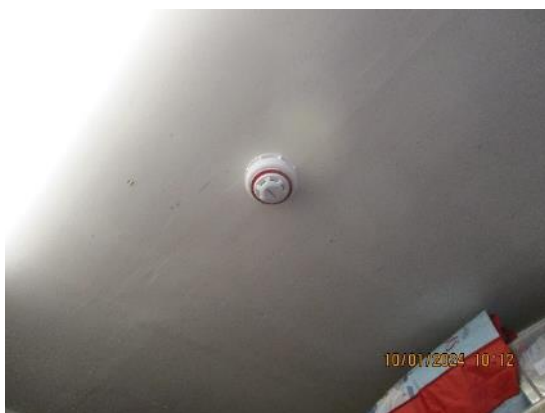
183. Smoke detection head. Typical.
