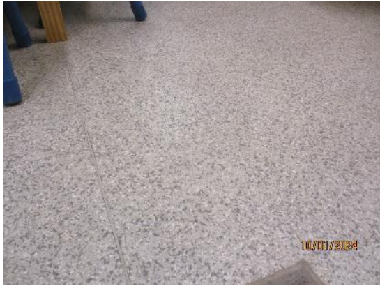
73. Sheet vinyl in satisfactory condition
