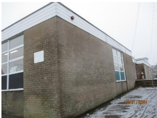
23. Brick external structure
