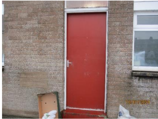
38. Timber service doors
