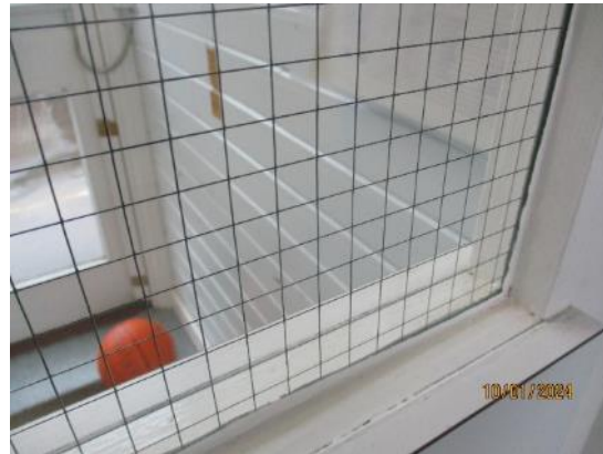
40. Georgian wired glass to external doors
