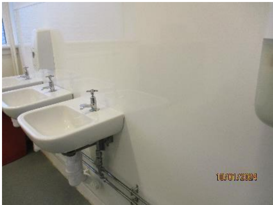
102. Wetwall, half height in pupil toilets
