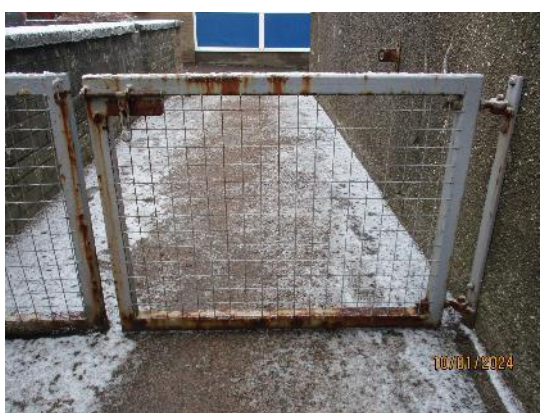
214. Metal frame and mesh gate
