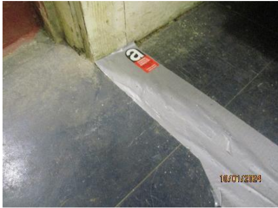
79. Tape repair to vinyl tiles
