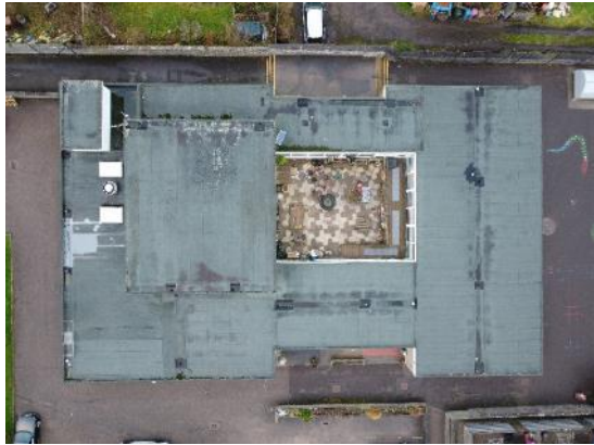
1. Aerial photo of roofs
