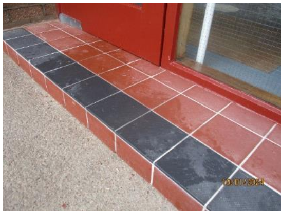
63. Quarry tile steps
