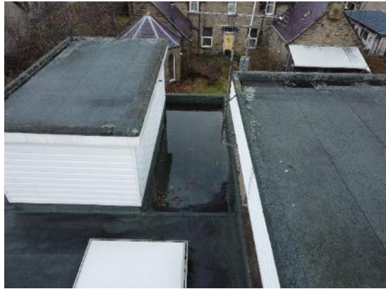
2. Tank House roof (left)
