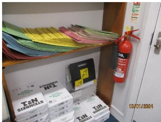
196. Induction hearing loop system.reception office 1/7
