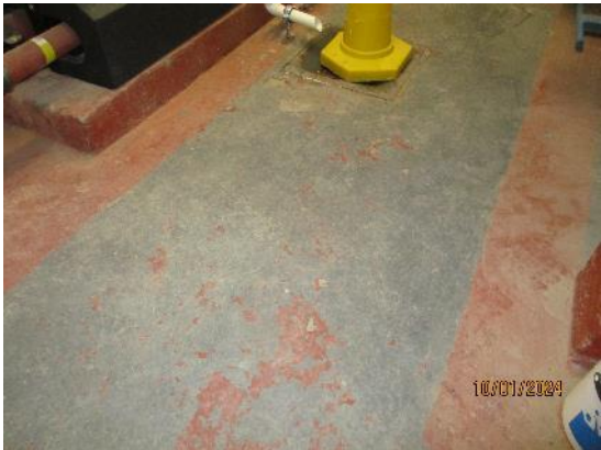
81. Painted concrete floor in Boiler Room
