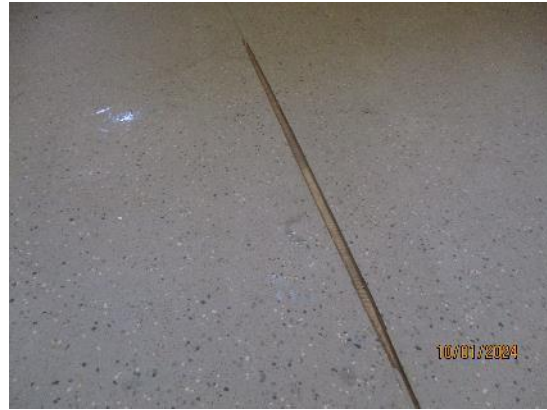
74. Sheet vinyl with open joints
