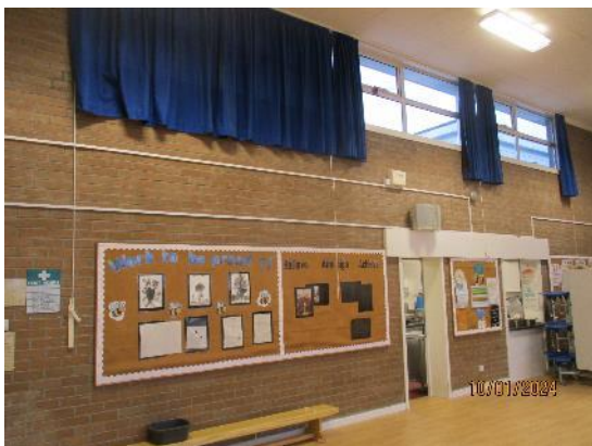
88. Facing brick walls
