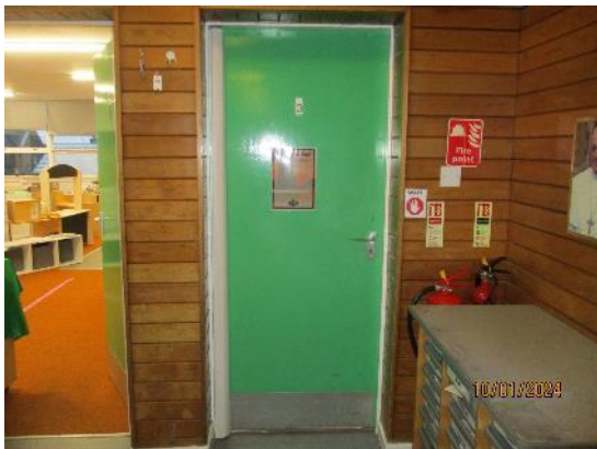
104. Timber hollow core classroom doors
