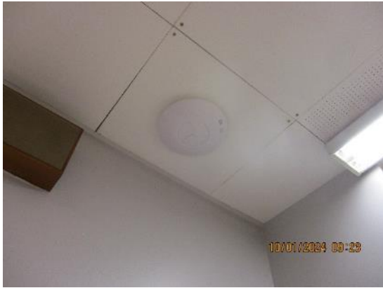
161. Extract fan – nursery kitchenette 1/15
