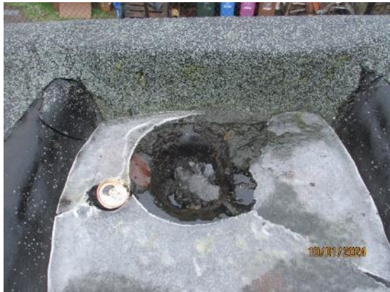
21. Blocked downpipes
