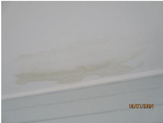
138. Watermarked plasterboard ceilings
