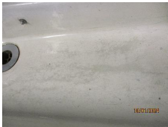
136. Surface wear and erosion
