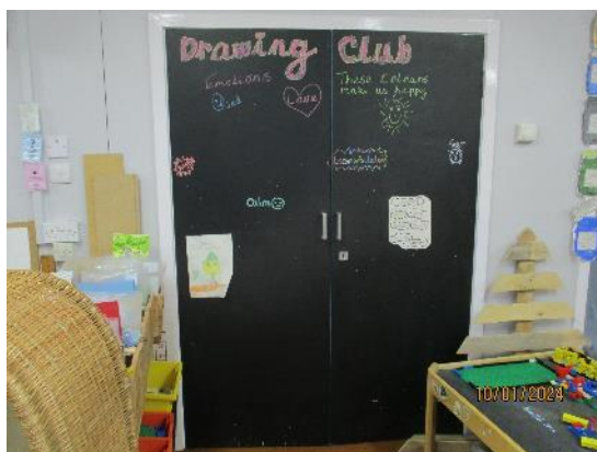
106. Timber hollow core double doors
