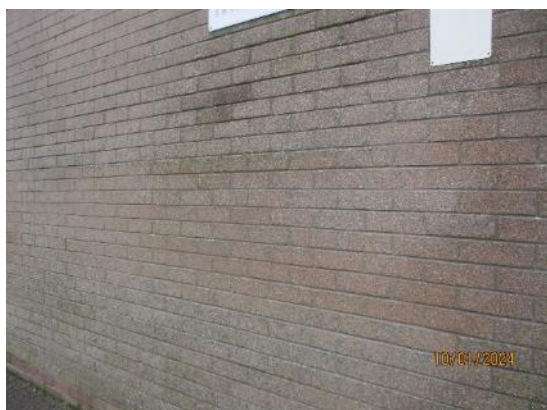
31. Facing brick external finish
