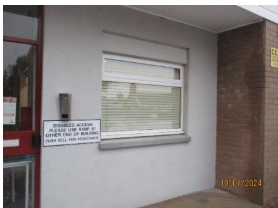
33. Textured paint finish to rendered walls
