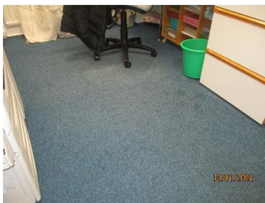
70. Carpet in satisfactory condition
