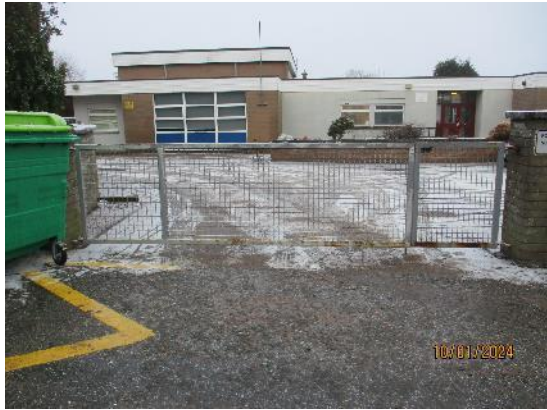
215. Metal frame and mesh vehicle access
