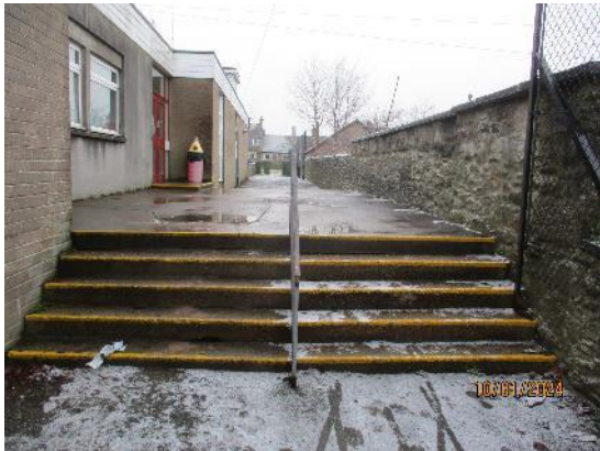
205. Concrete steps to rear
