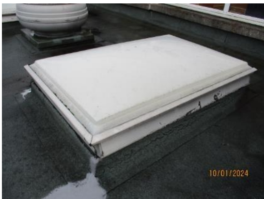
11. GRP rooflights above the Kitchen
