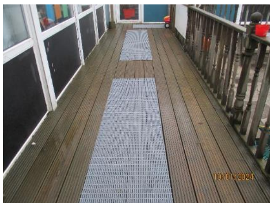
67. Raised timber decking
