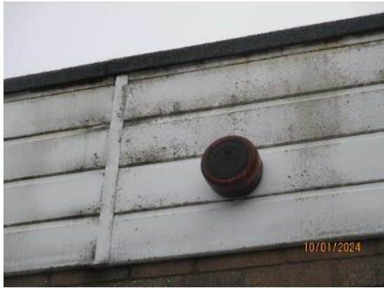
13. UPVC fascias to main building
