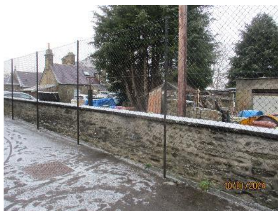
212. Chain link fencing
