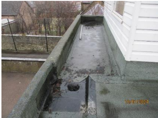
15. Felt box gutters and outlets
