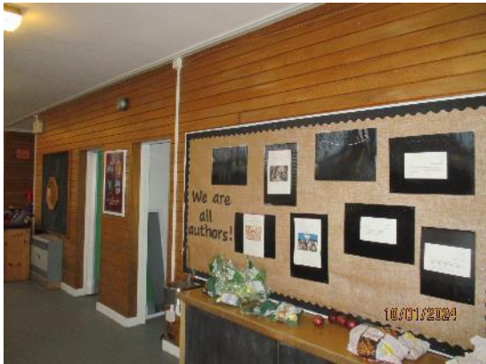
98. Timber linings – pupil corridor
