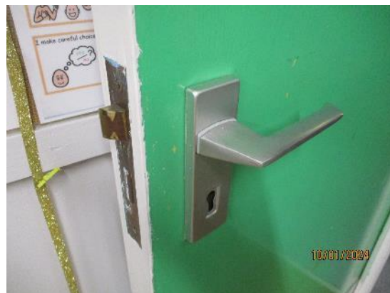
113. Aluminium lever handles to internal doors
