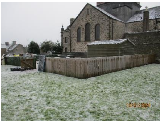
59. Bare timber fencing
