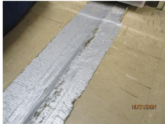
76. Tape repair to vinyl tiles
