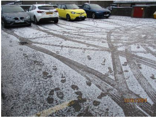
197. Tarmacadam access and car park
