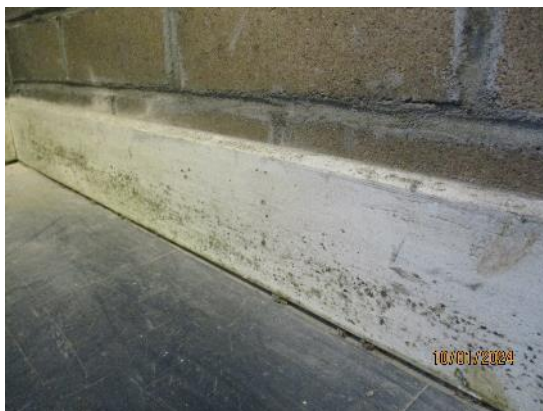
141. Mould marked skirting boards
