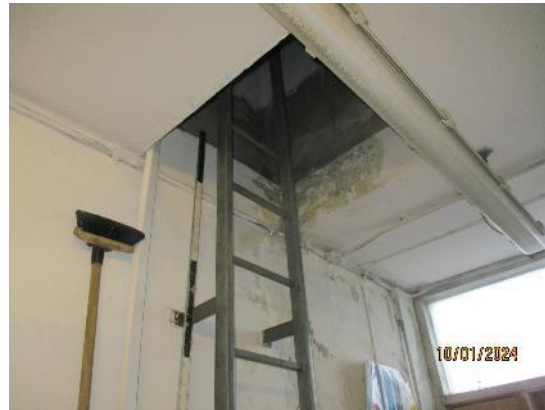
82. Steel ladder to Tank House
