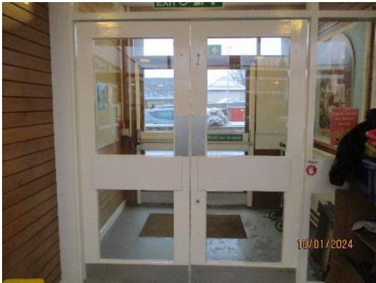
110. Timber double doors
