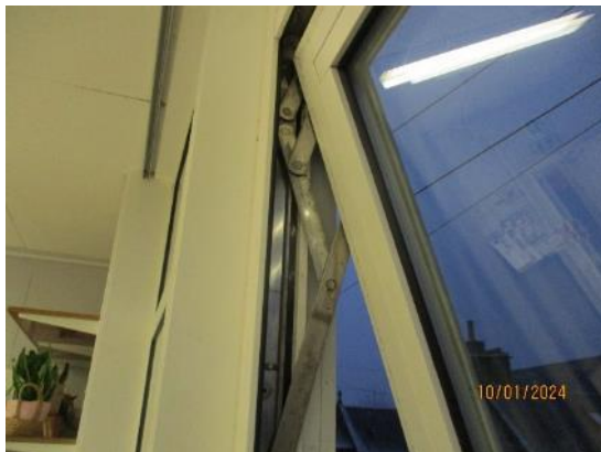
51. Typical hinge mechanism
