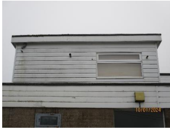
14. UPVC cladding to Tank House
