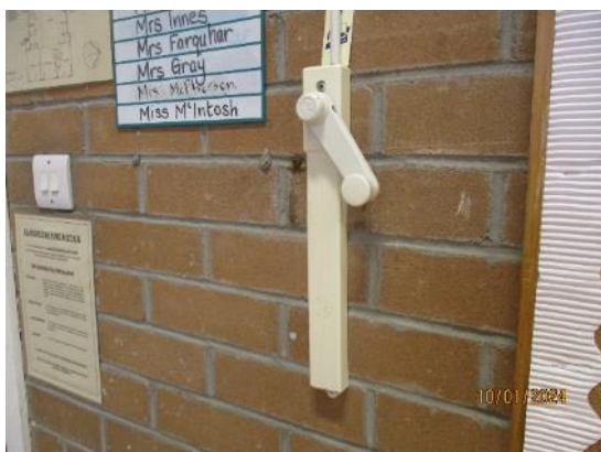
54. Winding handle mechanism
