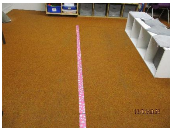
71. Repairs to damaged carpet
