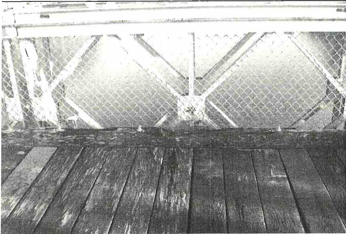
Showing condition of the ribands and the timber chesses
