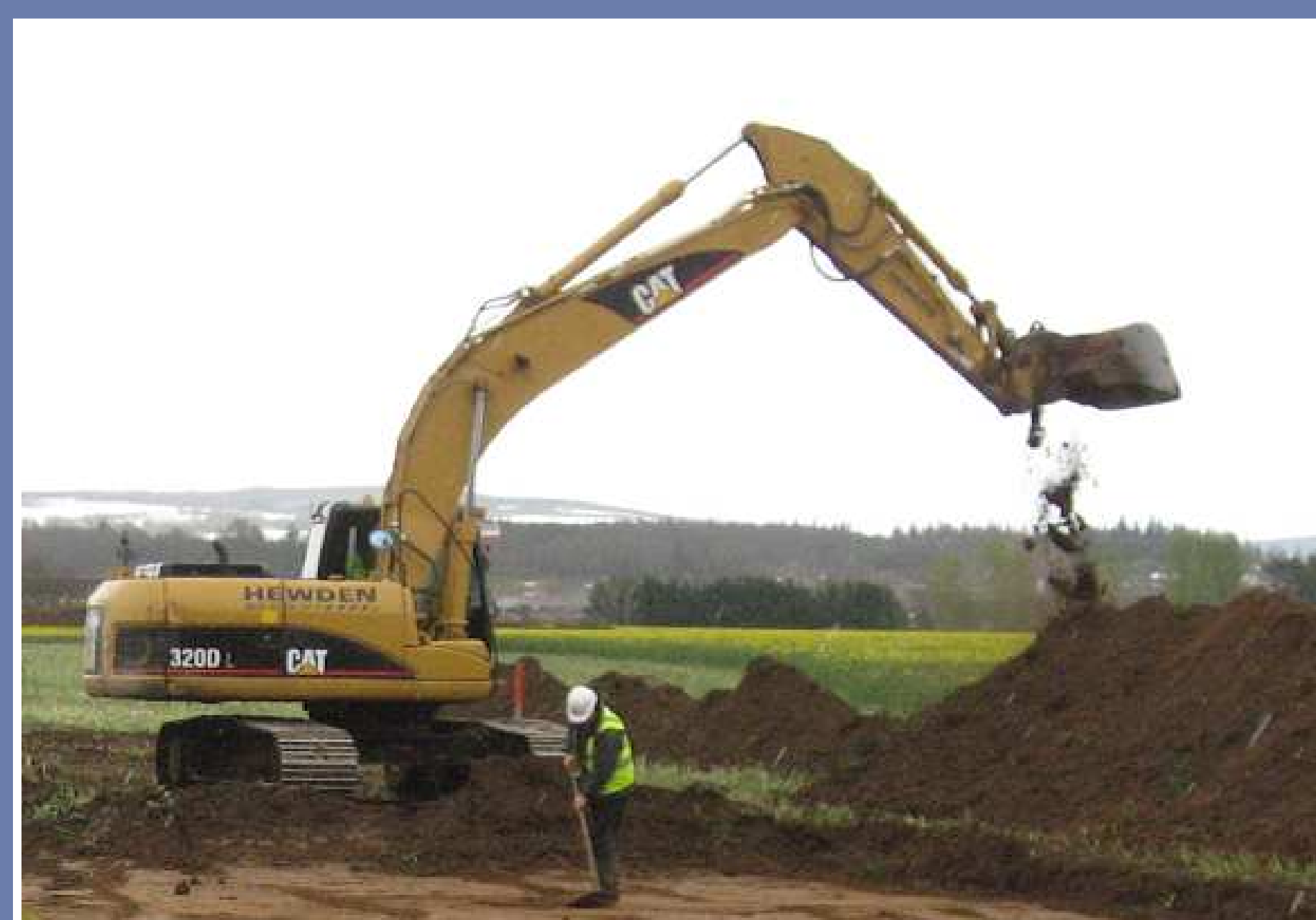
Top soil removal at the site of the A96 temporary diversion
