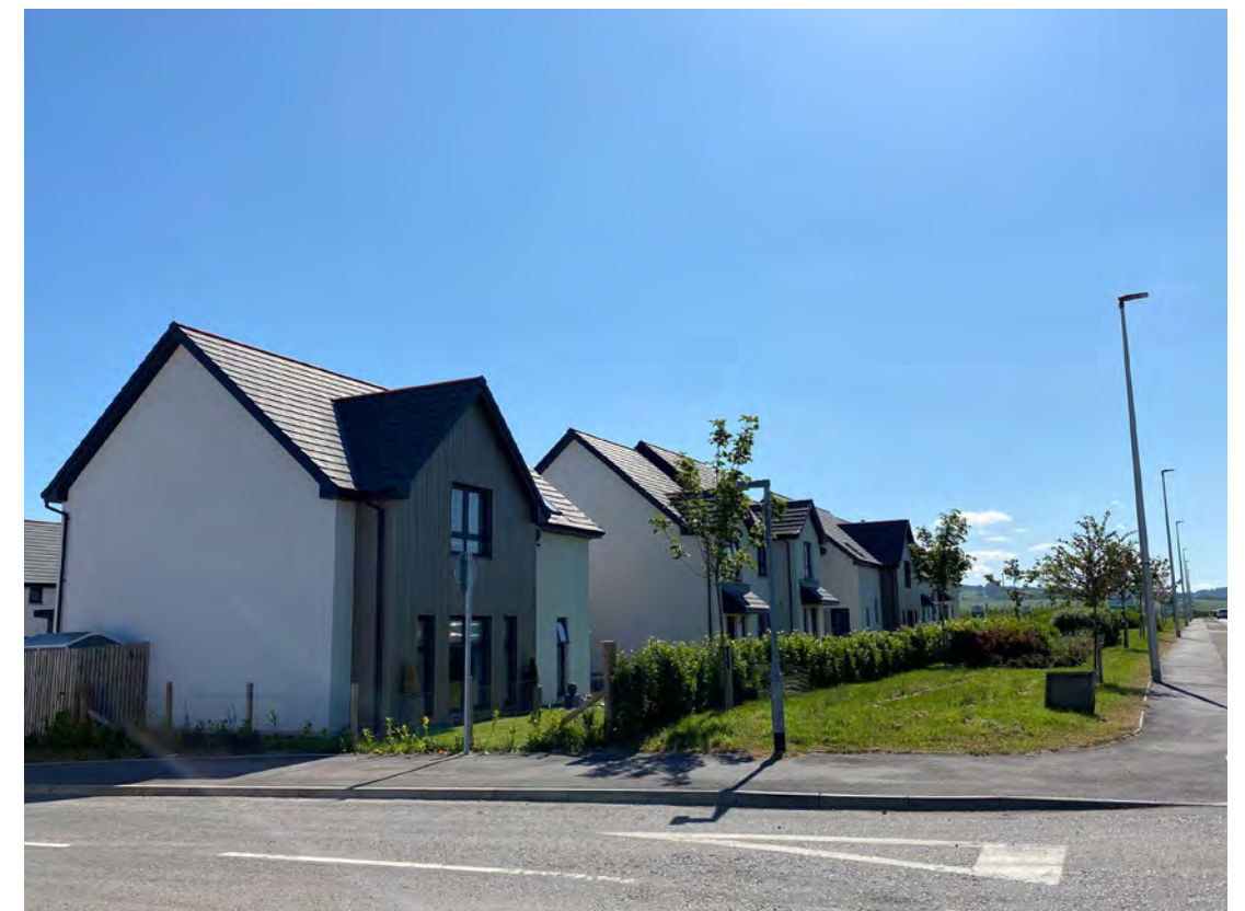
Development at Barhill Road
