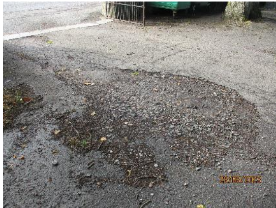
171. Eroded surface
