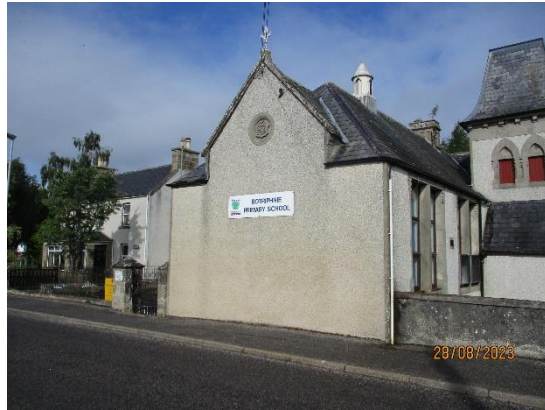
44. Stone with roughcast finish to south wing
