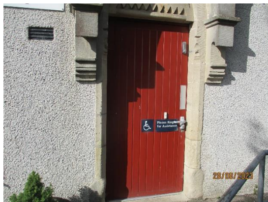
48. Timber side entrance from playground
