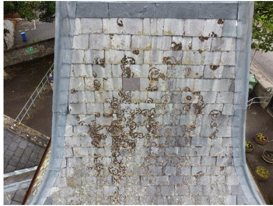
8. Slated roof to belltower
