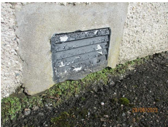
41. Ground level and underfloor ventilation
