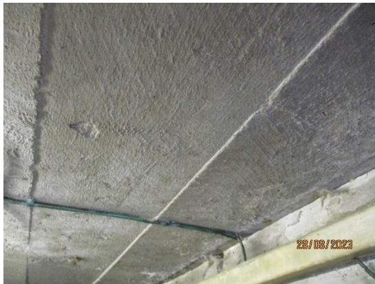
84. Concrete ceiling to the Boiler Room
