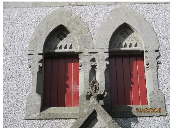
58. Timber screens to Belltower
