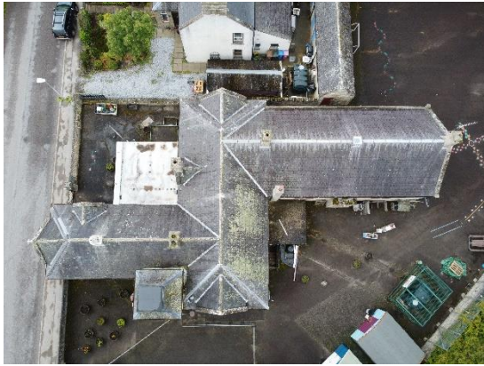
7. Overview of slated roof
