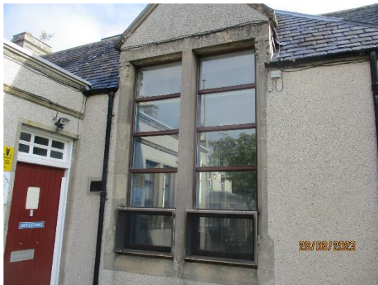
57. Large UPVC windows
