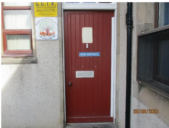
47. Timber front entrance door
