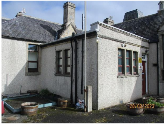
37. Metal flag pole fixed to concrete post
