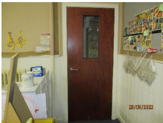
93. Timber hollow core doors
