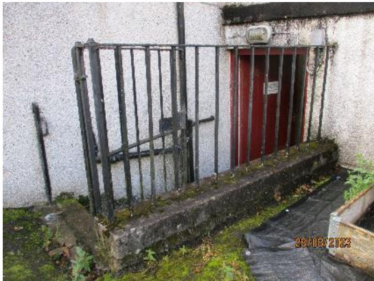
183. Metal bar fencing
