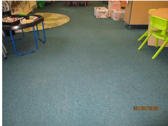
73. Carpet to classroom floors
