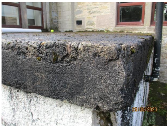
5. Concrete slab roof over boiler room
