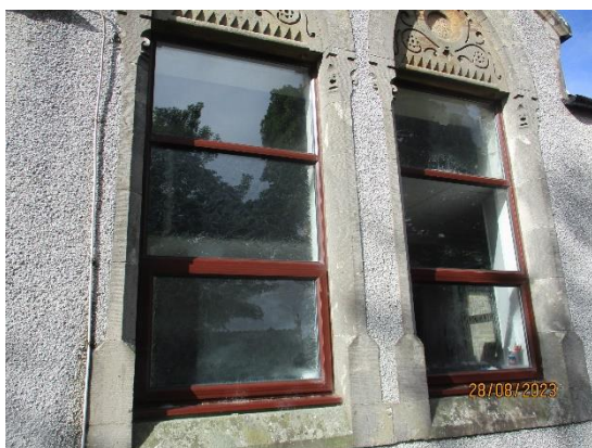
54. Typical UPVC windows
