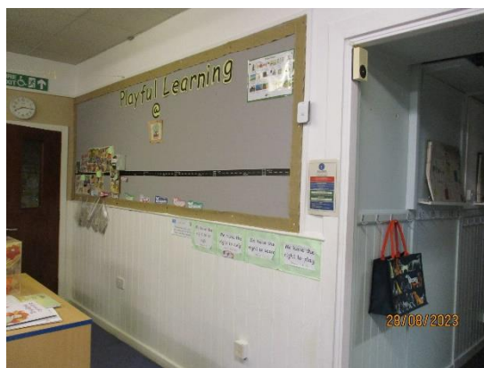
88. Low level timber linings to circulation areas
