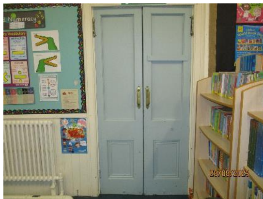
94. Timber panelled double doors
