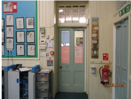
90. Timber panelled, part glazed doors
