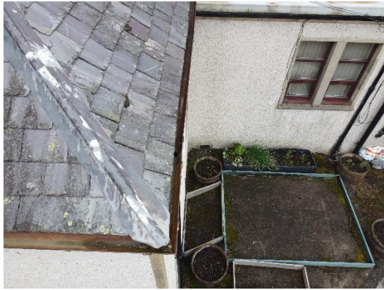
19. Cast iron 1/2 round gutters
