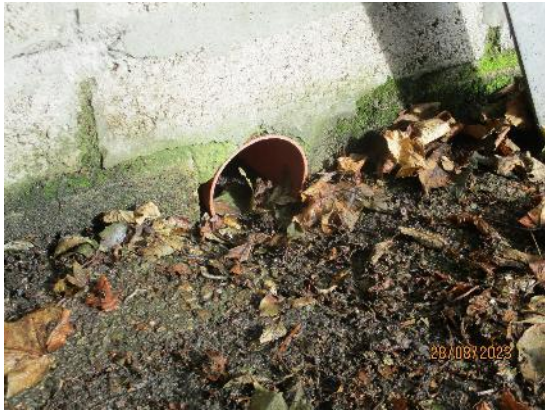
199. Playground surface water drainage by wall ducts
