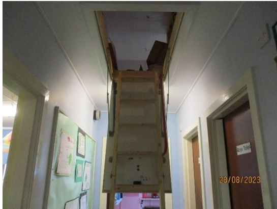
1. Access to water tank
