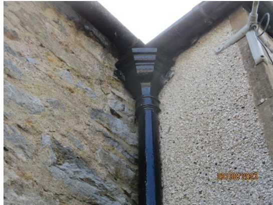
26. Cast iron hopper head and downpipe
