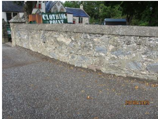
190. Natural stone wall to perimeter
