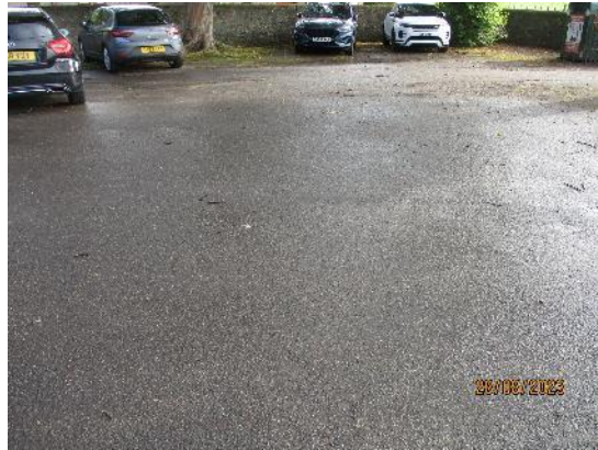
170. Tarmac car park
