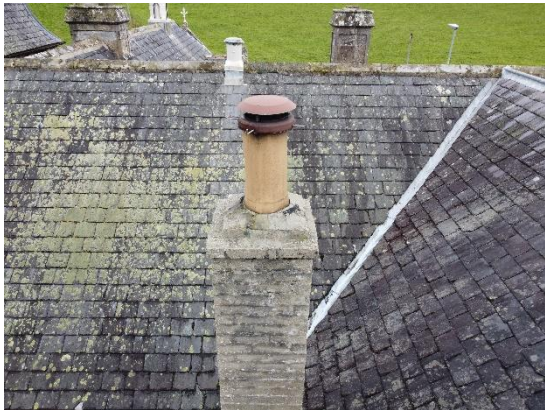
33. Boiler chimney stack
