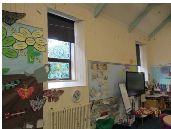
87. Timber linings to Hall
