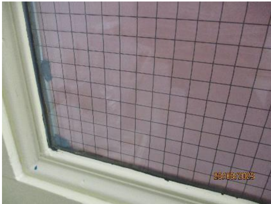
97. Georgian wired glazing to doors
