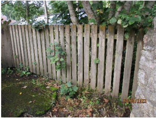
181. Timber boarded fencing
