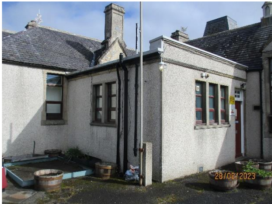
45. Masonry with roughcast finish to Reception
