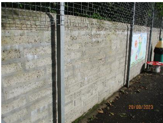
197. Concrete block retaining wall
