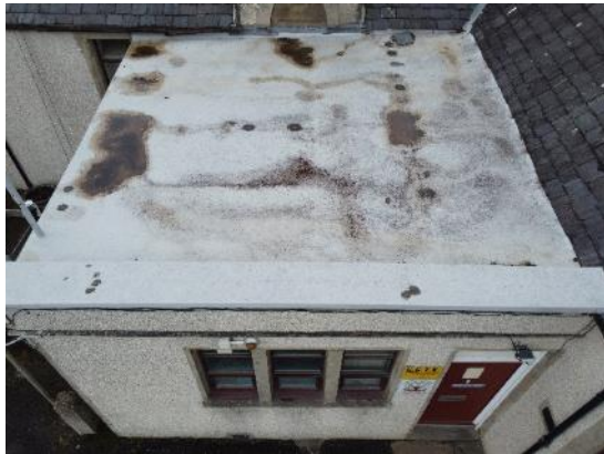
15. GRP roof to Reception
