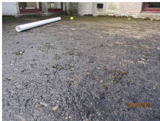
6. Concrete slab surface
