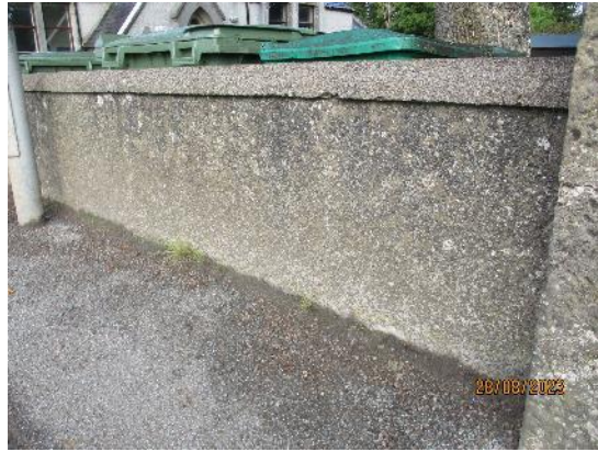
194. Masonry roughcast wall
