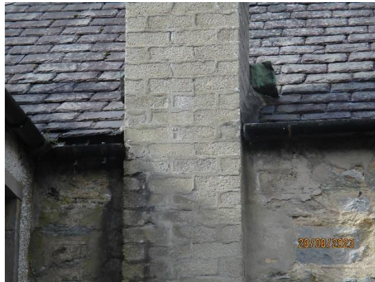
34. Brick boiler flue
