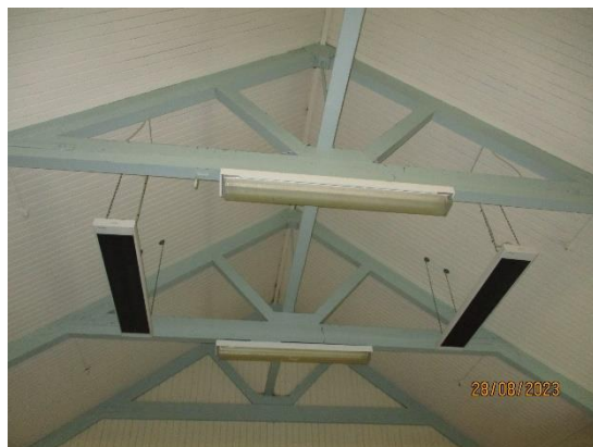
83. Timber linings to Hall ceiling (1/6)
