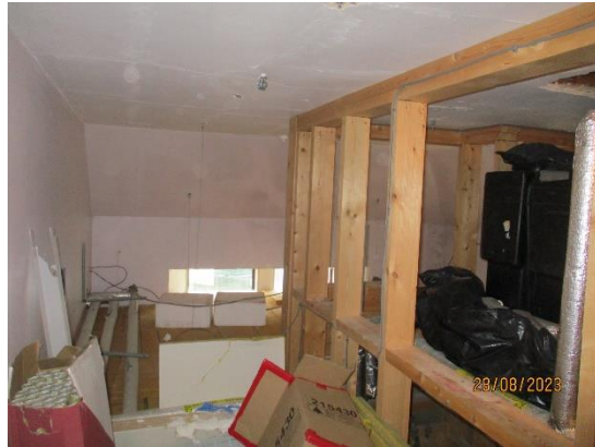
2. Roof void below structure
