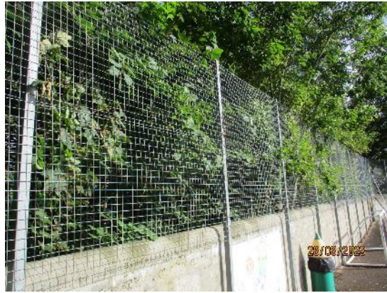
182. Chain link fencing
