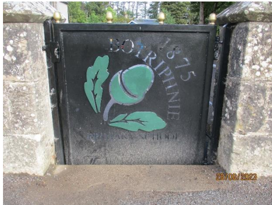
64. Painted metal gates
