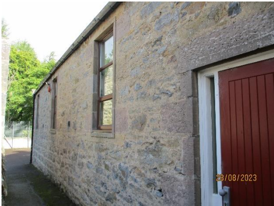
39. Stone walls to main school building
