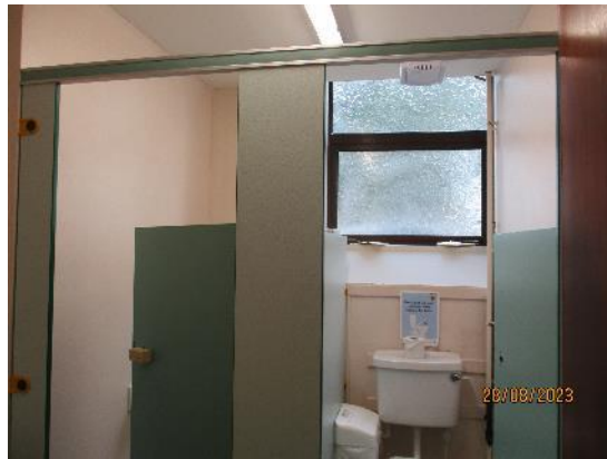
108. Composite panel toilet cubicles
