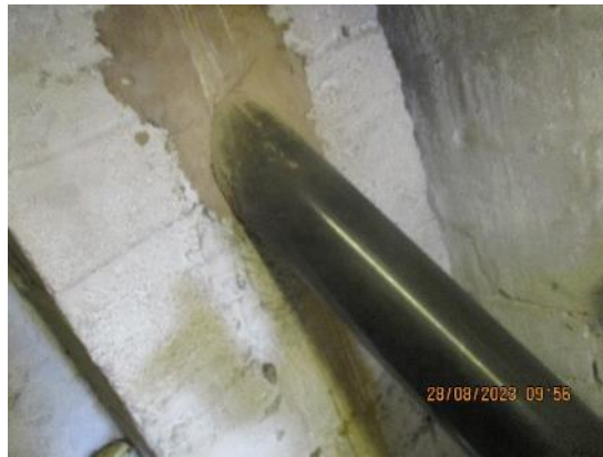
128. Boiler flue from appliance to brick chimney 0/14.
