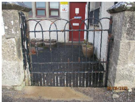
186. Metal hoop main entrance gate
