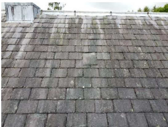
11. Isolated slipped slates
