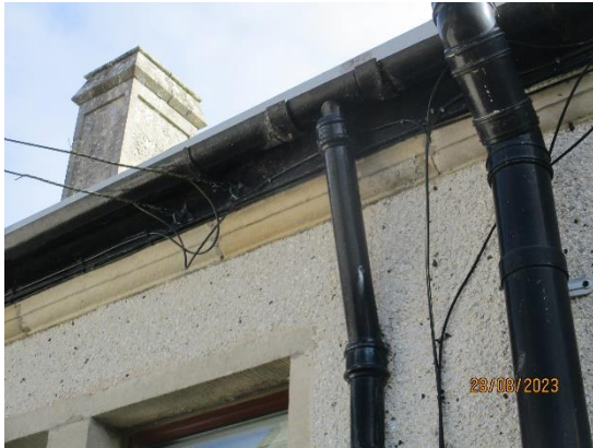
25. Cast iron downpipes
