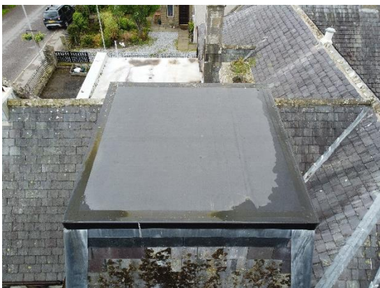
17. SPM roof to belltower
