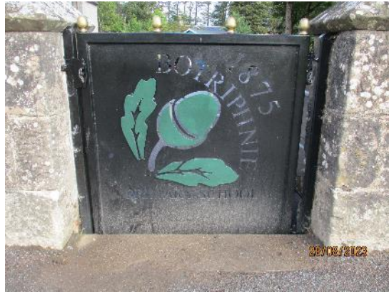
188. Steel plate gate to side entrance
