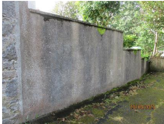
196. Masonry and smooth render wall
