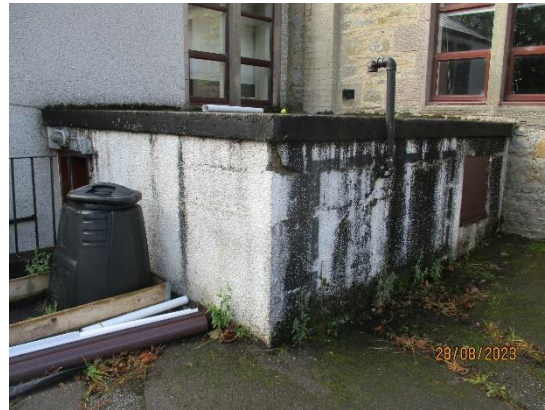
40. Blockwork walls – Reception & Boiler Room
