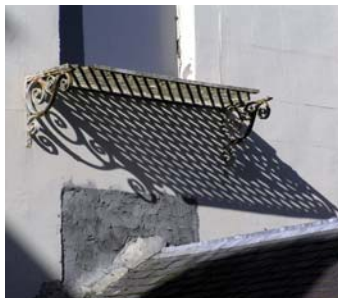
Surviving cast-iron balcony on the east elevation of the north wing
