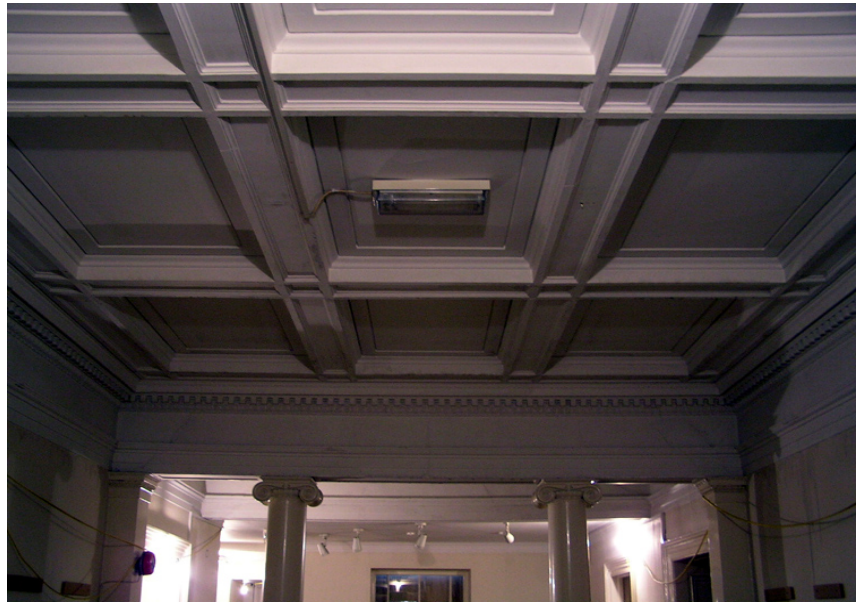
Coffered ceiling to the entrance hall and screen
