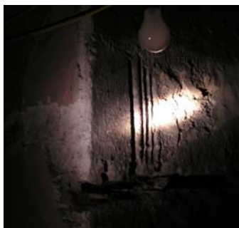
Dressed masonry reused within the roofspace at Grant Lodge
