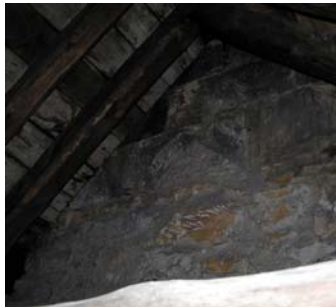
Evidence of earlier reused masonry to the party walls within the roofspace
