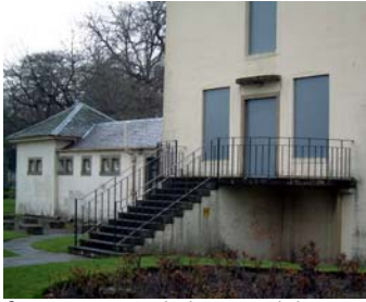
Concrete steps, balcony and door added in 1953
