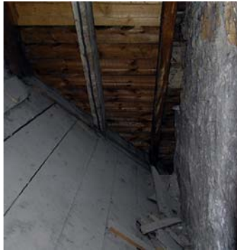
Evidence of the sarking to the original hipped roof still in position within the roofspace
