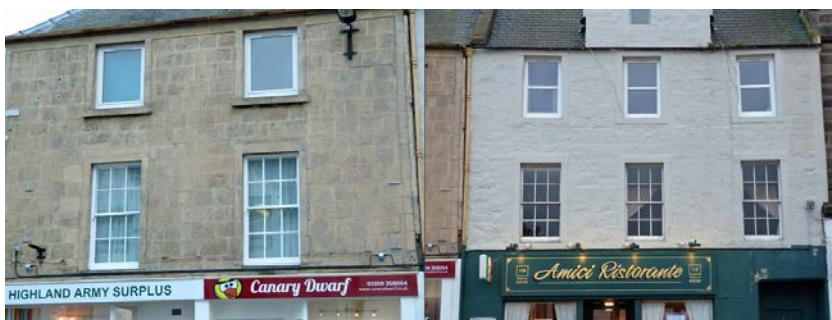
Properties on the High Street where window replacements no longer match the patterns or design of the traditional windows on the lower storey
