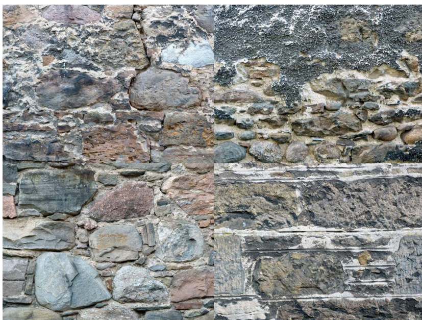
Rubble walling, lime pointing and sneck harling
