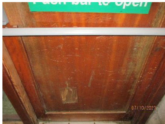
323. External timber doors
