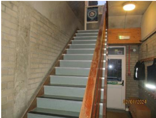
180. Concrete stairs – Leisure Centre
