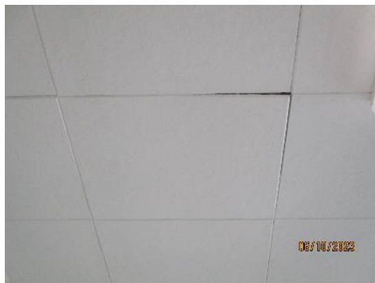
199. Fibre ceiling tiles
