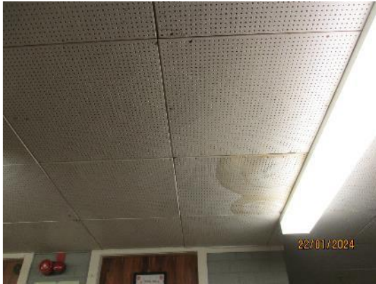
212. Watermarked fibre tiles – Leisure Centre
