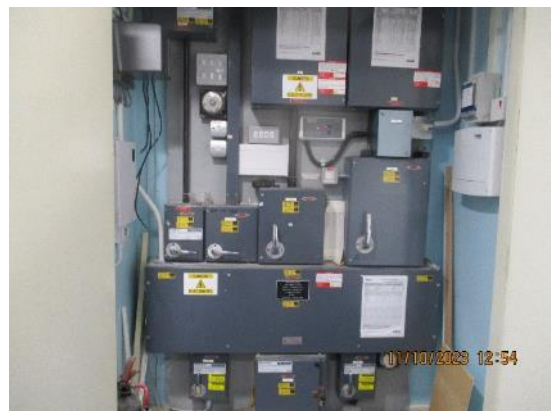
397. Switchgear and busbar – Music block.
