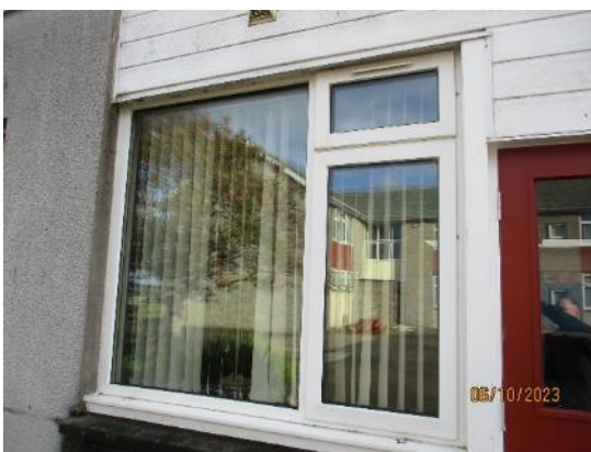
116. PVC windows – Block M
