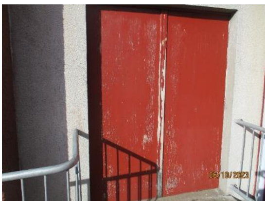
101. Timber double fire escape doors
