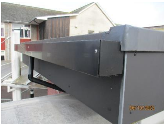
53. Metal box gutters to new entrance
