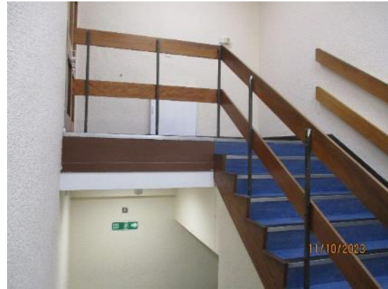
191. Metal and timber balustrades – Block K
