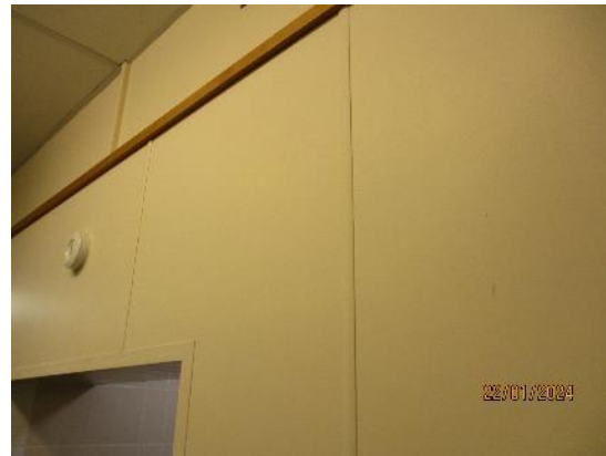
243. Composite panelling – Leisure Centre
