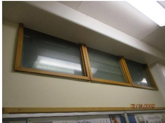
251. Timber borrowed lights - School
