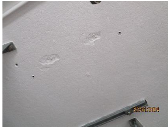
215. Concrete ceilings – Plant rooms
