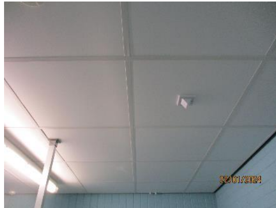
209. Suspended ceiling tiles – Leisure Centre
