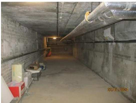
147. Suspended concrete floor around pool
