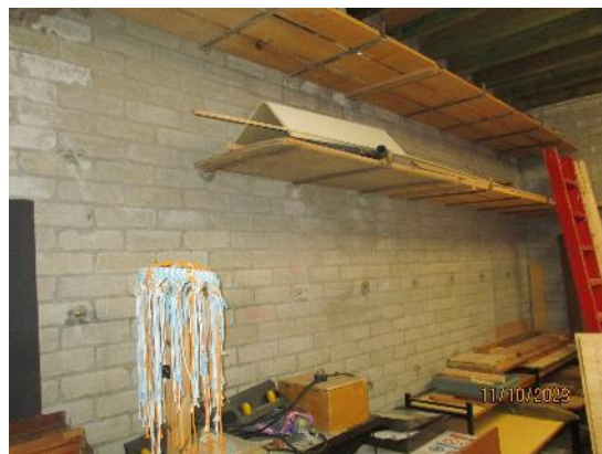
217. Brick external walls
