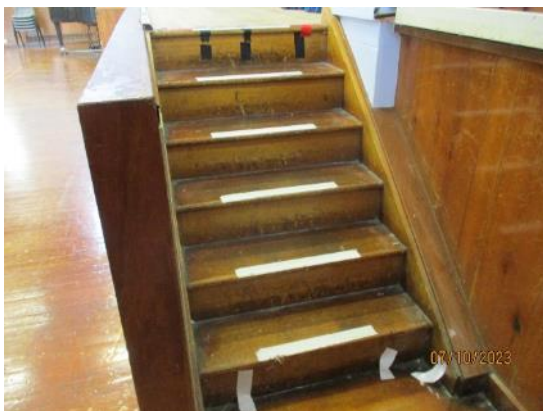
176. Timber stairs to the stage
