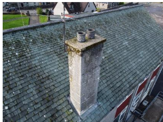
72. Masonry chimney stack
