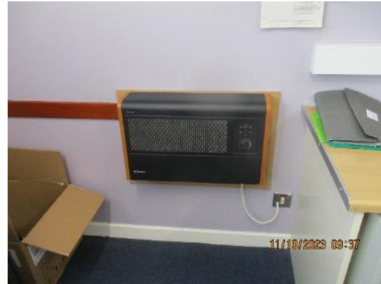
357. Electric fan convector K Block typical.
