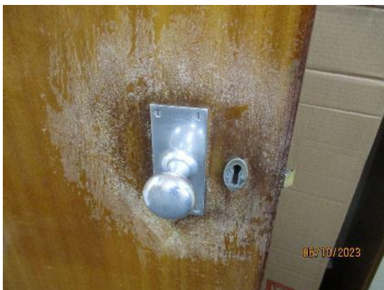
258. Varnished timber doors
