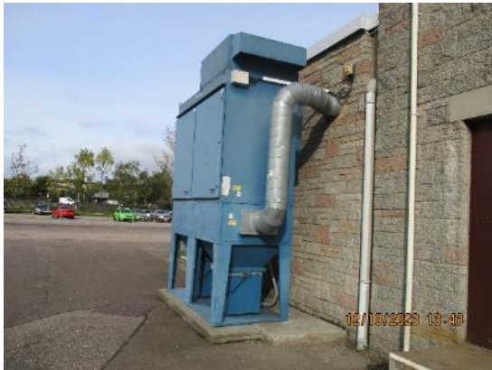
388. LEV collection unit and fan – Technology dept.
