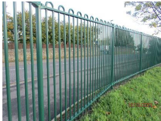
527. Security metal bar fence, to road
