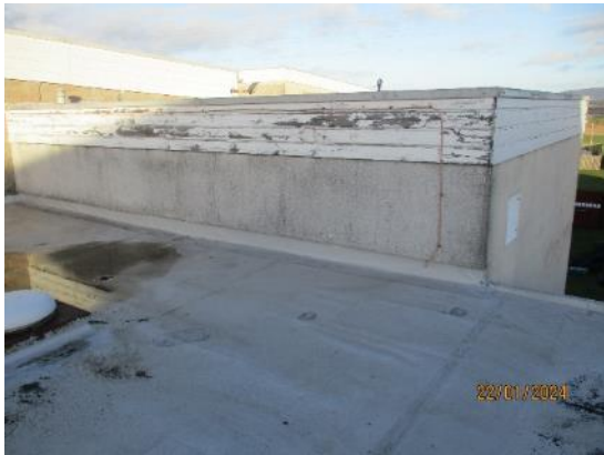
45. Timber fascia boards - School
