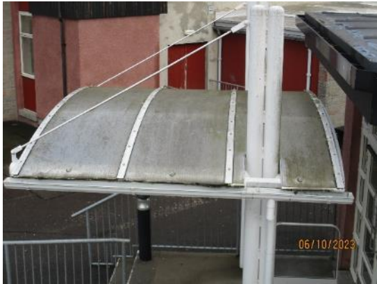
143. Polycarbonate canopy to new entrance
