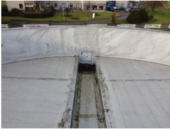
37. SPM box gutter above Meeting Room
