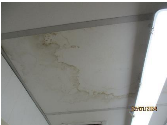
210. Watermarked suspended ceilings
