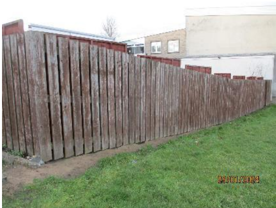
532. Timber boarded fence to playgroup
