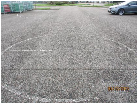
506. Tarmac rear access road
