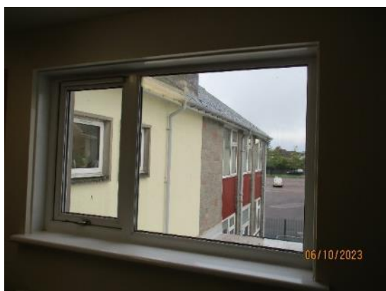
111. PVC windows internally
