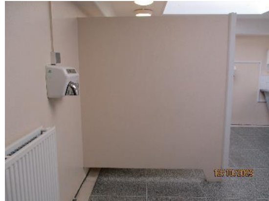
219. Terrazzo partitions in Toilets/Changing Rooms
