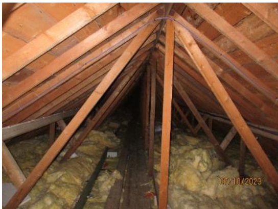
5. School timber pitched roof
