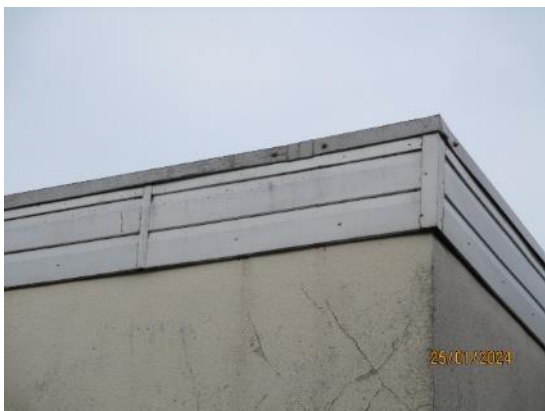
47. PVC fascia boards – Leisure Centre
