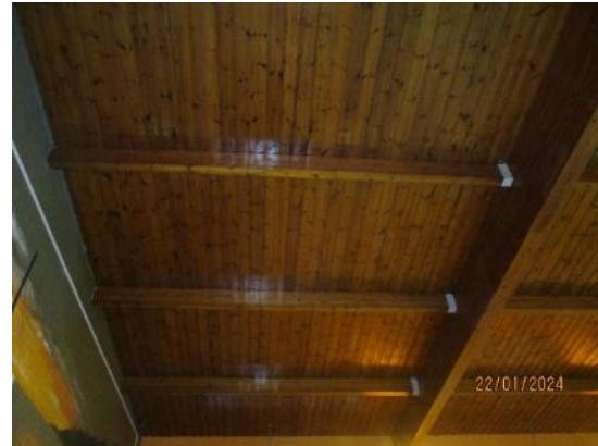
8. Glulam beams – Swimming Pool
