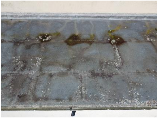
31. GRP bubbling and blistering
