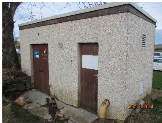
559. Gas meter house with metal profile roof
