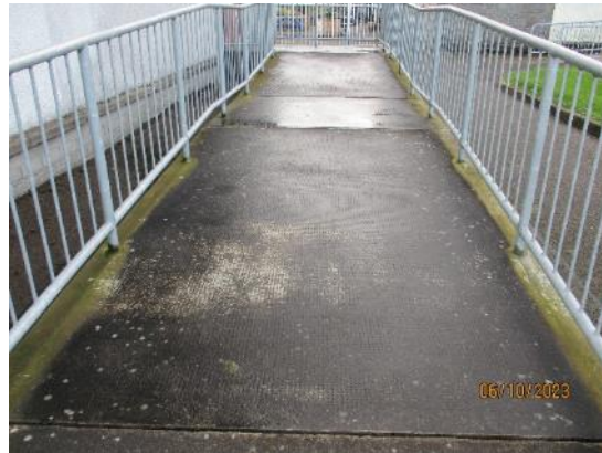
140. Concrete ramps to fire exits
