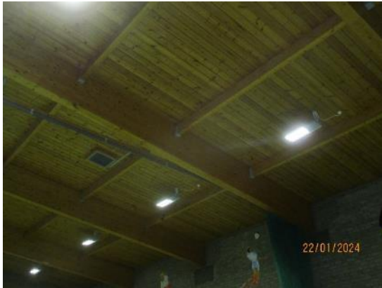
7. Glulam beams – Games Hall
