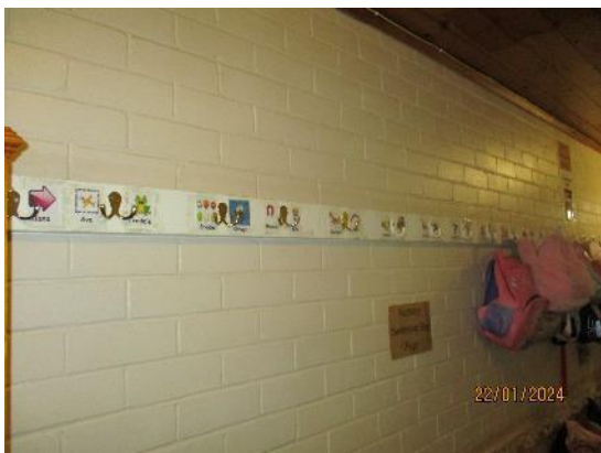
240. Brickwork internal walls
