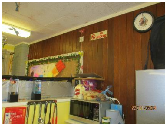
241. Timber linings – Leisure Centre
