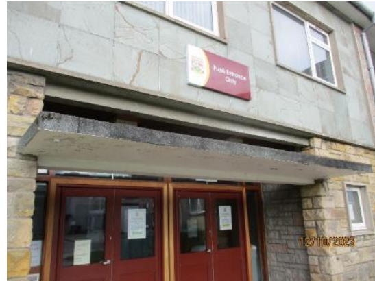
144. Concrete/felt canopy to pupil entrance
