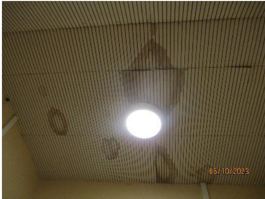
200. Water marked fibre ceiling tiles
