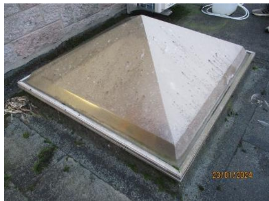
42. GRP rooflights to Leisure Centre
