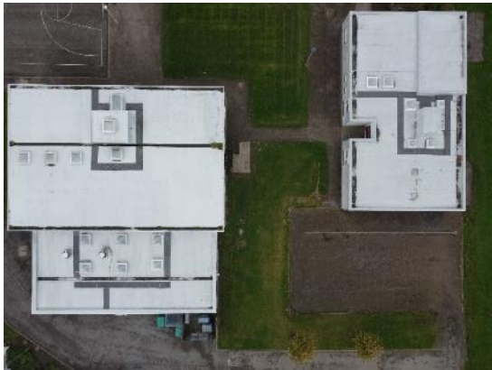
21. Single ply membrane to Blocks K and M
