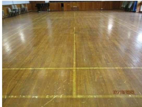
158. Timber floor boards
