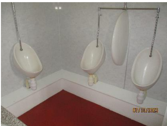
233. Wetwall in toilets
