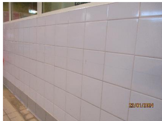
247. Ceramic tiles around the pool
