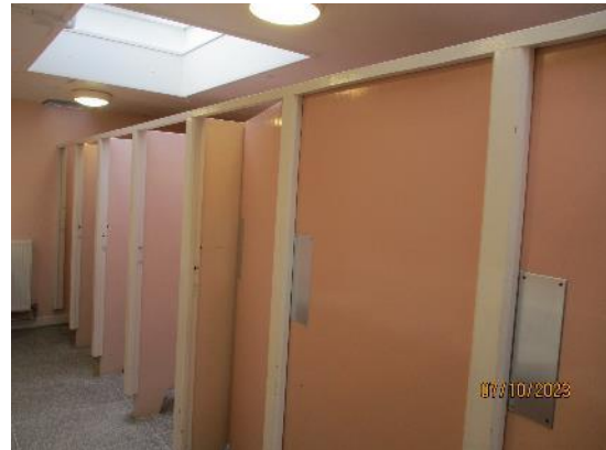
263. Timber cubicle doors
