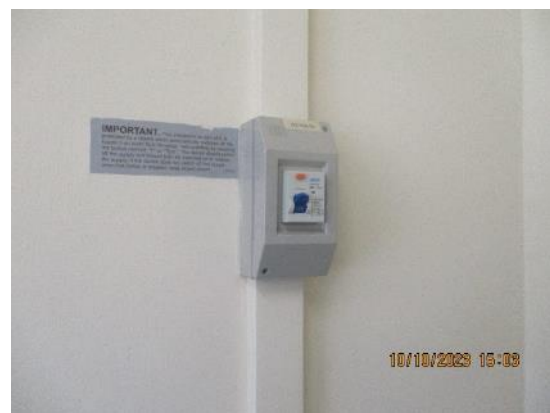
403. 32A RCD – classroom typical.
