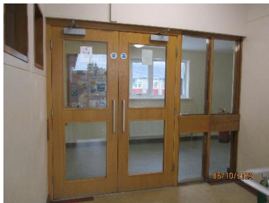
253. Glazed screens - School
