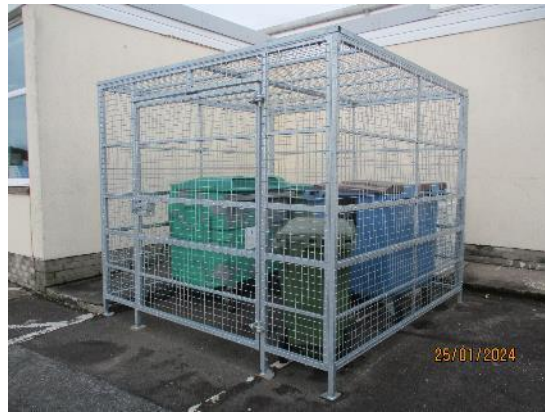
549. Caged bin enclosure – Leisure Centre
