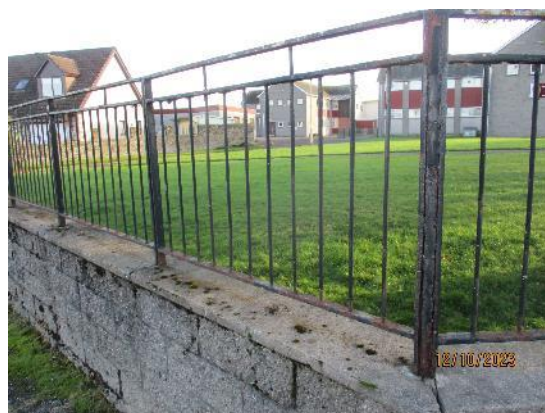
529. Metal railings to rear entrance
