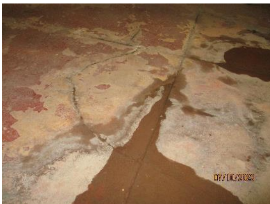
322. Painted concrete floors
