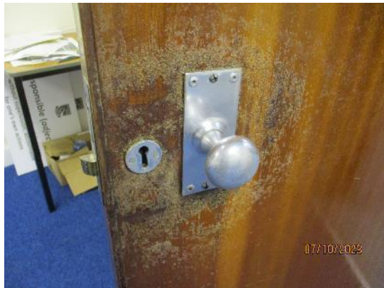
324. Internal timber doors
