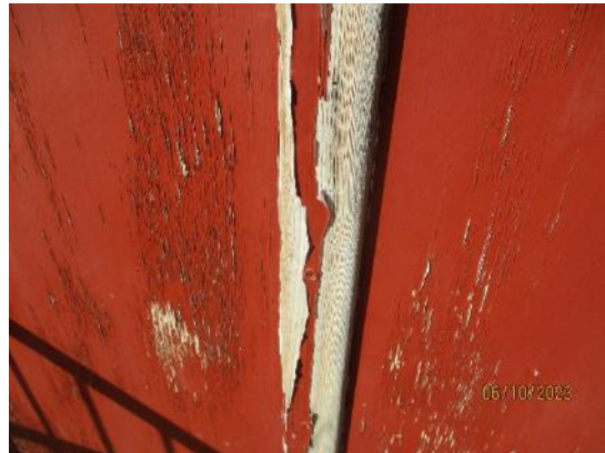
128. Timber external doors
