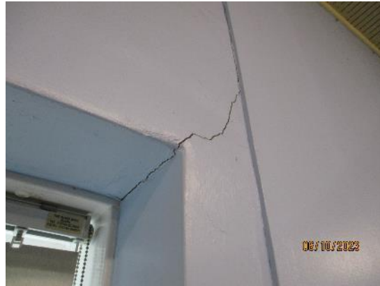
225. Cracked plaster
