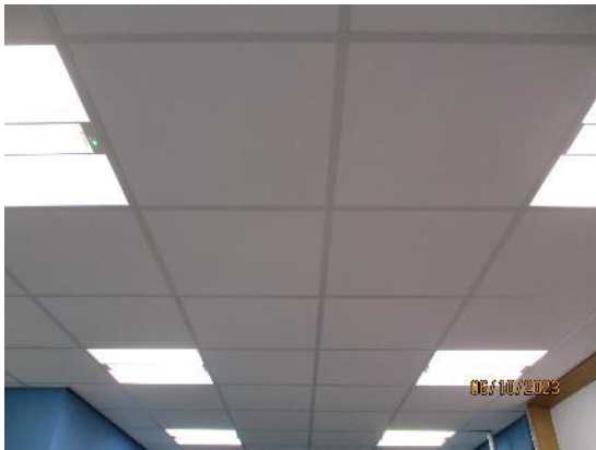
194. Suspended ceiling tiles - School
