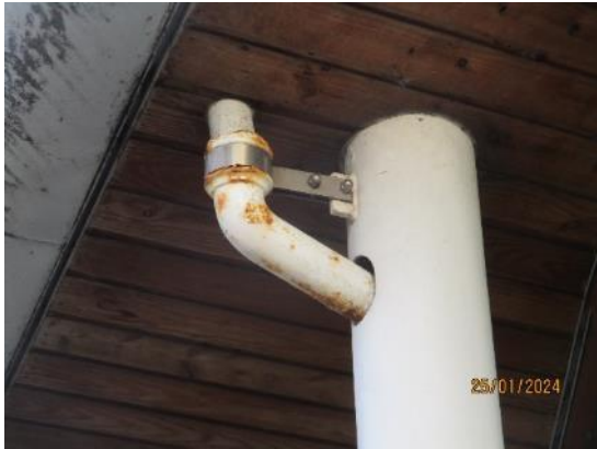
67. Cast iron downpipes – Leisure Centre
