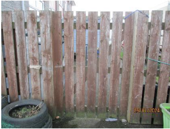
536. Timber boarded gate to playgroup
