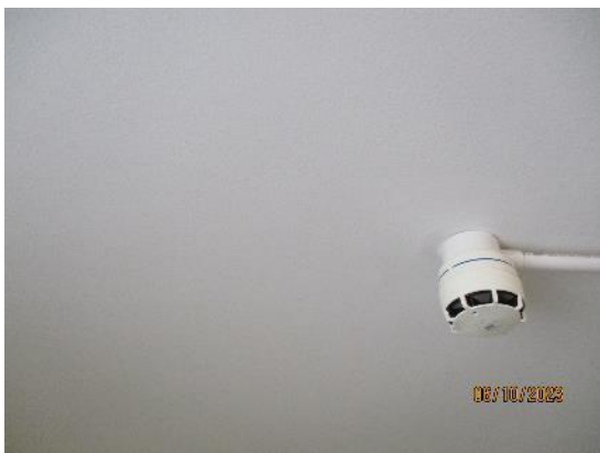
204. Plaster/plasterboard ceilings - School
