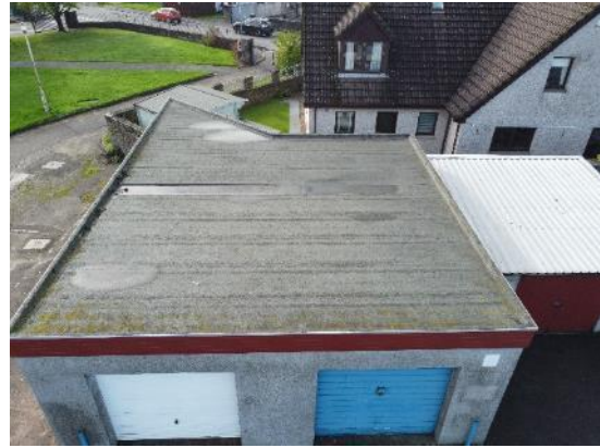
20. Mineral felt to Shelter and Garage
