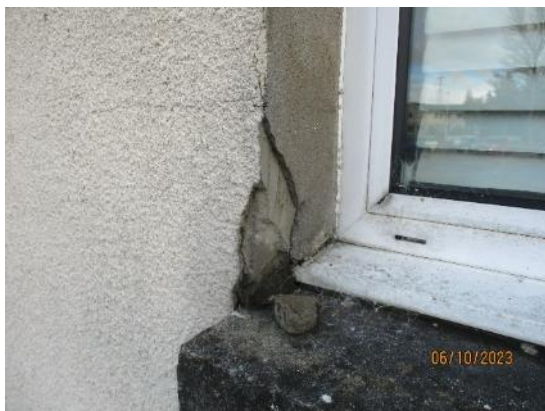
77. Cracked roughcast
