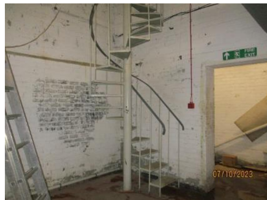
177. Metal spiral stair to boiler room
