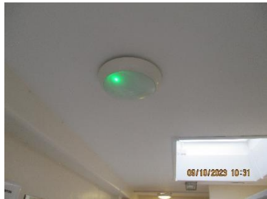
407. Lighting 1/74 girls toilets main school.
