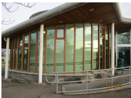
117. Timber curved screen – Leisure Centre
