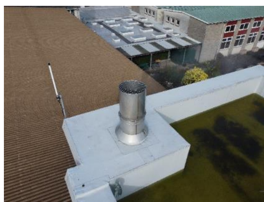
445. Boiler chimney termination roof view.
