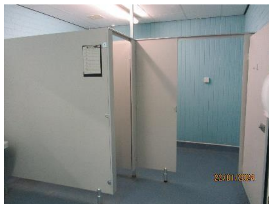
300. Toilet cubicle partitions
