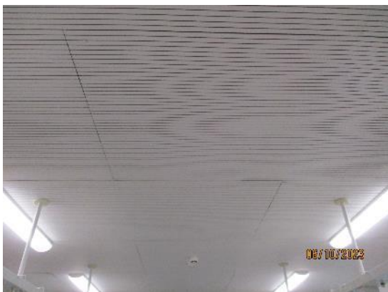
198. Ribbed fibre ceiling tiles
