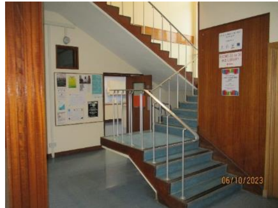
175. Concrete stairs - School
