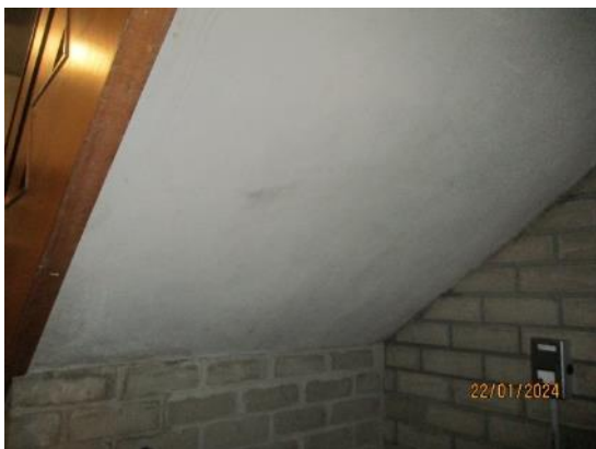
188. Plastered soffits – Leisure Centre
