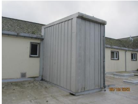
86. Metal profile lift enclosure
