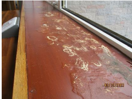
249. Blistered, laminating window sills
