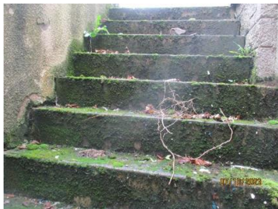
136. Concrete steps to boiler room
