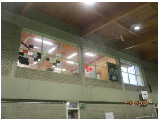
252. Powder coated borrowed lights – Leisure Centre
