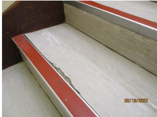
185. Damaged treads
