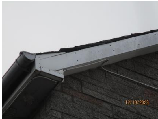
44. PVC fascia and barge boards - School
