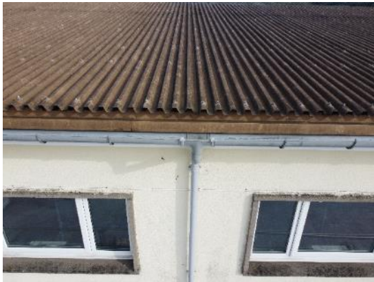
51. UPVC gutters - School
