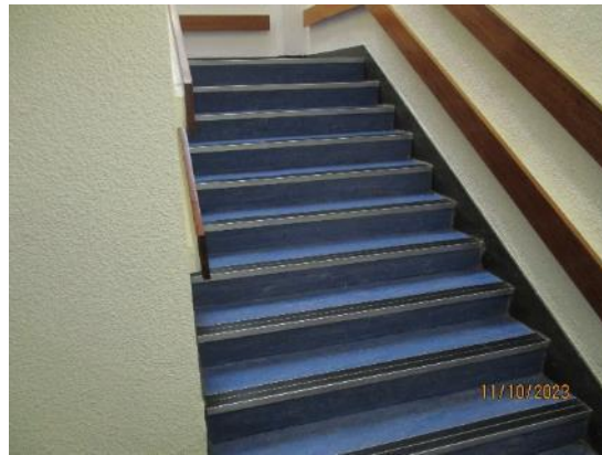
179. Concrete stair to Block K
