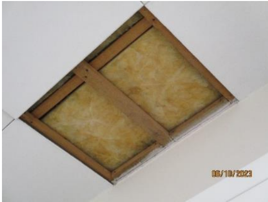
49. Mineral fibre insulation to flat roofs - School
