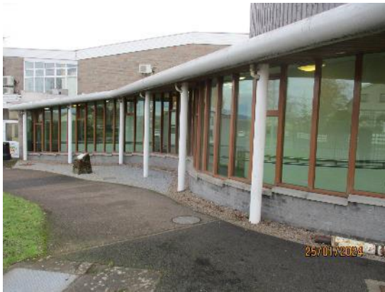
524. Tarmacadam footpath – Leisure Centre
