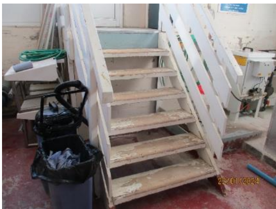
182. Timber stair in Plant Room
