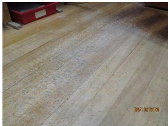
160. Timber boards to store rooms
