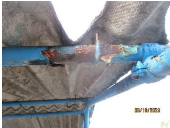
134. Metal frames to outbuildings
