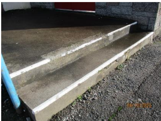
135. Concrete steps to fire exits
