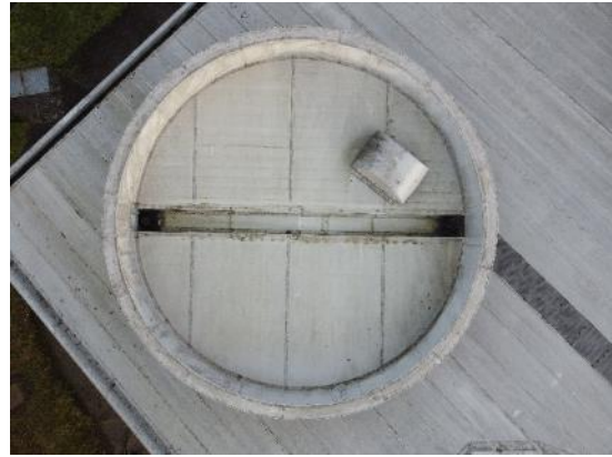
26. Circular roof above Meeting Room
