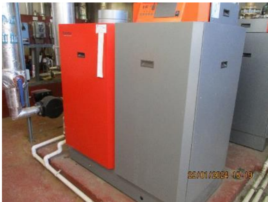
446. Natural gas condensing boiler
