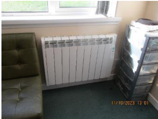
358. Rointe electric panel convector – M Block typical.
