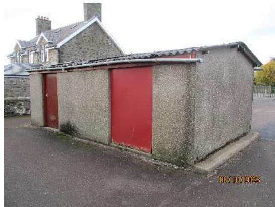
551. Brick external store with asbestos roof
