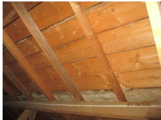
6. Timber sarking boards
