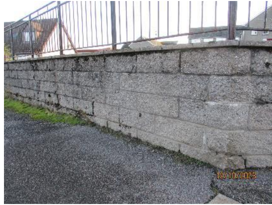
537. Concrete block wall to rear
