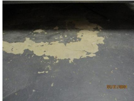
173. Painted concrete floors
