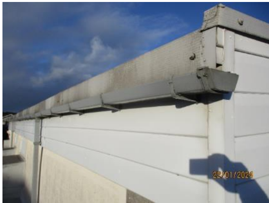
55. UPVC gutters – Leisure Centre
