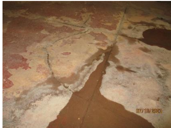
163. Painted concrete floors
