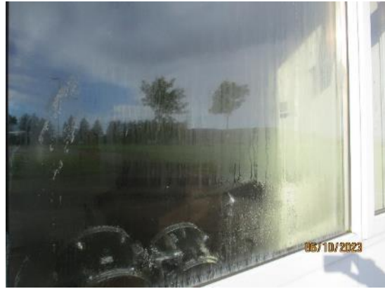
122. Blown double glazed units – Block M
