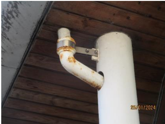
127. Cast iron downpipes
