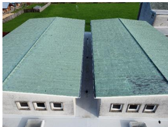
12. Copper roofs to Gym Halls
