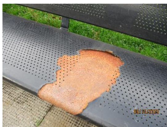
517. Surface peeling and corroding
