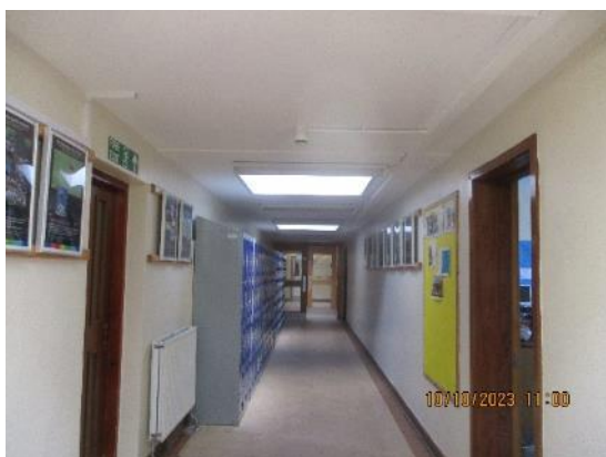
410. Lighting – corridor of main school typical.
