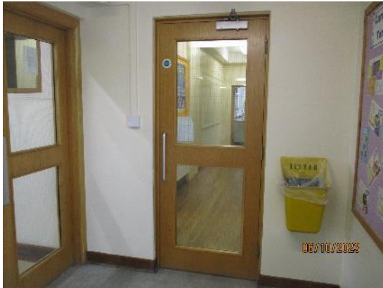
254. Timber veneered doors - School
