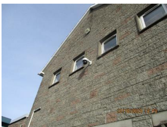
444. CCTV camera external. Main building.
