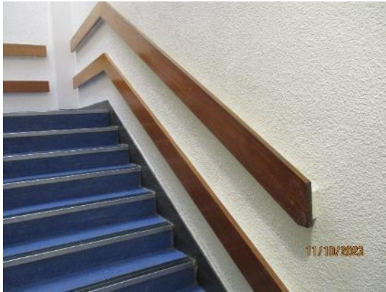
190. Timber handrails – Block K
