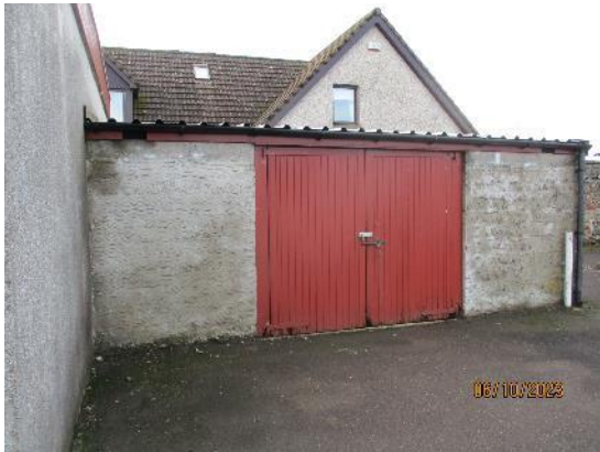
556. External store with metal profile roof
