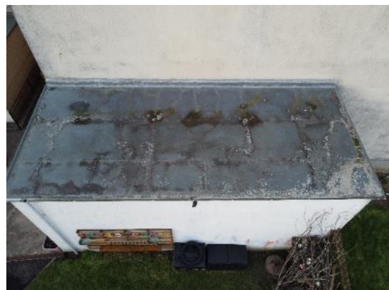
30. GRP roof above Games Hall Store
