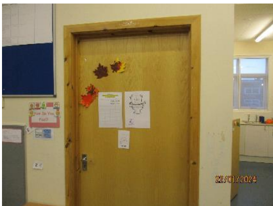
270. Timber veneered doors
