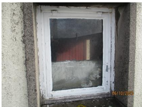
113. Timber windows – water tank house
