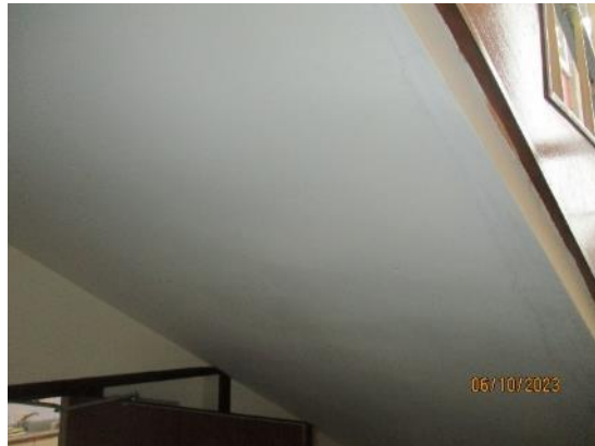
187. Plastered soffits - School
