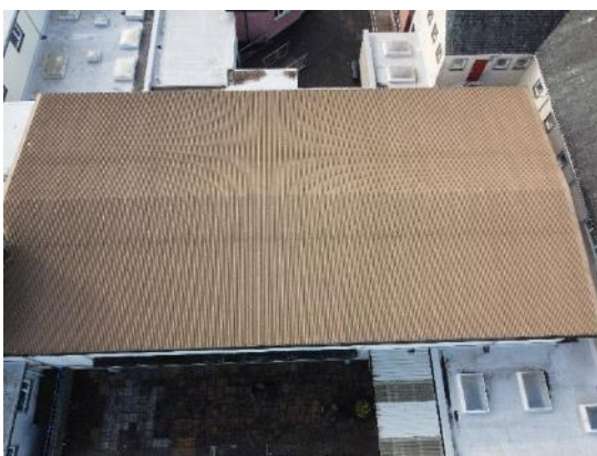
14. Metal profile roof to Hall and Stage
