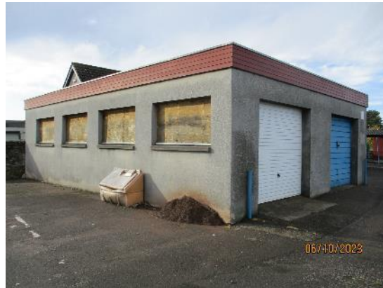
557. Brick garages with felt roof
