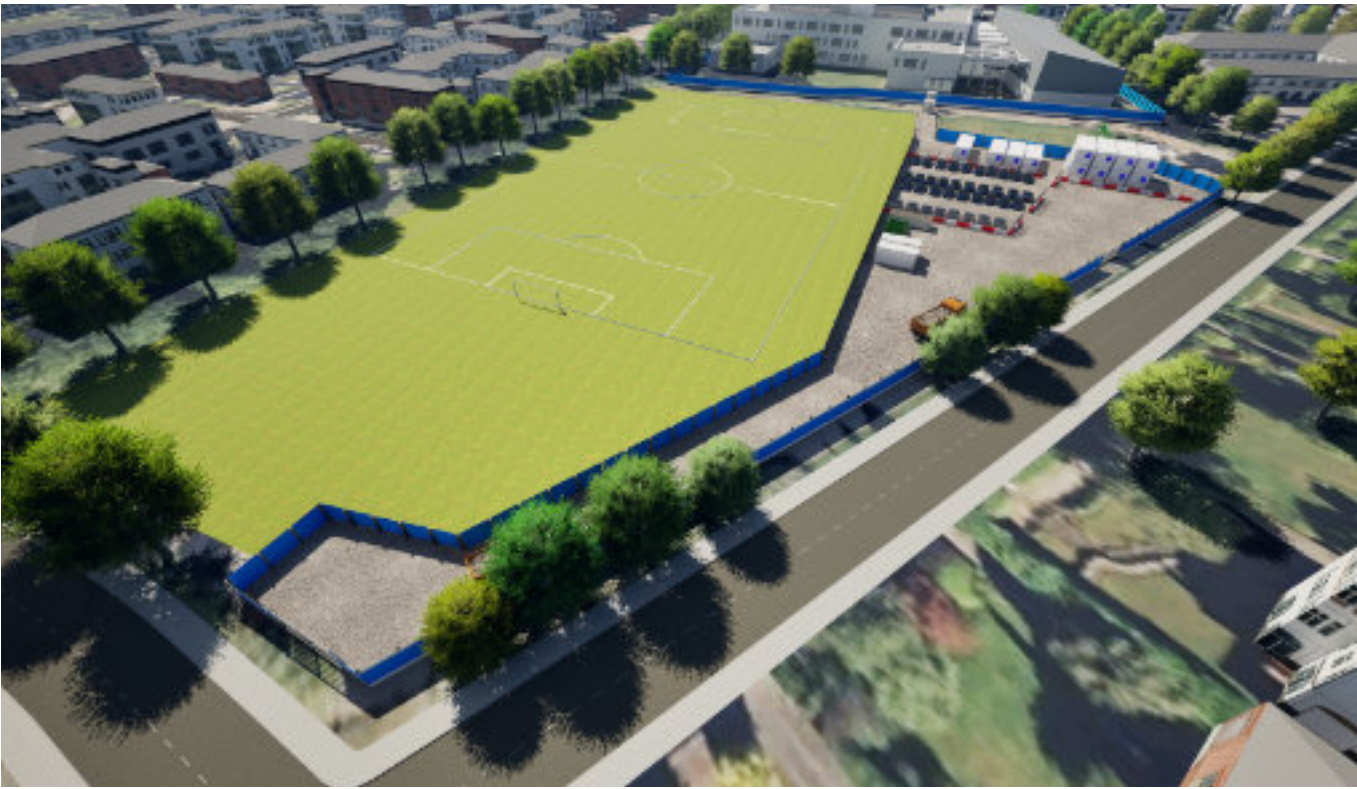
Aerial view of contractor's compound during Phase 1
