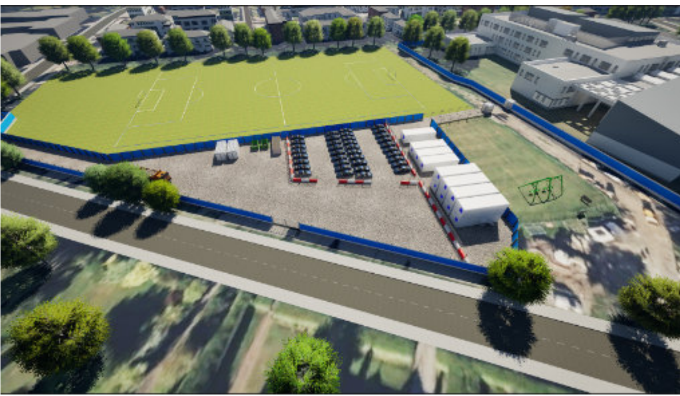
Aerial view of contractor's compound during Phase 1
