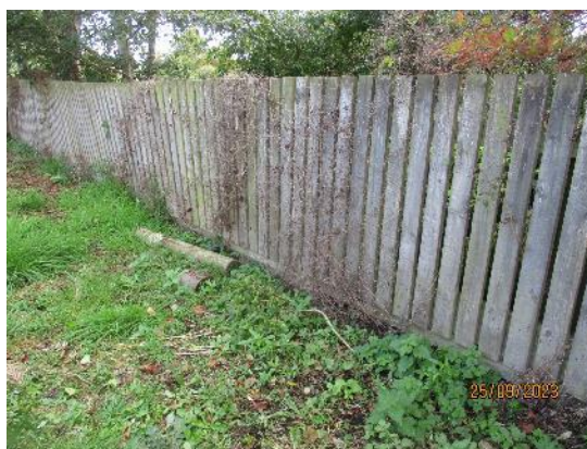
213. High timber boarded fencing
