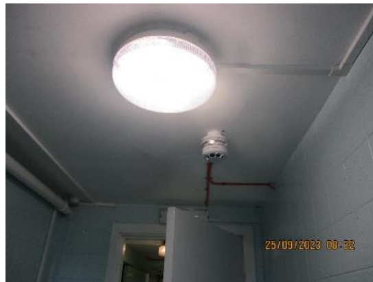
193. Combined smoke detector and sounder.
