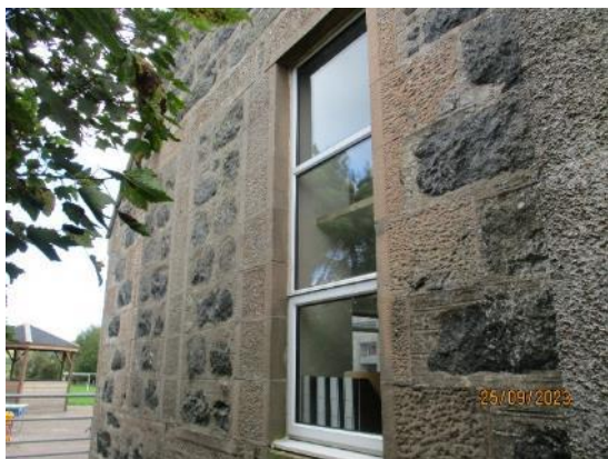
59. Large UPVC windows
