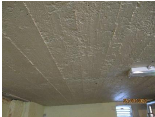
109. Concrete ceiling to Boiler Room
