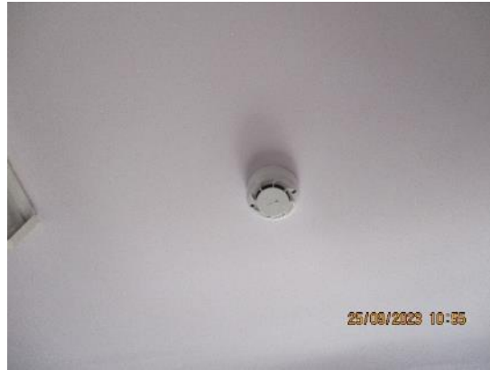
191. Smoke detector typical.
