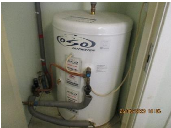
168. Hot water cylinder – kitchen supply.
