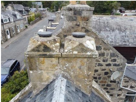
33. Capped and ventilated chimney stack
