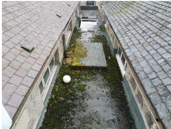
9. Felt roof above corridor
