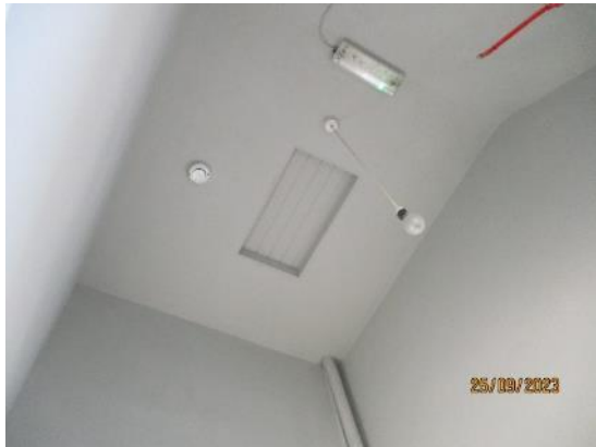
104. Lath & plaster ceilings
