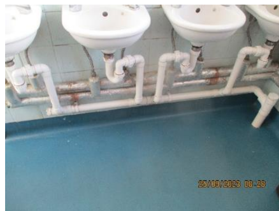
171. Pipework – hot and cold / boys toilets.
