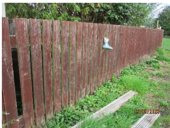
212. Timber boarded fencing
