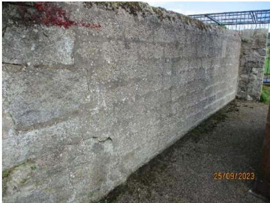
228. Concrete block wall
