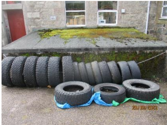
51. Roughcast walls to Boiler Room
