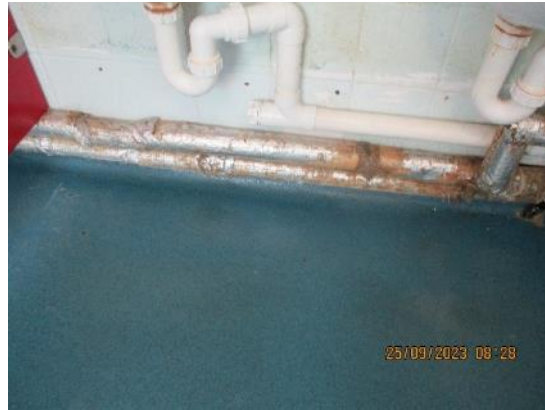
173. Pipework – hot and cold boys toilets.
