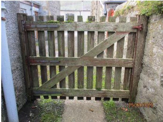
220. Timber boarded gates
