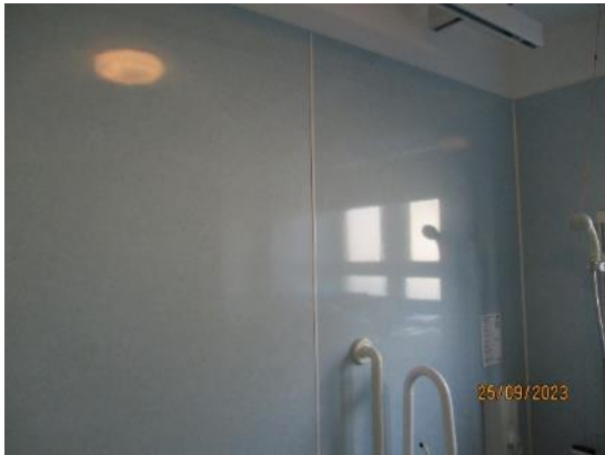
116. Wetwall in Shower Room
