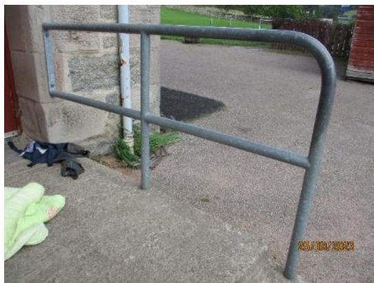
77. Galvanised tubular guard rails
