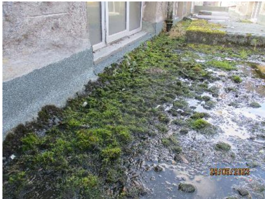
10. Extensive moss growth trapping water
