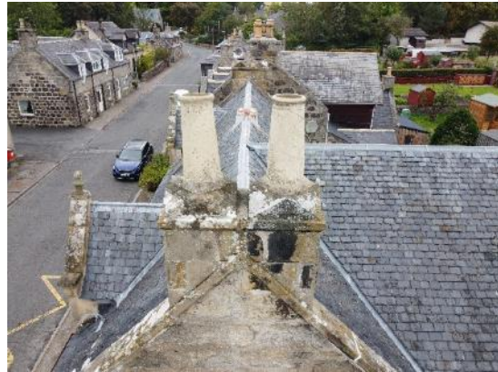
32. Stone chimney stack
