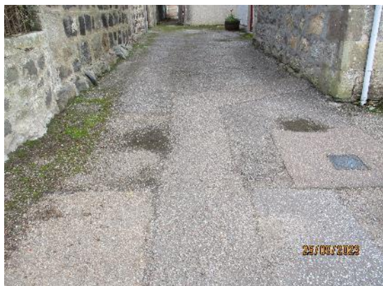
210. Tarmacadam entrance footpath
