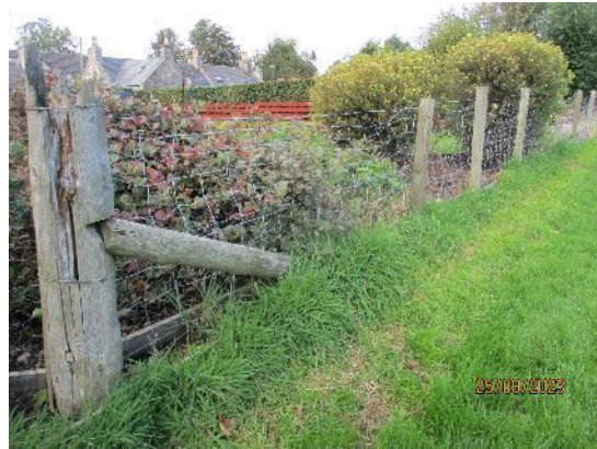
215. Timber post & wire fencing
