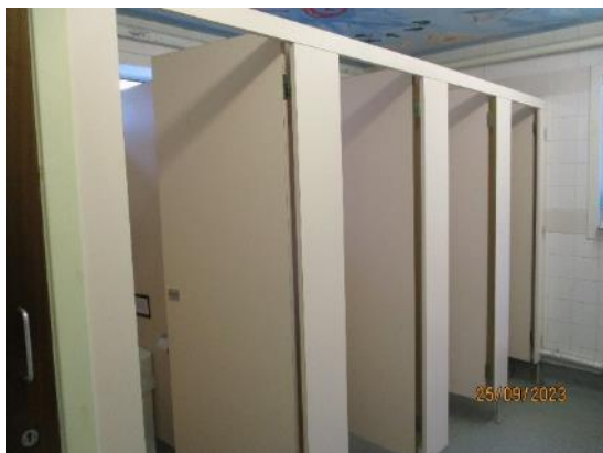
136. Composite panel toilet cubicles
