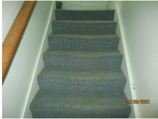
92. Timber stair to first floor
