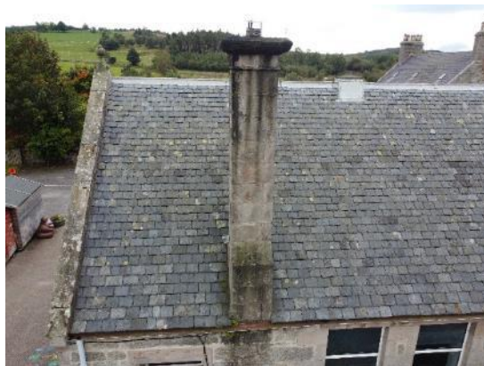
35. Stone boiler flue
