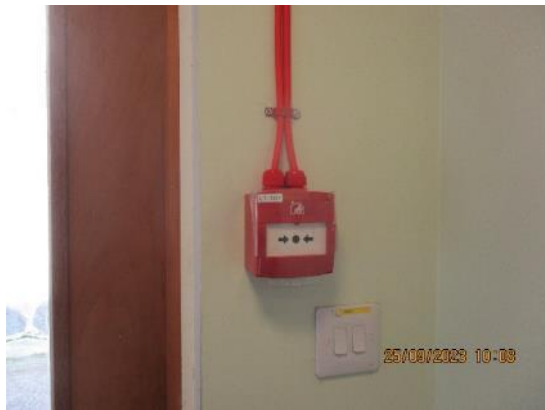
192. Fire alarm system call point typical.
