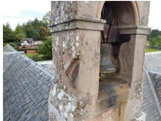
40. Cracked/spalling stonework
