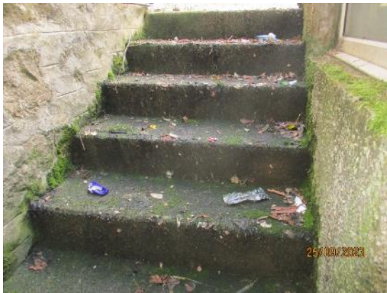
73. Concrete steps to Boiler Room
