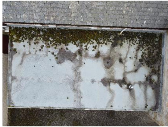
14. GRP roof above Kitchen and entrance
