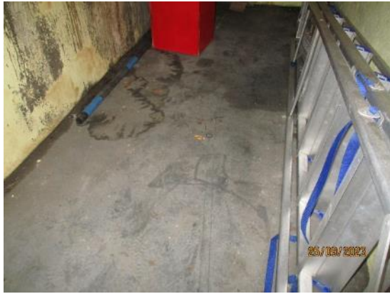
91. Concrete floor in Boiler Room
