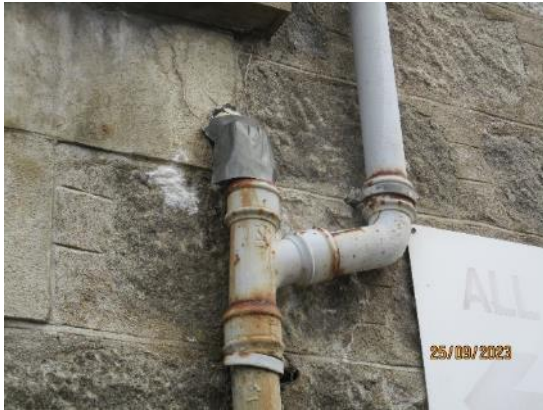
31. Patch repair to cast iron downpipe
