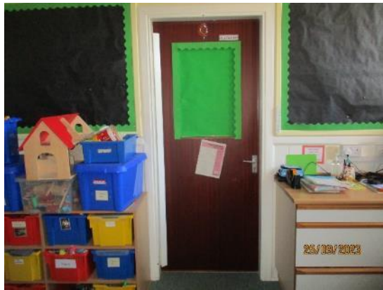
121. Timber veneered doors to classrooms
