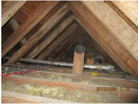
1. Timber trussed roof above two storey part
