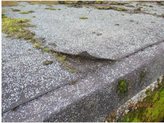
13. Felt lifting at edges
