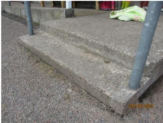
75. Concrete steps to Play Group entrance
