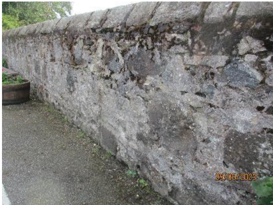
222. Natural stone perimeter walls
