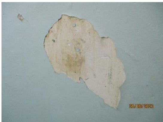
148. Lath & plaster walls
