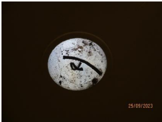
21. Cleaning of sunpipes required
