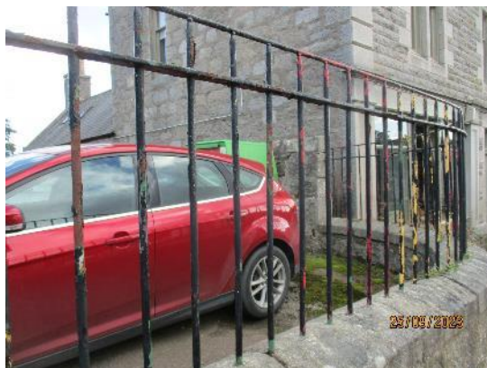
211. Metal railings above stone wall
