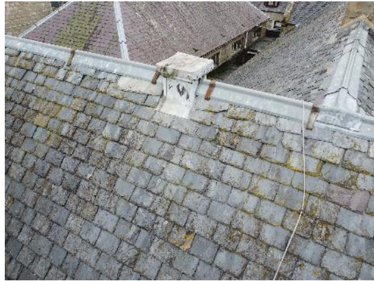
4. Isolated slipped slates
