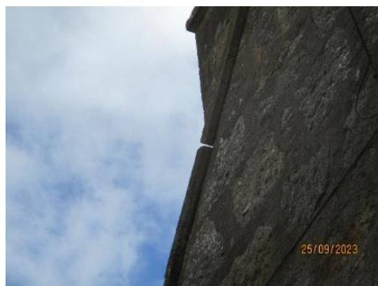
48. Repointing of skew stones
