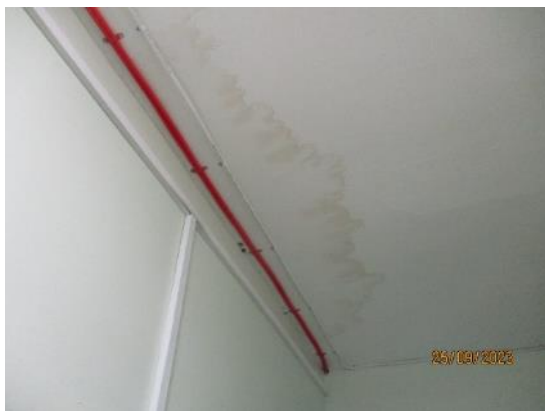
100. Watermarked plasterboard ceilings
