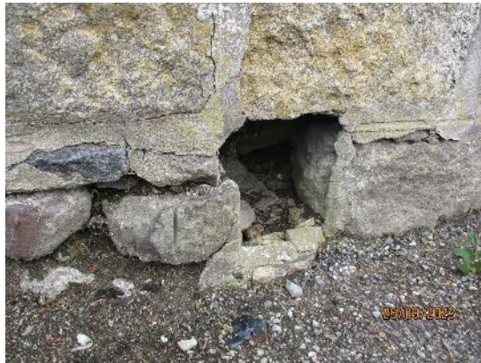
223. Isolated repairs and repointing
