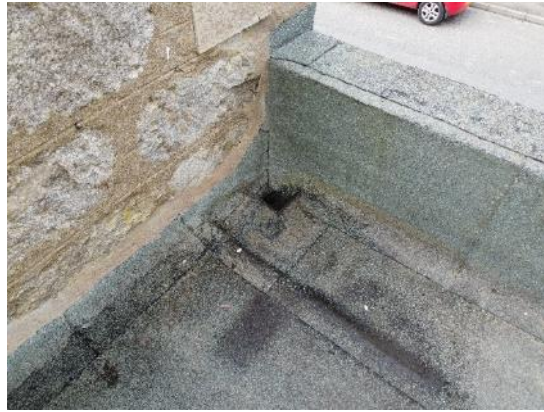
26. Rainwater outlet from felt flat roof
