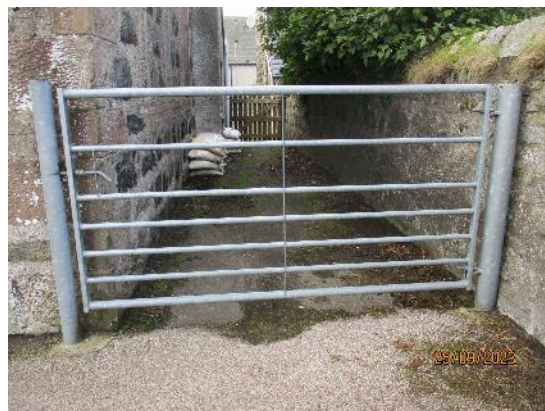
219. Galvanised rail gate
