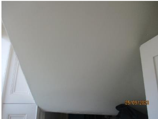
94. Lath & plaster soffit
