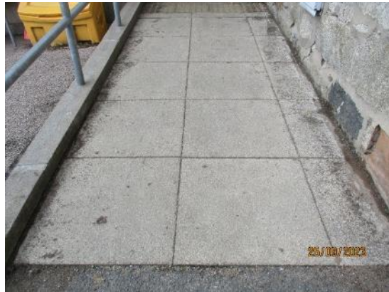
76. Paving slab ramps
