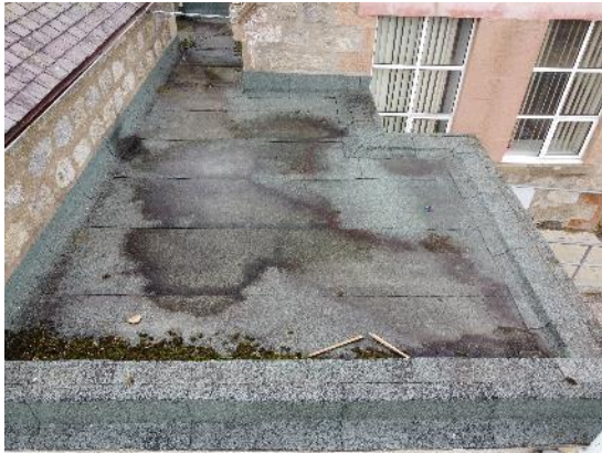
7. Felt roof above Boy's toilets
