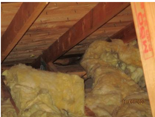
17. Disturbed insulation
