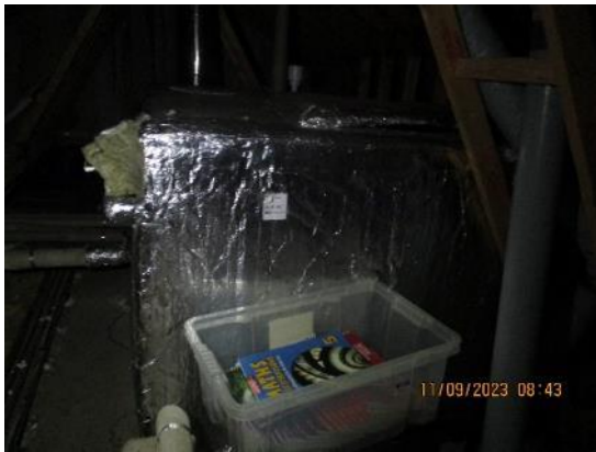
124. Cold water tank in attic space.
