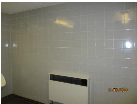
79. Ceramic wall tiles full height
