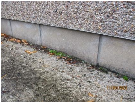
31. Dressed blockwork underbuilding
