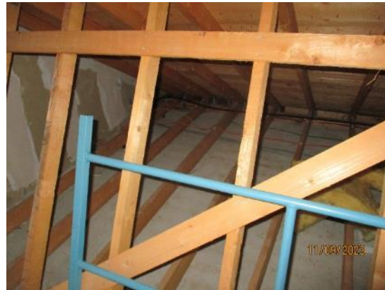
16. Missing insulation
