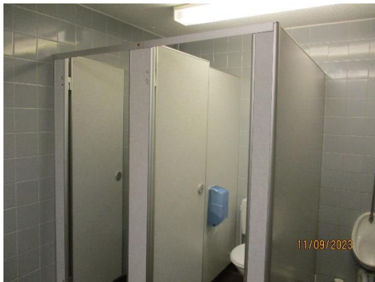
95. Composite panel cubicles
