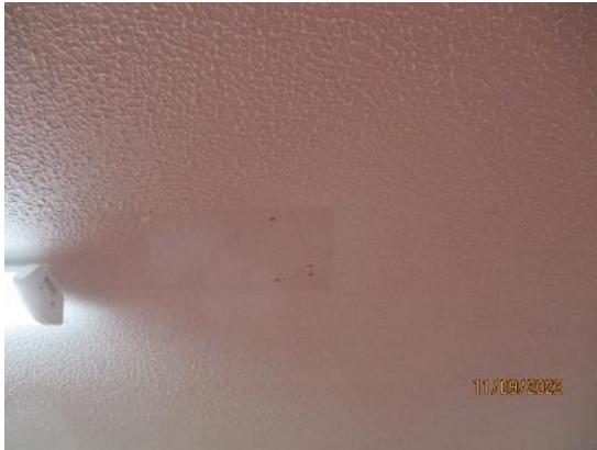
69. Textured finish to plasterboard ceilings
