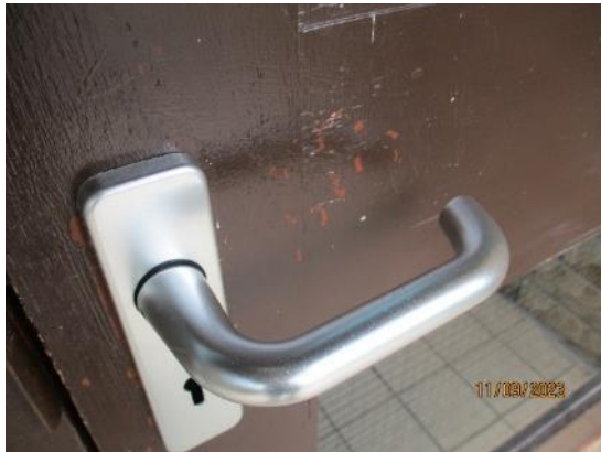
50. Timber external doors
