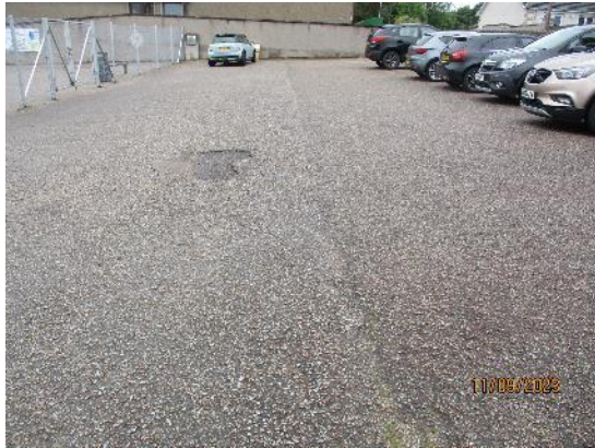
154. Tarmacadam car park
