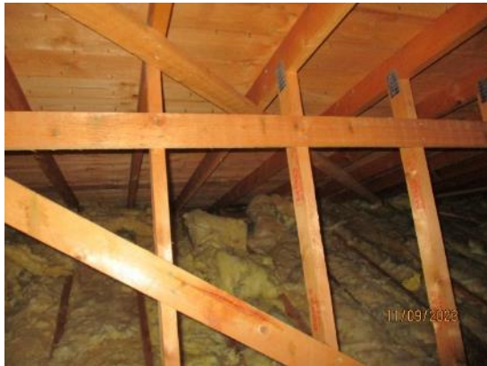
15. Mineral fibre insulation laid over ceilings
