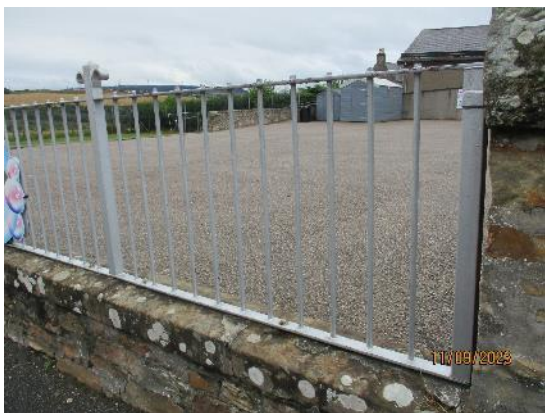
176. Metal bar railings above stone walls
