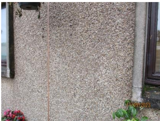
29. Roughcast finish to external walls
