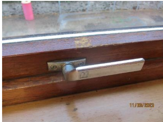
46. Lever handles to timber windows
