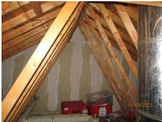
1. Timber trusses to all roofs
