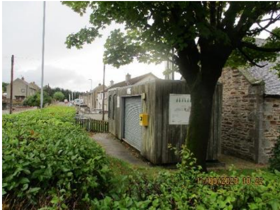
118. Biomass plant room. District heating source.
