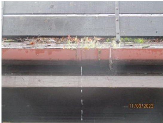
19. Blocked/leaking gutters
