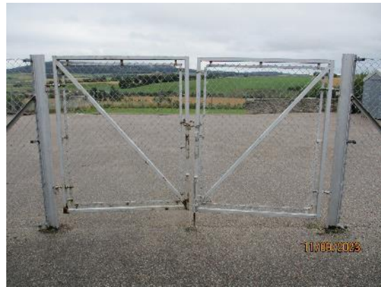
179. Metal framed chain link gates
