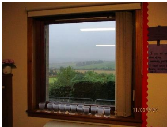
42. Internal view of timber windows
