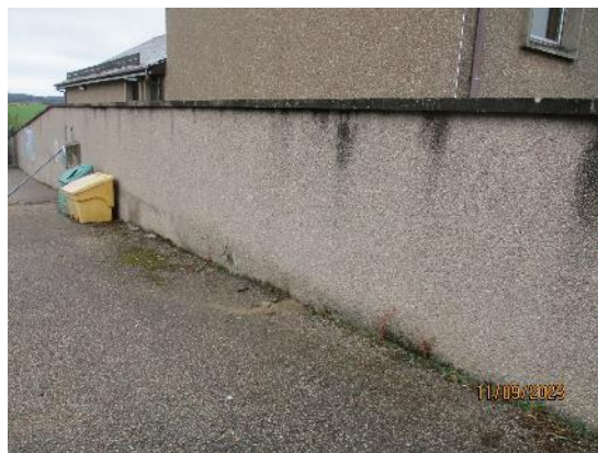
189. Retaining wall with roughcast surface
