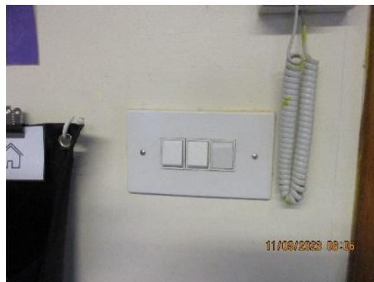
135. Flush fitted wiring accessories – light switch typical.
