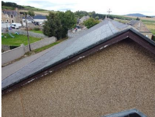
48. Roof joinery items
