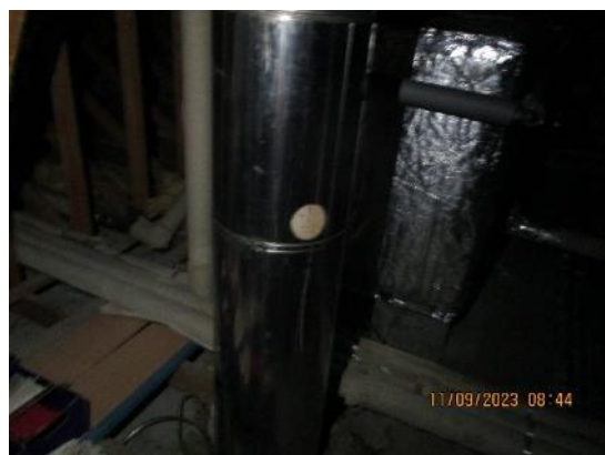
152. Boilers flue rising through attic space.
