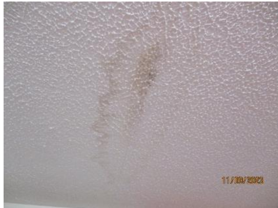
72. Watermarked plasterboard
