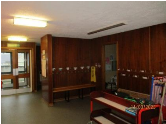
77. Timber plywood linings full height
