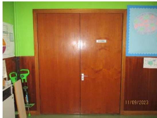
84. Timber solid core double doors
