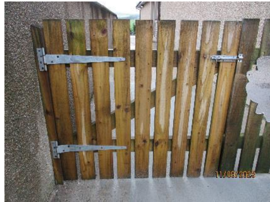
181. Timber boarded gates to both sides
