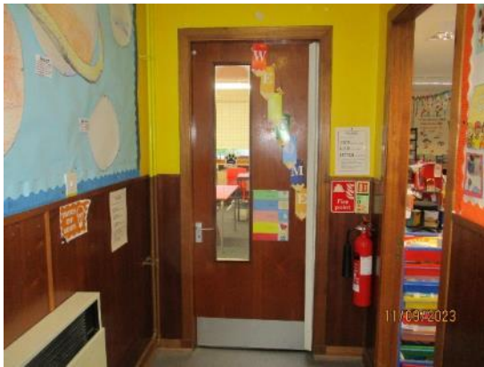
81. Solid core timber doors with vision panels
