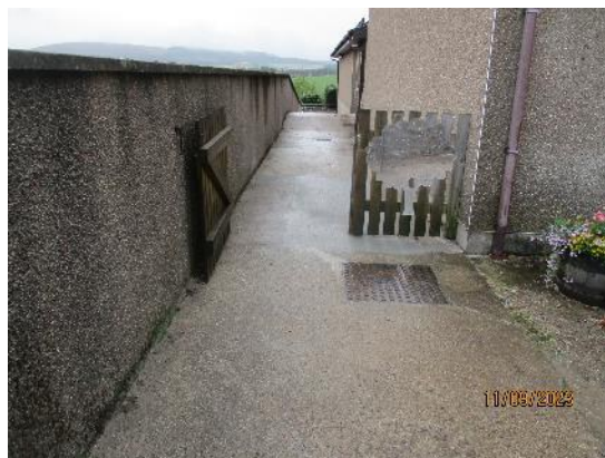
159. In-situ concrete footpaths
