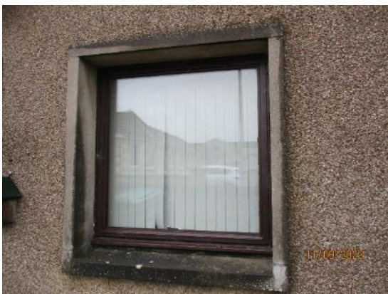
41. Timber windows to most elevations
