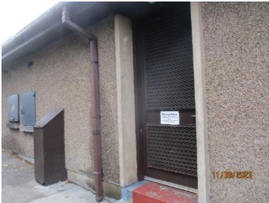
39. Timber door to Boiler Room
