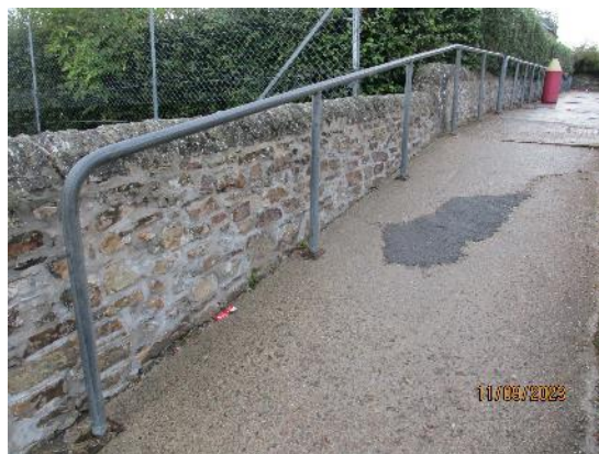
177. Galvanised rail to boundary wall
