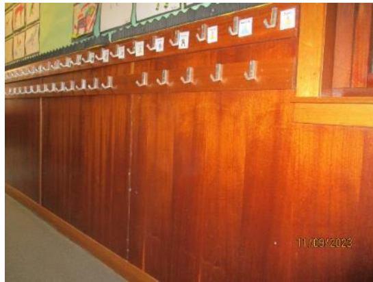
76. Timber plywood linings to half height
