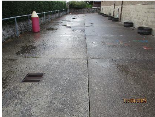
161. In-situ concrete playground
