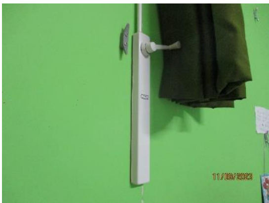
47. Winding handles to aluminium windows
