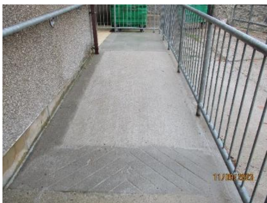
54. Concrete ramp to entrance
