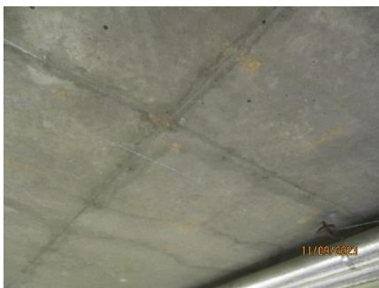
74. Concrete ceiling to Boiler Room
