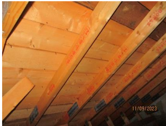
2. Timber sarking boards
