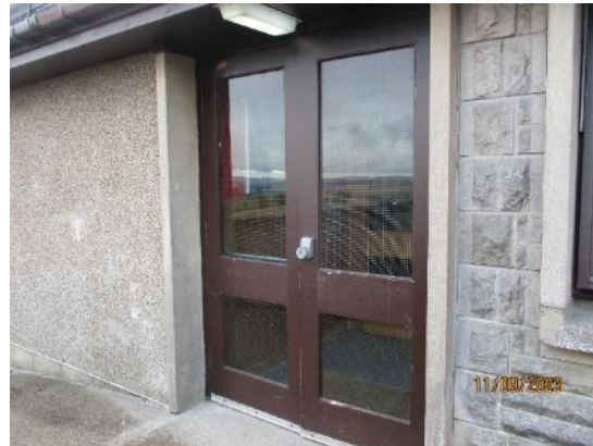
40. Double timber doors
