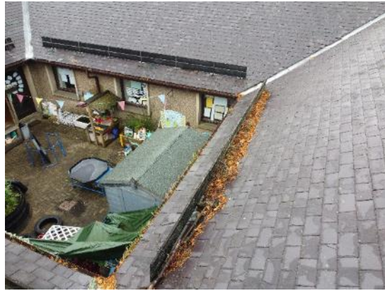
26. Leaf fall and debris trapped by snow boards
