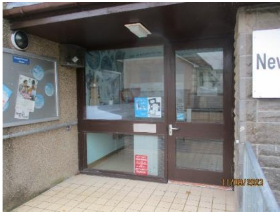
37. Timber entrance screen
