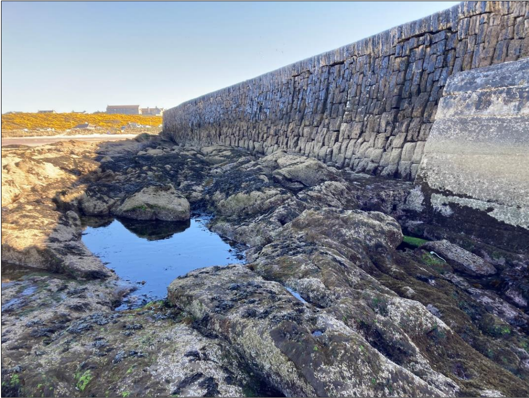
Photo 31: Outer Face of East Pier
