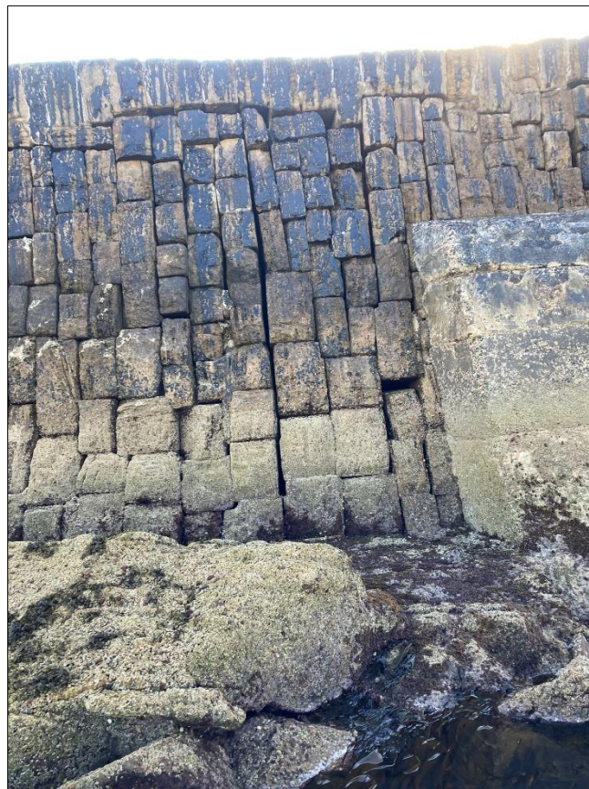
Photo 32: Outer face of East Pier.
