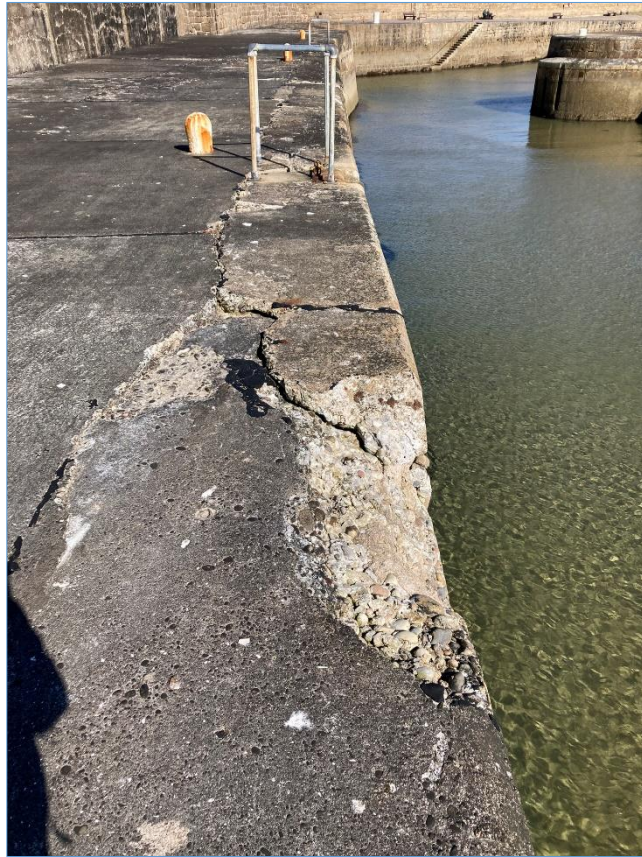
Photo 9: North Pier Cope.
