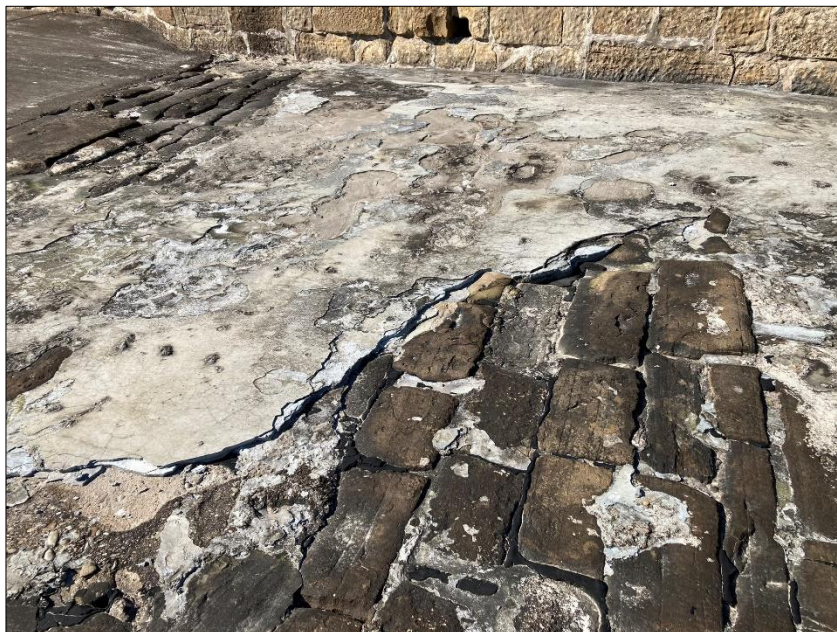
Photo 12: North Pier deck.
