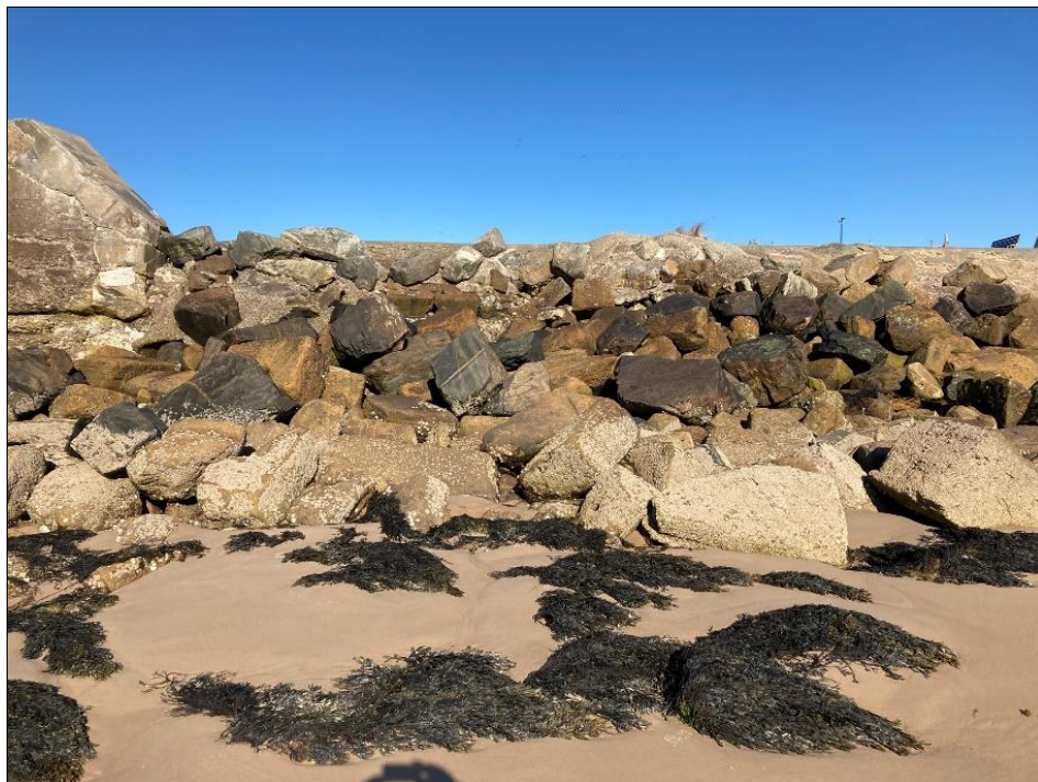
Photo 28: Rock armour south end of West Pier.
