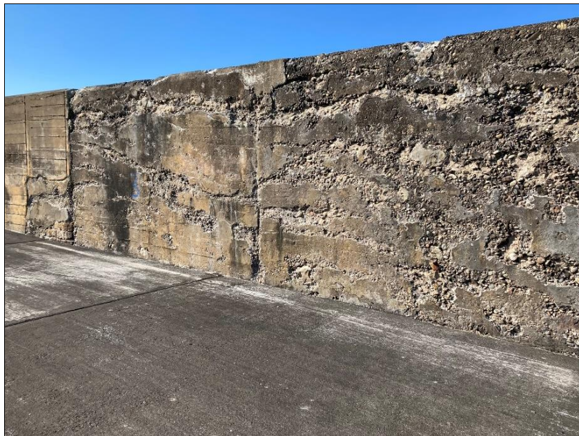
Photo 10: North Pier Parapet Wall.
