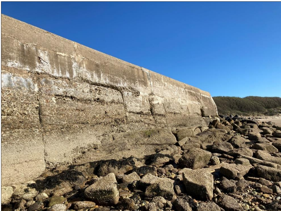
Photo 30: Parapet Wall south end of West Pier.
