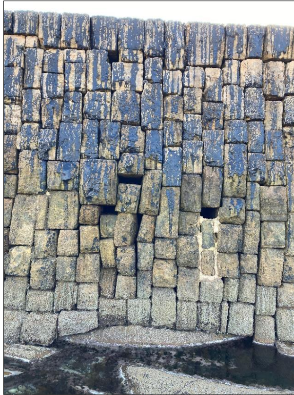
Photo 33 : Outer face of East Pier
