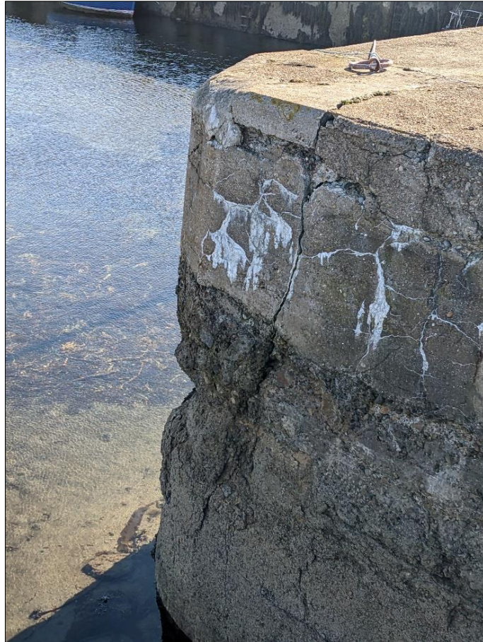
Photo 27: South Pier west corner inner basin.
