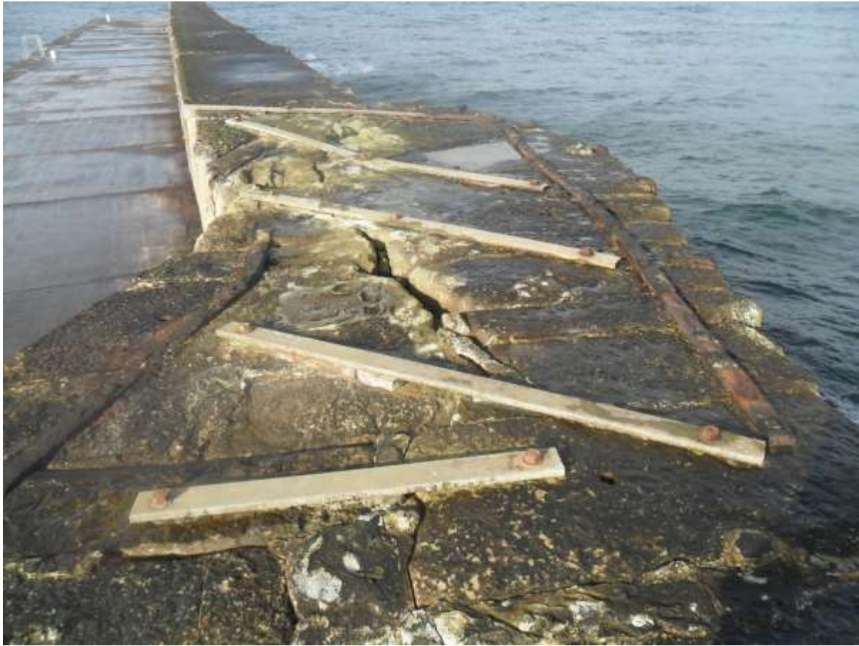
Reinforcement Bars on Masonry Parapet
