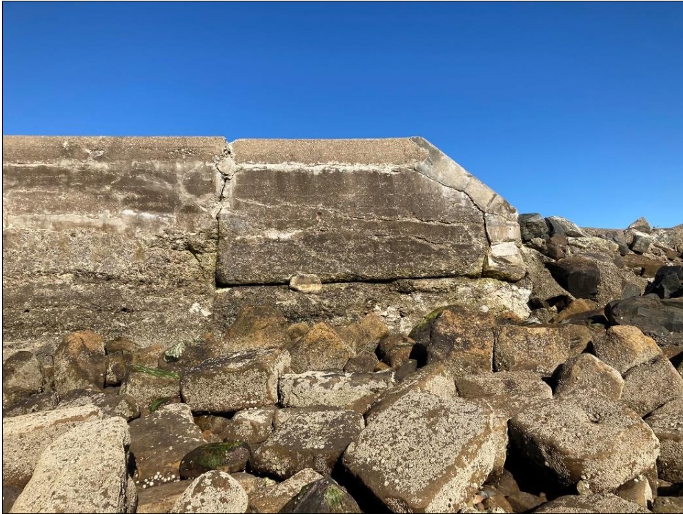
Photo 29: Parapet wall south end of West Pier.
