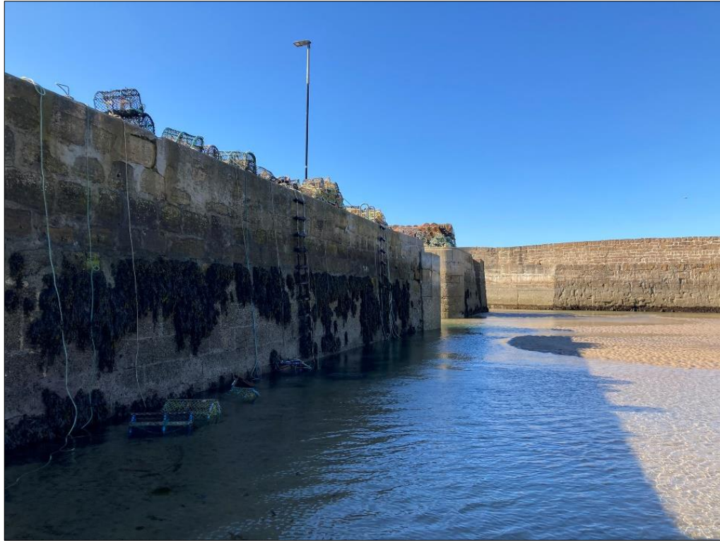
Photo 21 : Central Pier quay wall face outer basin.
