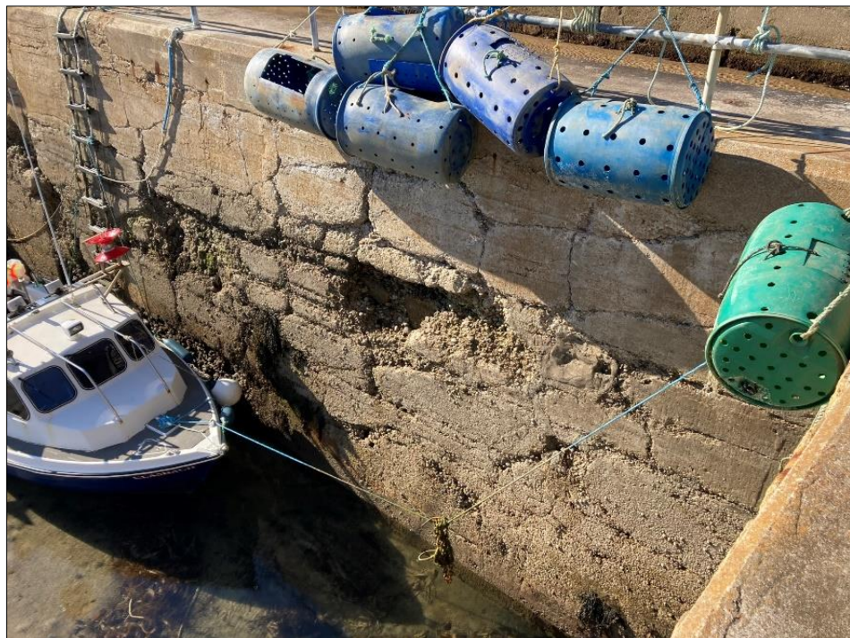
Photo 24: South Pier quay wall inner basin face.
