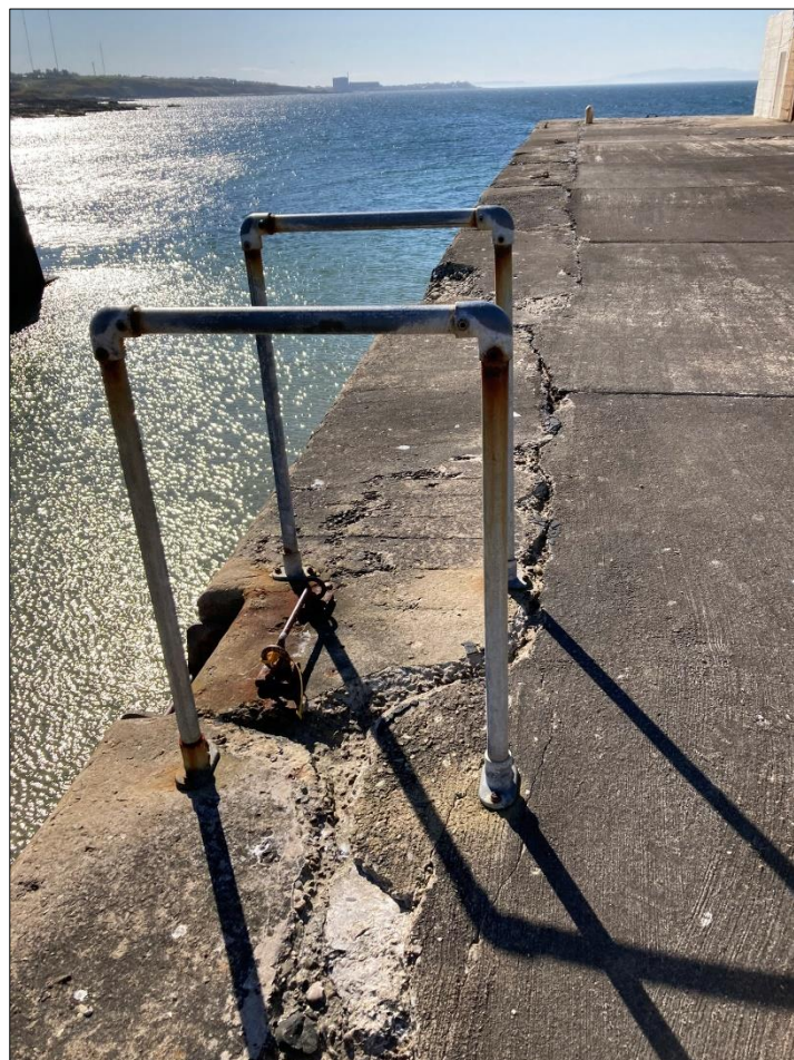
Photo 8: North Pier cope.
