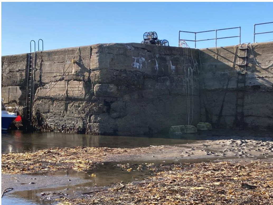
Photo 26: South Pier west corner inner basin.
