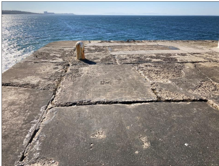
Photo 7: North pier deck.
