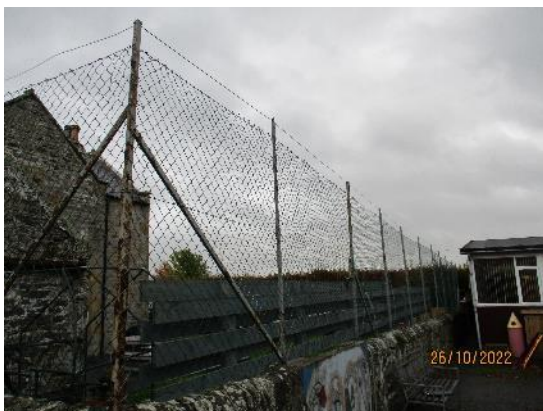
145. Chainlink above walls
