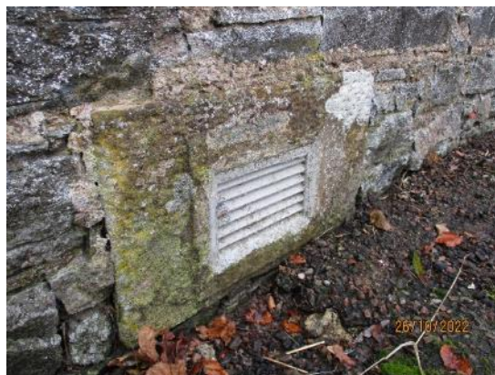
30. Ground level – Old building
