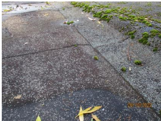
9. Felt has exceeded useful life
