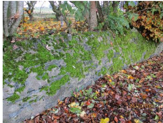
150. Natural stone walls
