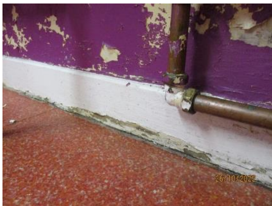
92. Skirtings and walls
