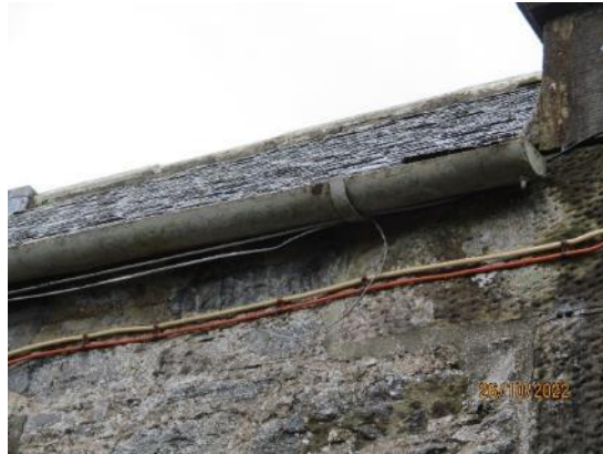
20. Cast iron gutters to old building
