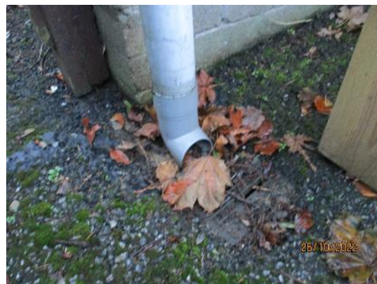
152. Surface water drainage gully
