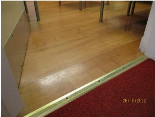
66. Laminate flooring – Staff room
