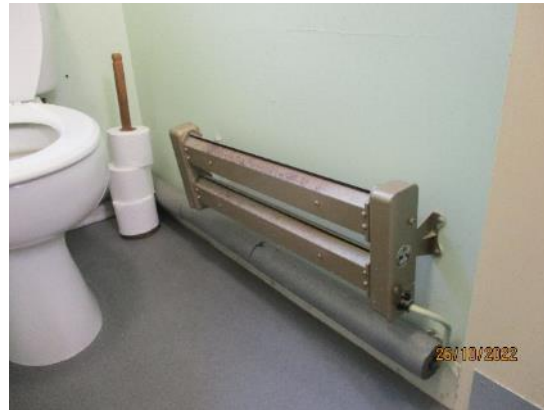
102. Electric tube heater – class block
