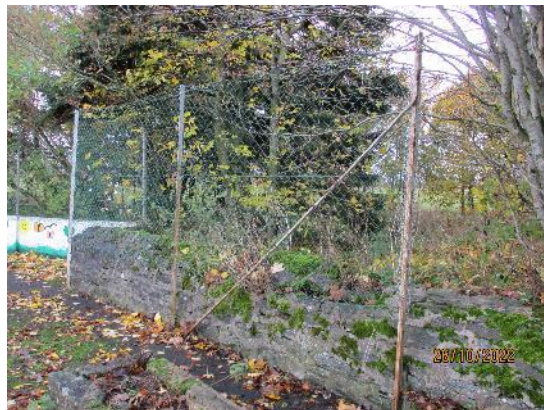
144. High chainlink fencing
