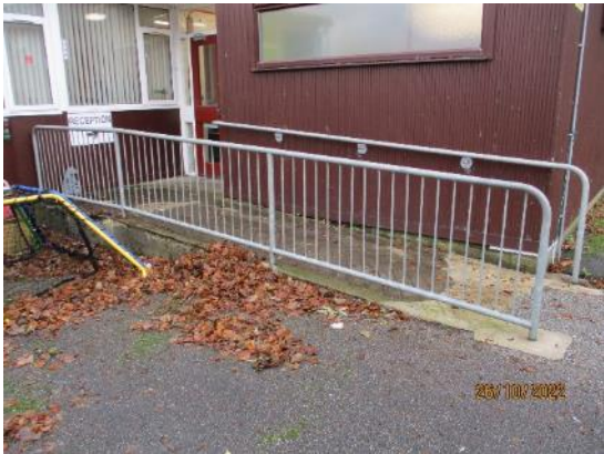
57. Galvanised handrail to ramp
