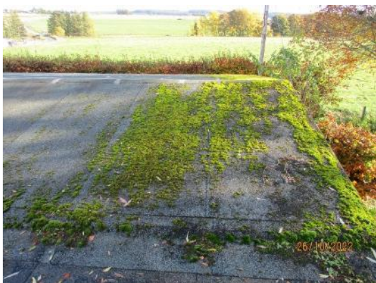
11. Surface moss to pitched felt roof
