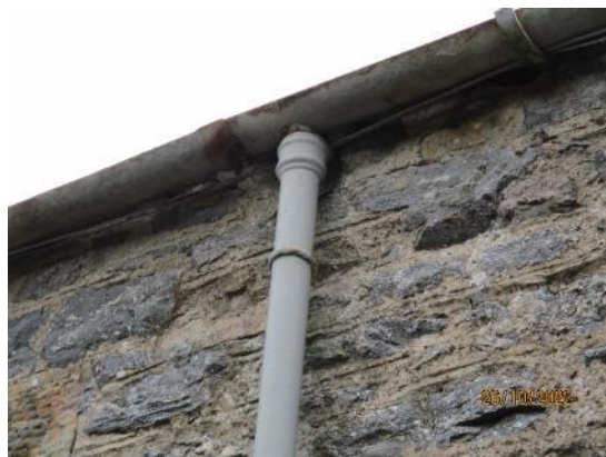
24. Cast iron rainwater downpipes
