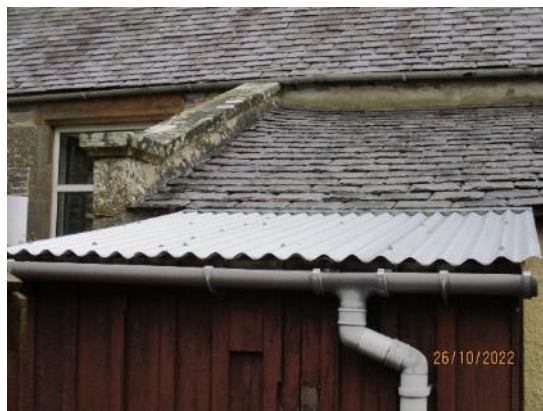
6. Metal profile lean-to roof
