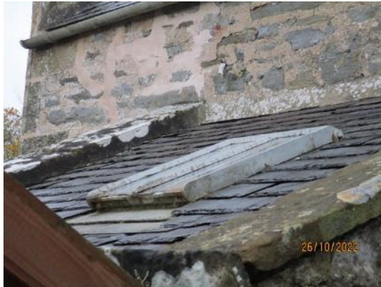
13. Metal skylight to old building
