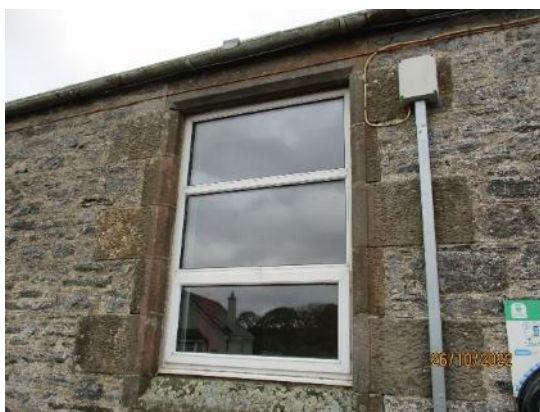
44. UPVC windows – old block
