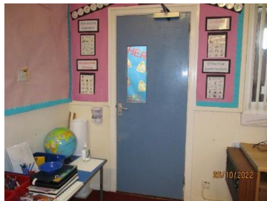
87. Timber doors – Teaching block
