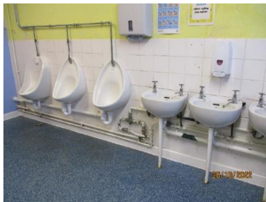
81. Ceramic wall tiles – Boys toilet
