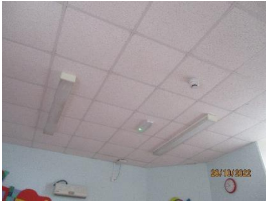
123. Lighting – old building dining room
