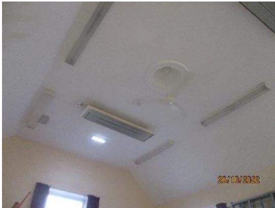
101. Electric radiant panel heater assembly roof
