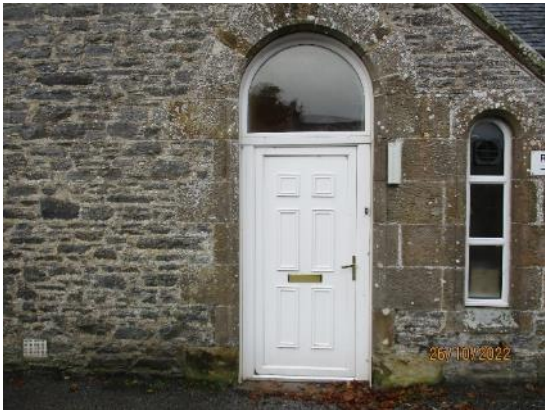
39. UPVC door to old building
