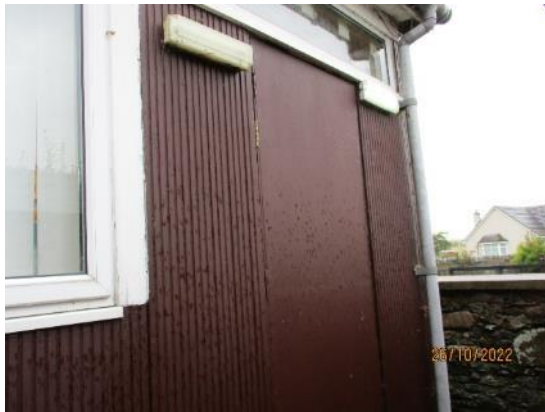
37. Timber fire escape doors
