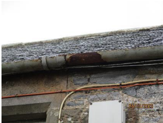
21. Surface corrosion
