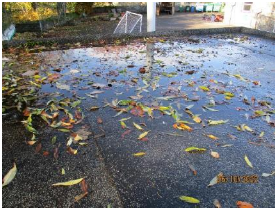
7. Felt roof to teaching block
