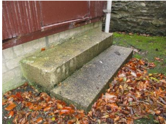
56. Concrete steps to fire exits
