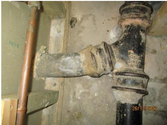
89. Lead waste pipes
