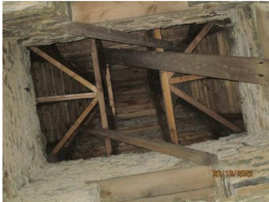
1. Bell tower roof structure
