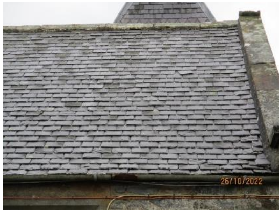
3. Slate to old building
