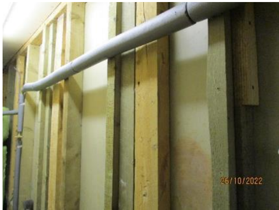
76. Timber framed walls – Teaching block
